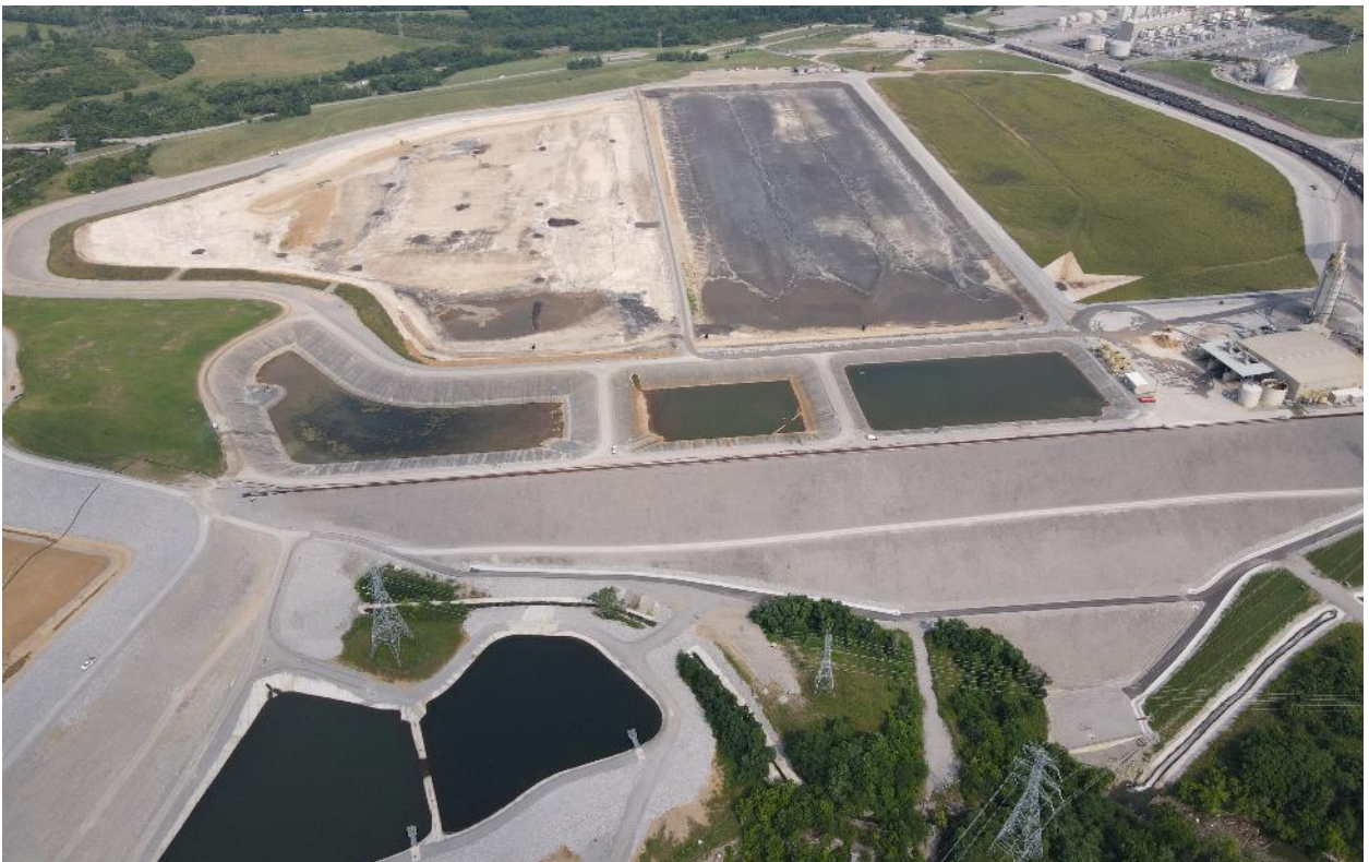
E.W. Brown Landfill Phase II and Closure – June 2021
