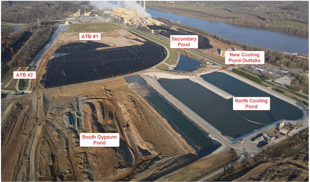
Ghent ATB #1 – Looking West – March 2021
