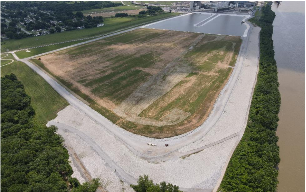
Mill Creek Main Ash Pond Closure – July 2021
