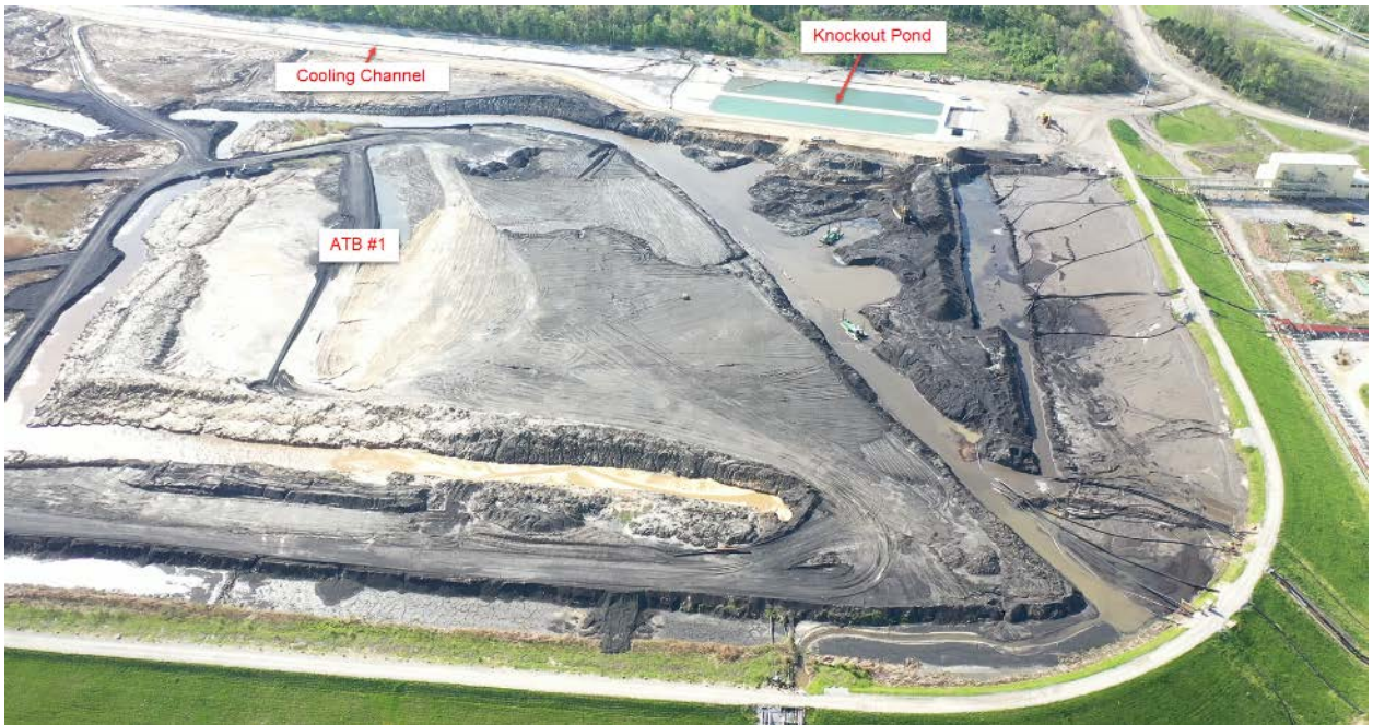
Ghent ATB #1 Cooling Channel – Looking North – April 2019
