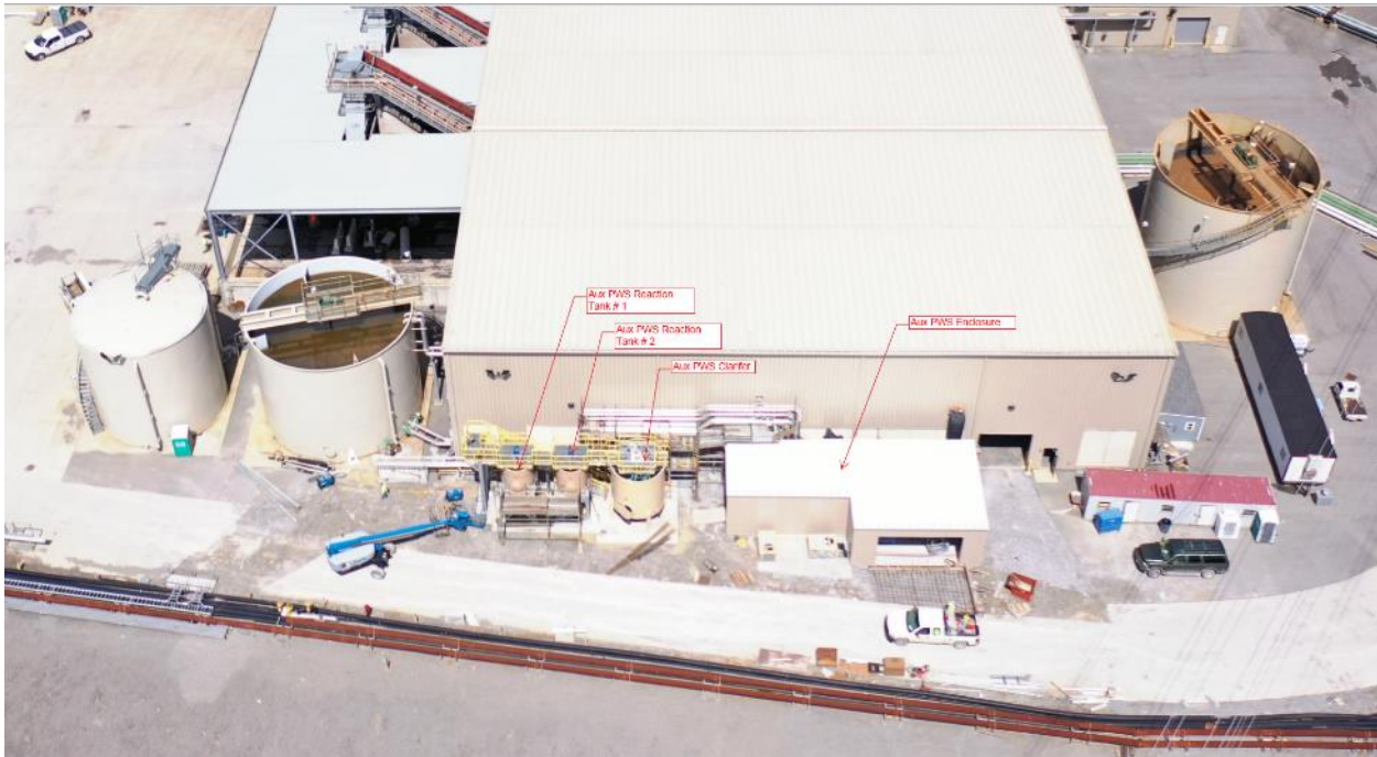
E. W. Brown PWS Treatment System – June 2019
