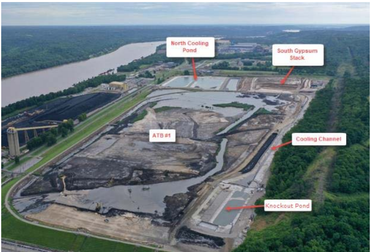
Ghent ATB #1 Cooling Channel – Looking West – June 2019
