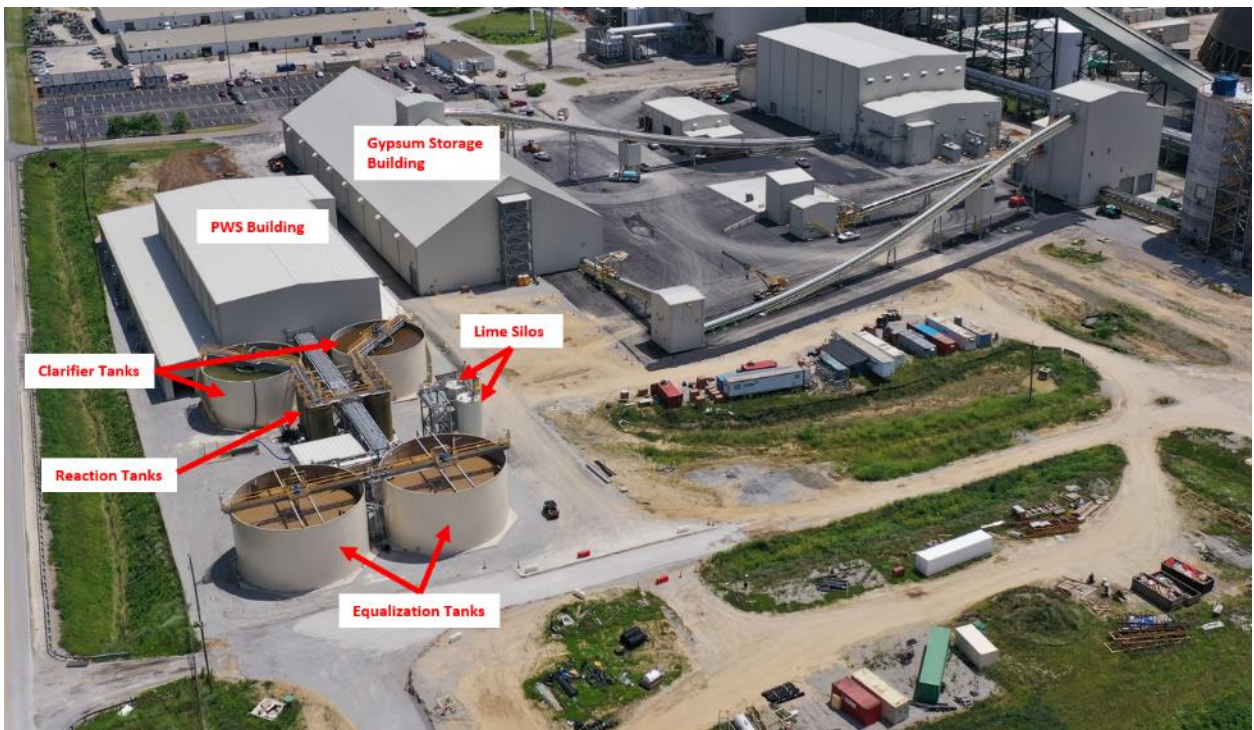
Trimble County PWS Facility – Site View Looking Southwest – June 2019
