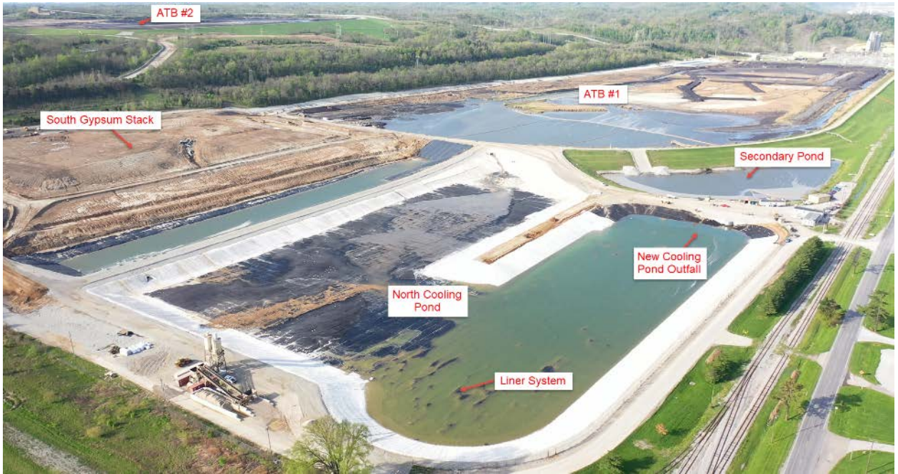
Ghent Gypsum Stack – Looking South – April 2019
