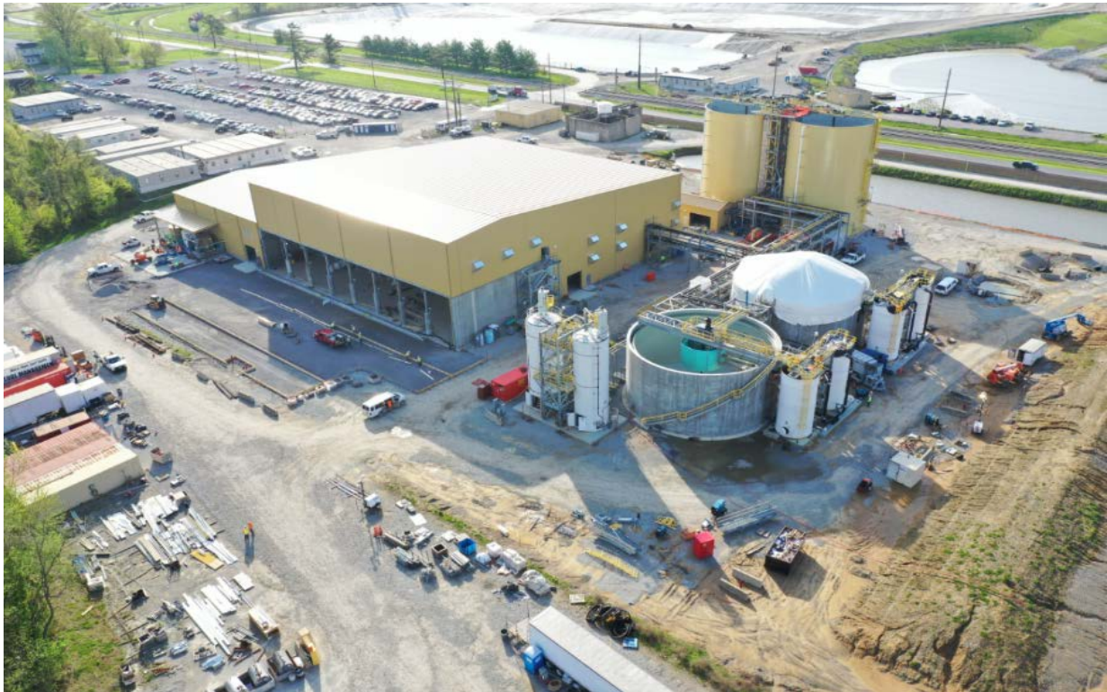
Ghent PWS Facility – Site View – April 2019
