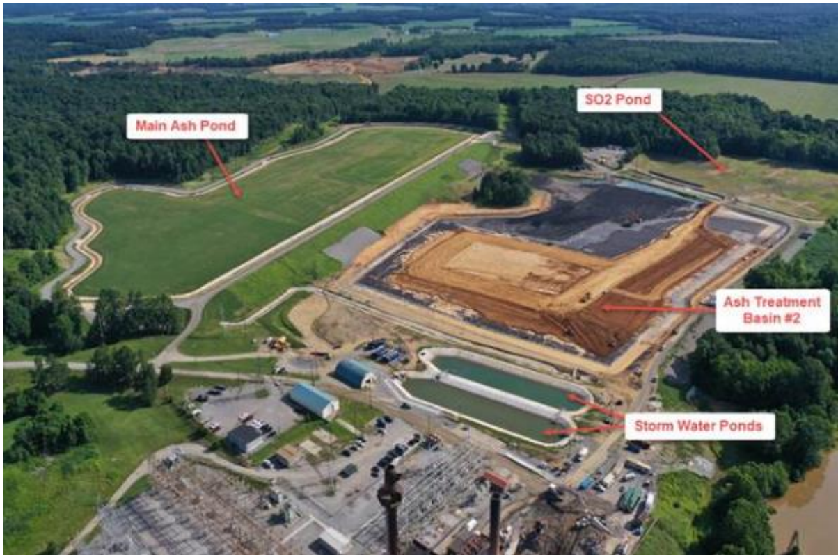
Green River CCR Impoundments – Site View – June 2019
