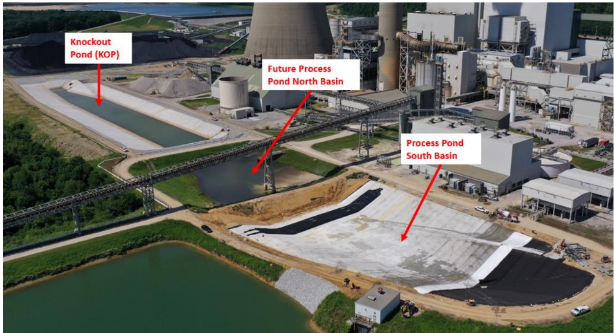
Trimble County Process Water Ponds – Looking Northeast – June 2019
