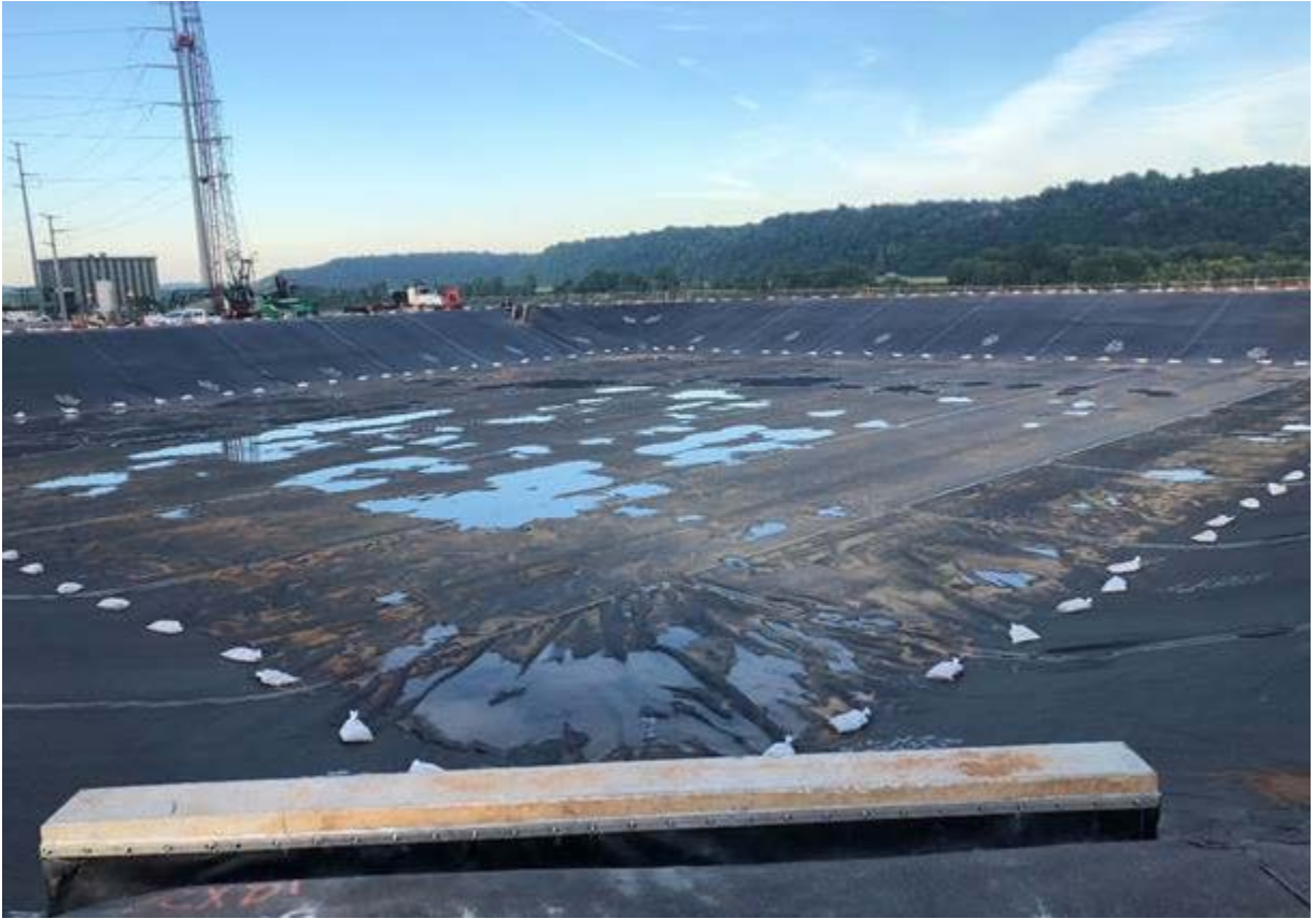
Mill Creek Knock-Out Pond
