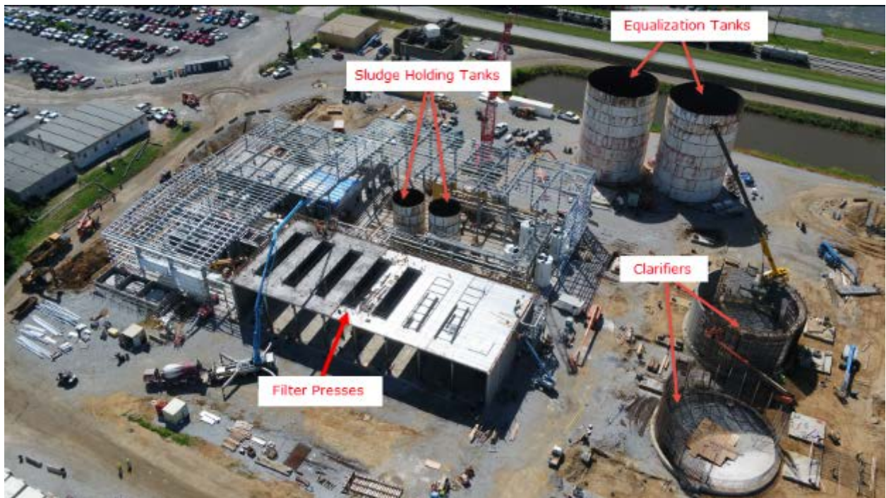
Ghent PWS Facility – Site View
