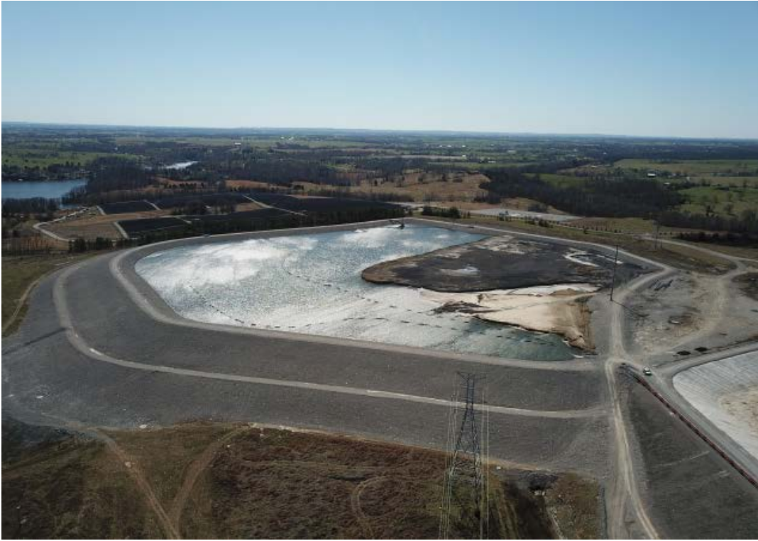
E.W. Brown Aux Pond – Pre-Construction
