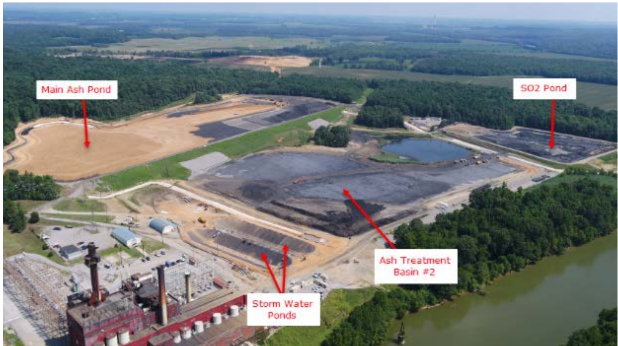
Green River CCR Impoundments – Site View
