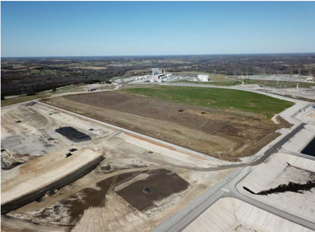
E.W. Brown Landfill Phase II and Closure – Pre-Construction
