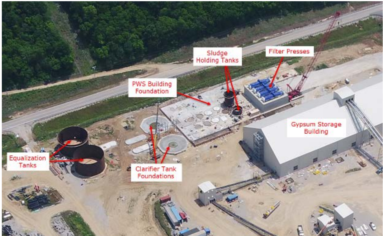
Trimble County PWS Facility – Site View
