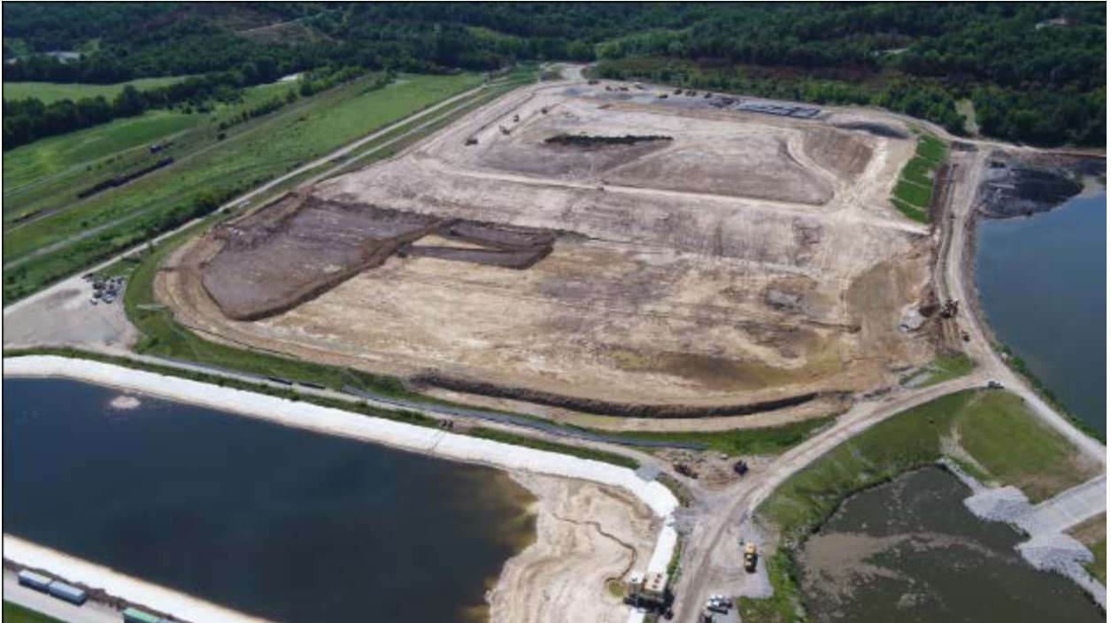
Ghent Gypsum Stack – Looking South
