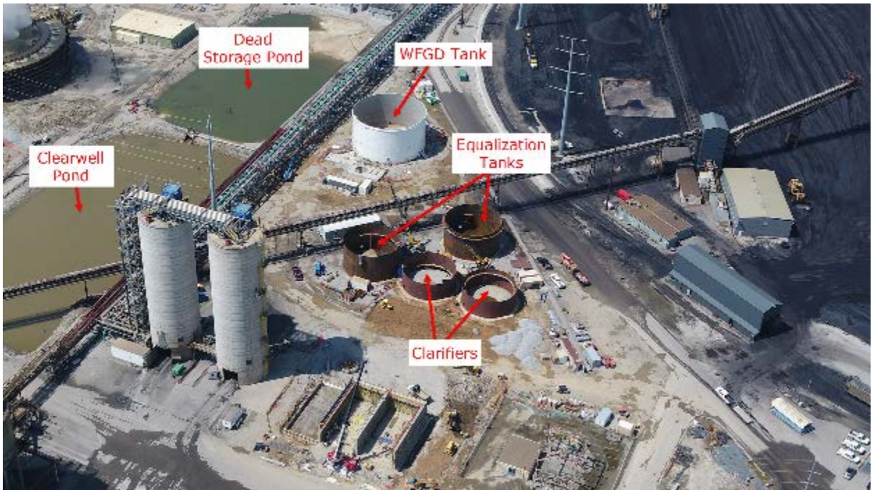
Mill Creek PWS Facility – Site View
