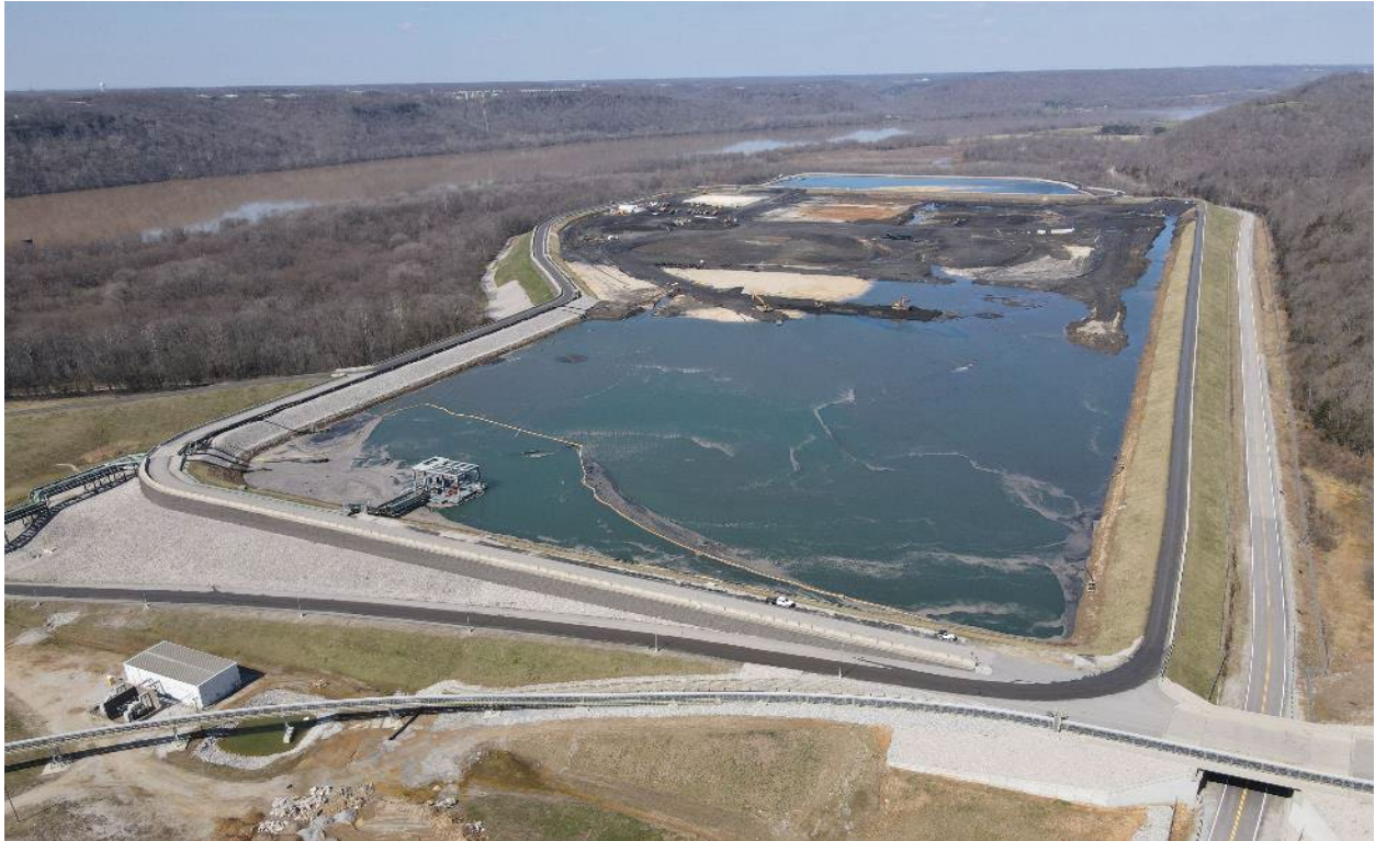
Trimble BAP – Looking North – April 2022
