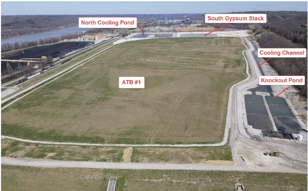
Ghent ATB #1 and Cooling Channel – Looking East – April 2022
