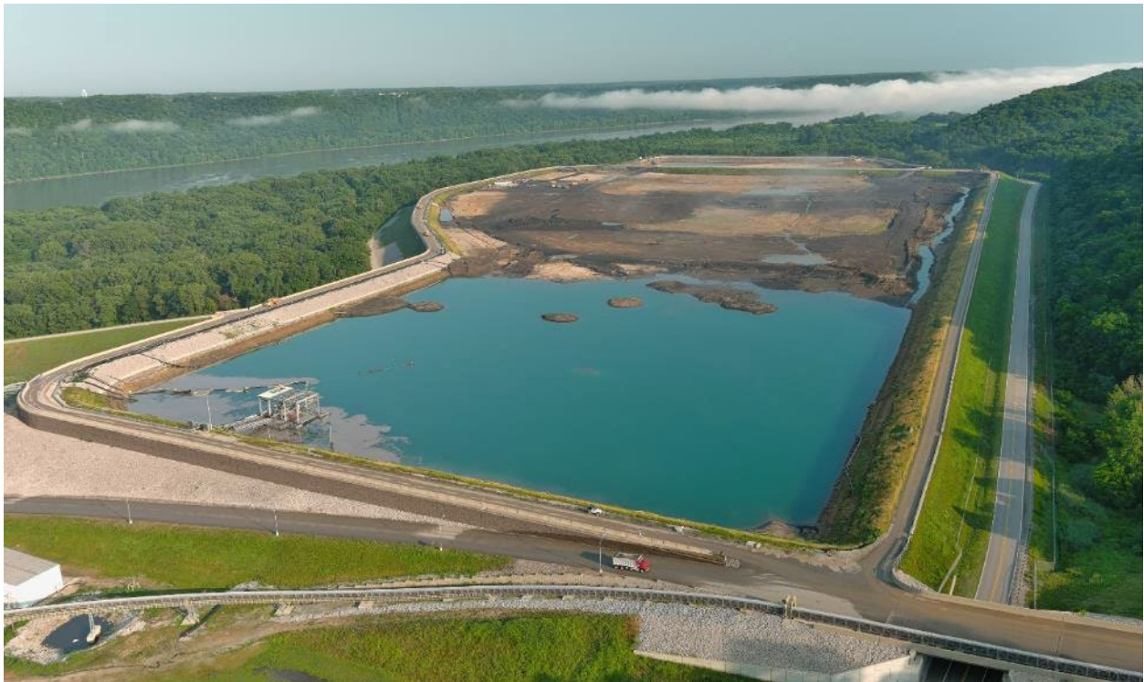
Trimble BAP – Looking North – July 2022
