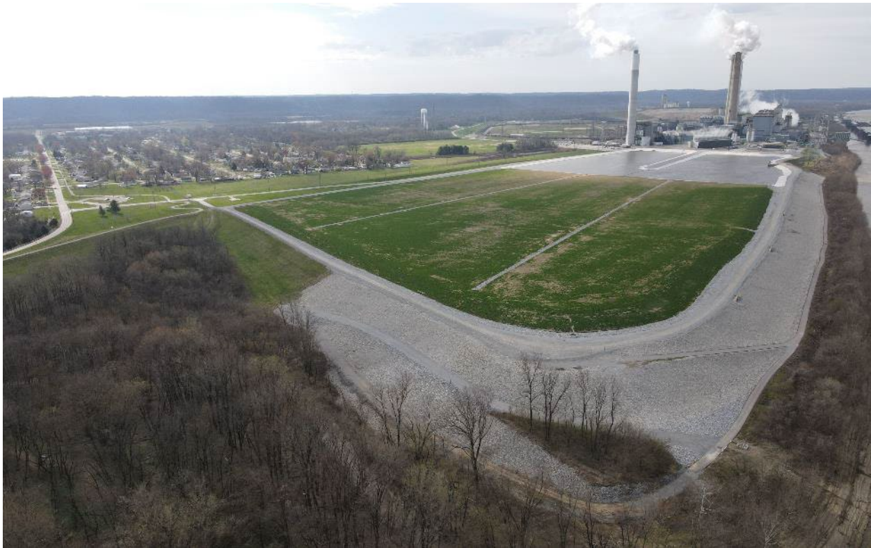
Mill Creek Main Ash Pond Closure – March 2022 – No Change July 2022
