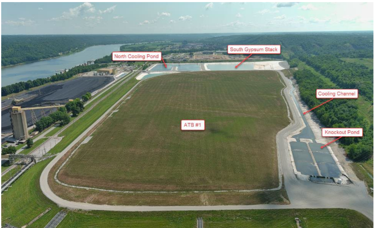
Ghent ATB #1 and Cooling Channel – Looking East – July 2022
