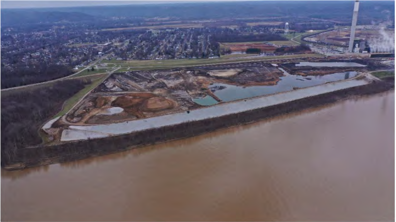
Mill Creek Main Ash Pond Closure – December 2019
