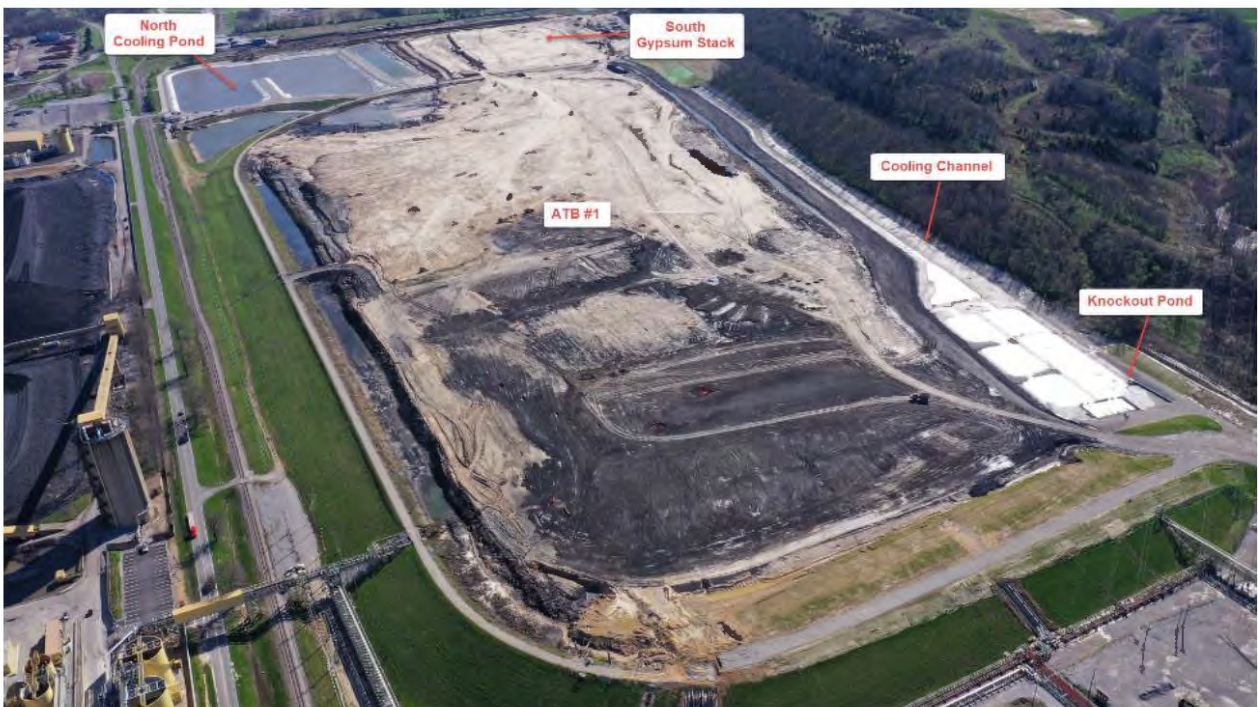
Ghent ATB #1 Cooling Channel – Looking East – March 2020
