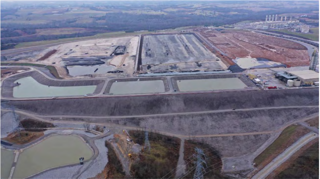
E.W. Brown Landfill Phase II and Closure – December 2019
