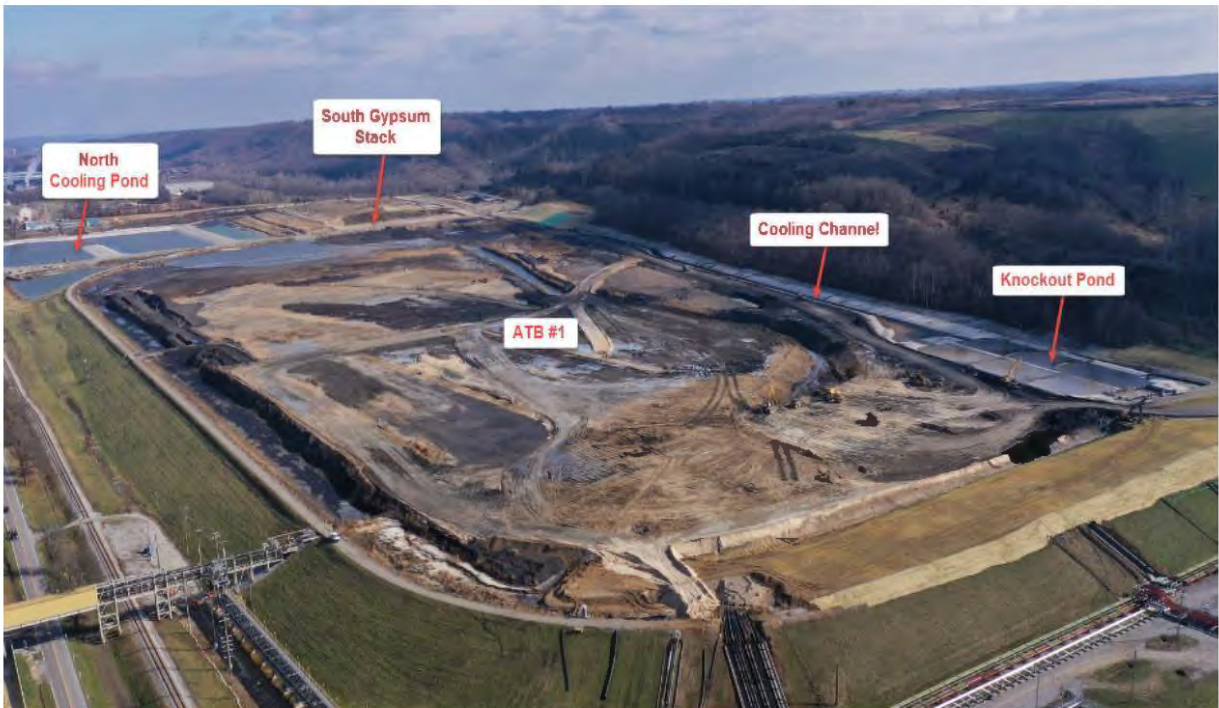
Ghent ATB #1 Cooling Channel – Looking East – December 2019
