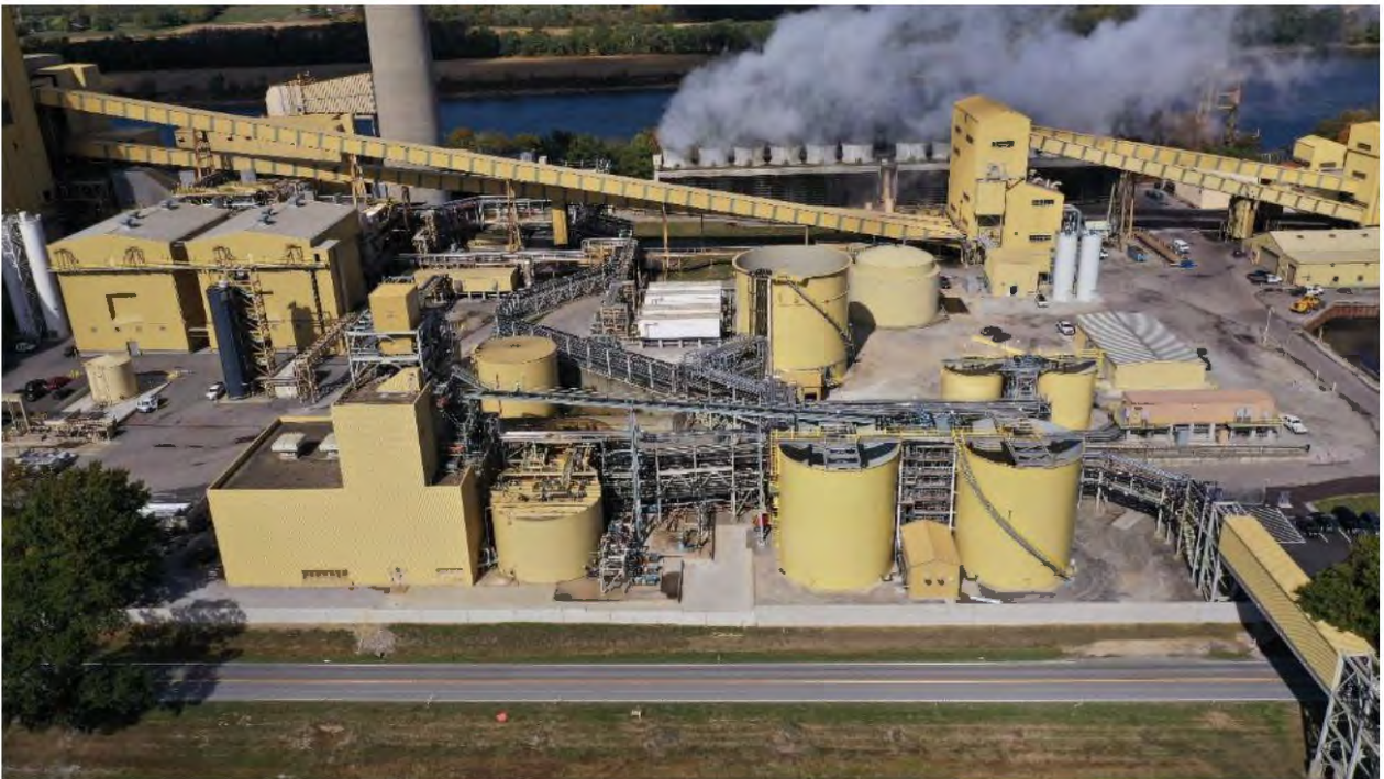
Ghent PWS Tank Farm – Site View – October 2019 – No Change in March 2020
