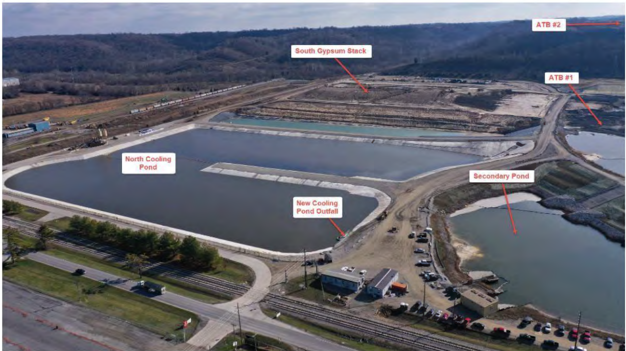
Ghent Gypsum Stack – Looking East – December 2019
