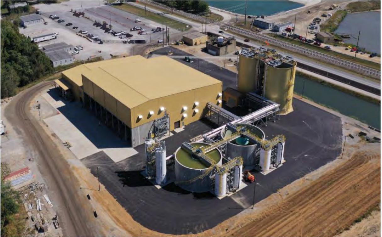
Ghent PWS Facility – Site View – October 2019 – No Change in March 2020
