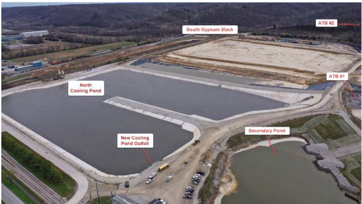
Ghent Gypsum Stack – Looking East – March 2020
