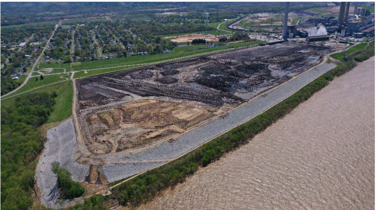
Mill Creek Main Ash Pond Closure – March 2020
