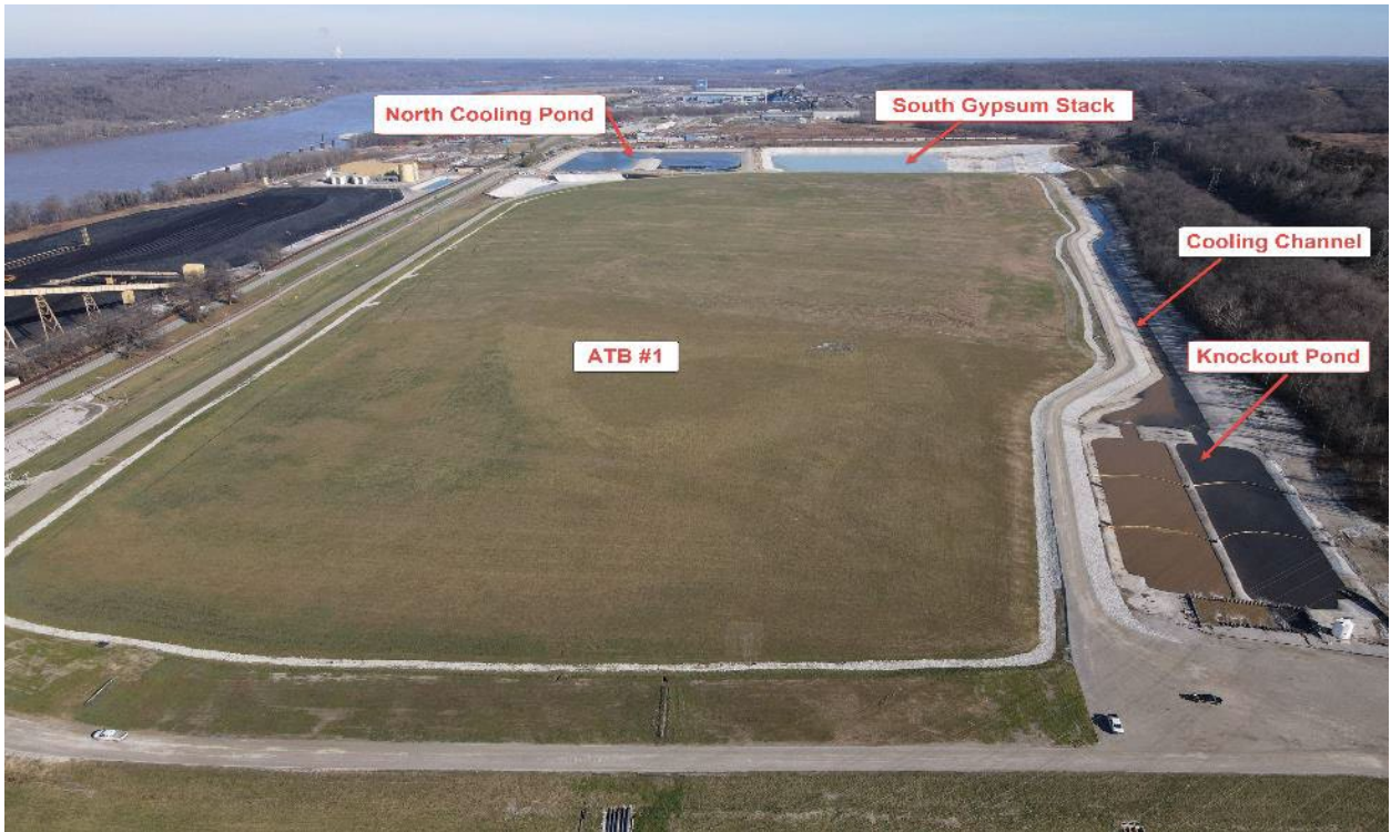
Ghent ATB #1 and Cooling Channel – Looking East – January 2022
