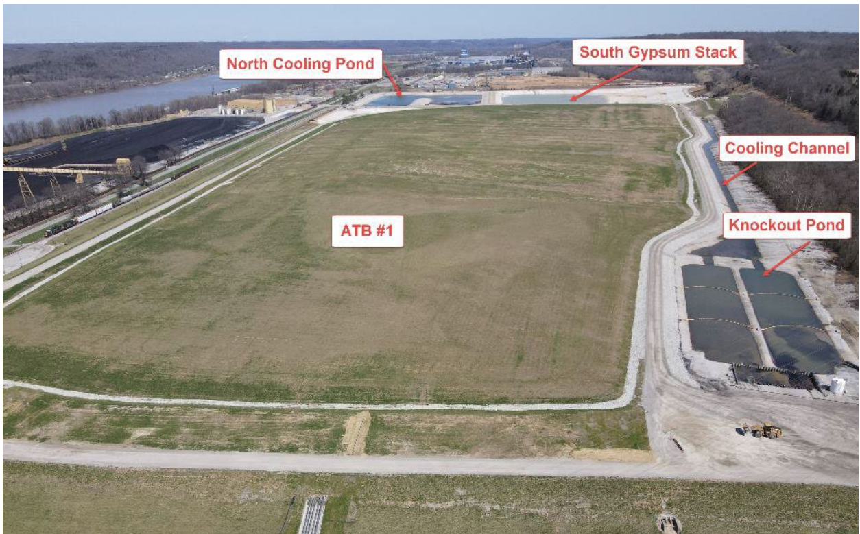
Ghent ATB #1 and Cooling Channel – Looking East – April 2022
