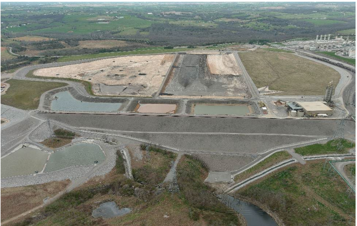
E.W. Brown Landfill Phase II and Closure – March 2022
