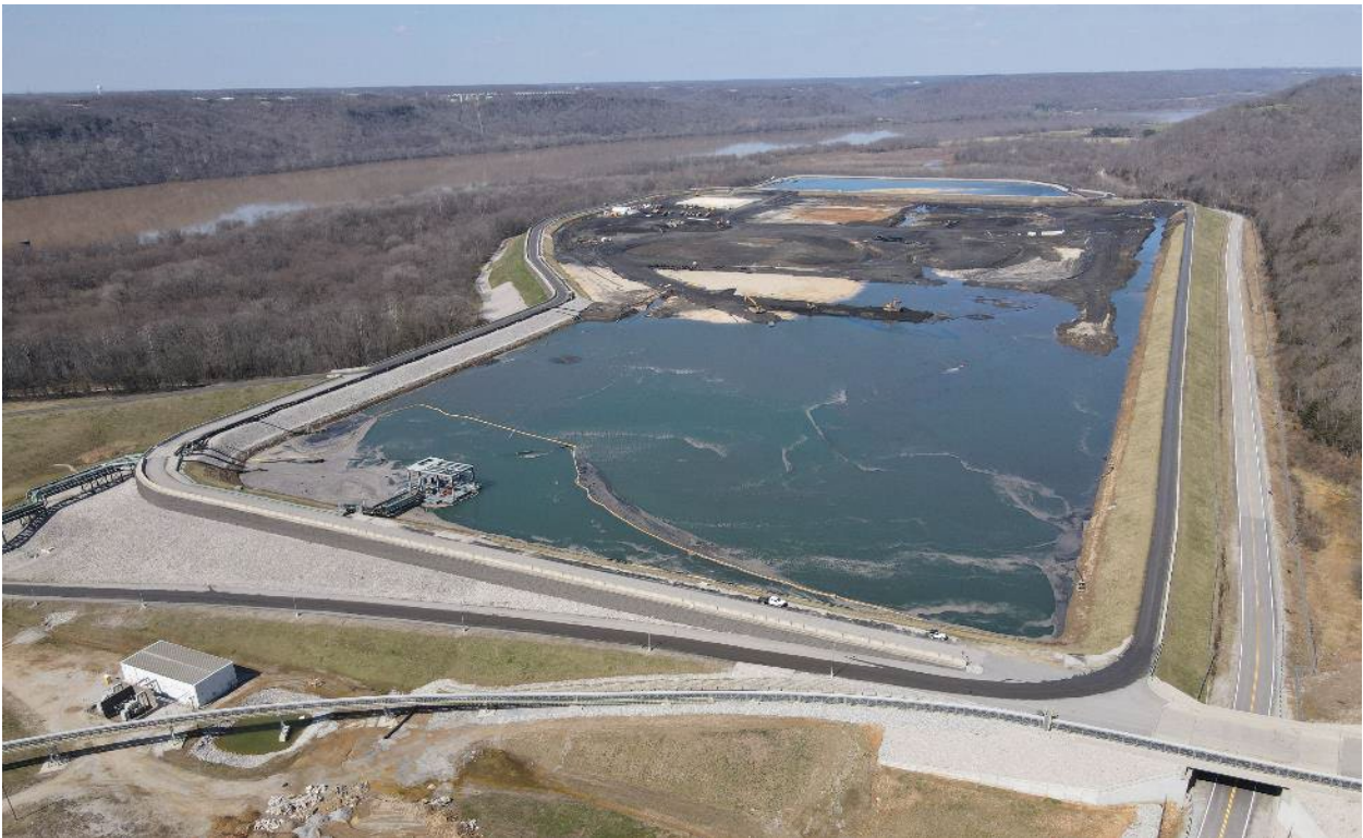
Trimble BAP – Looking North – April 2022
