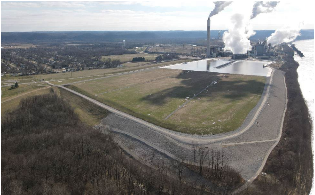
Mill Creek Main Ash Pond Closure – January 2022
