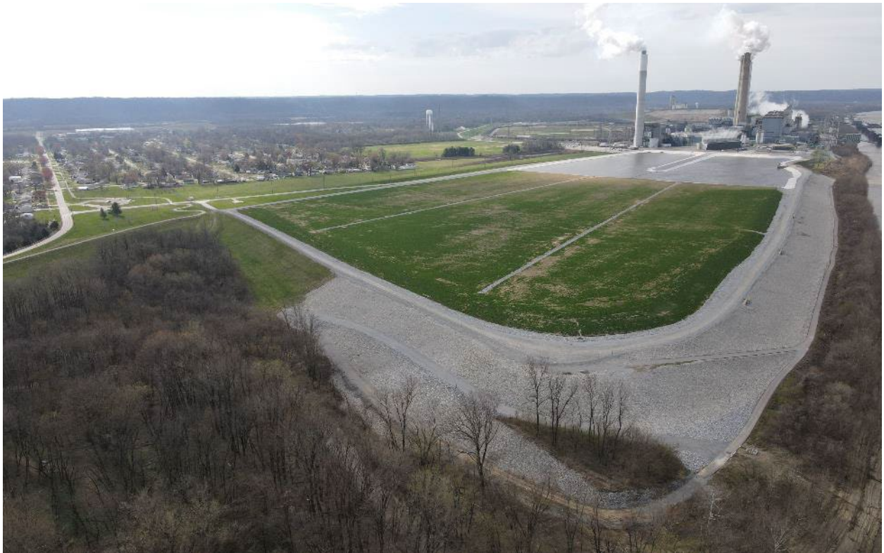
Mill Creek Main Ash Pond Closure – March 2022
