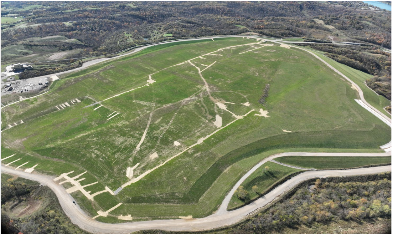
Phase III Ghent ATB #2 – December 2024
