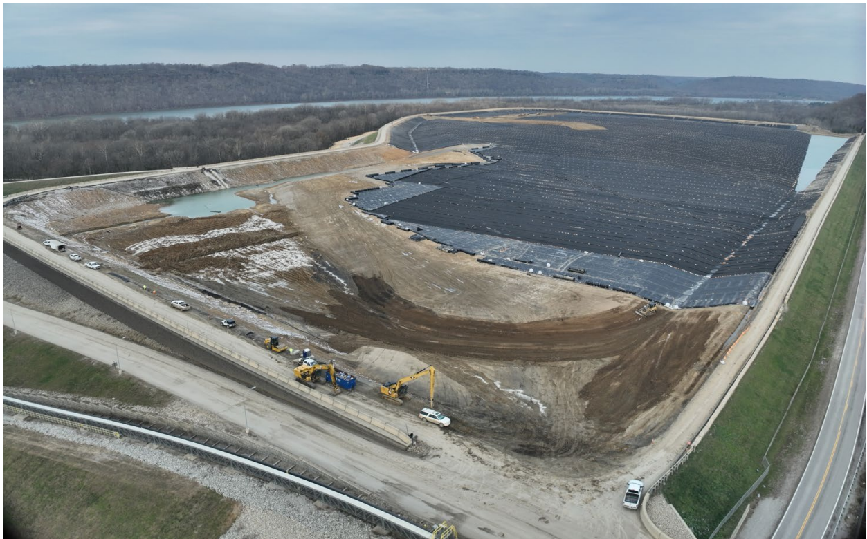
Trimble BAP – Looking Northeast – December 2024
