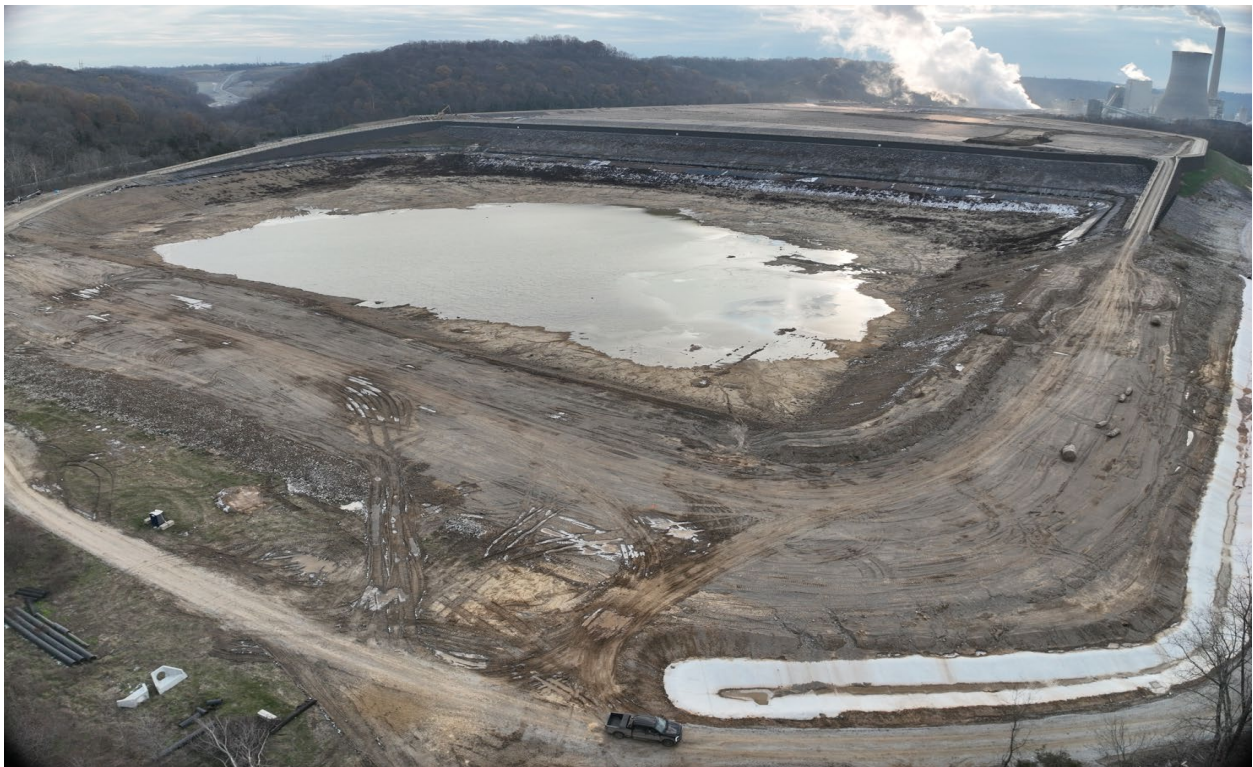
Trimble GSP – Looking South – December 2024
