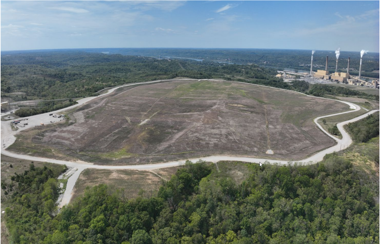
Phase III Ghent ATB #2 – September 2024
