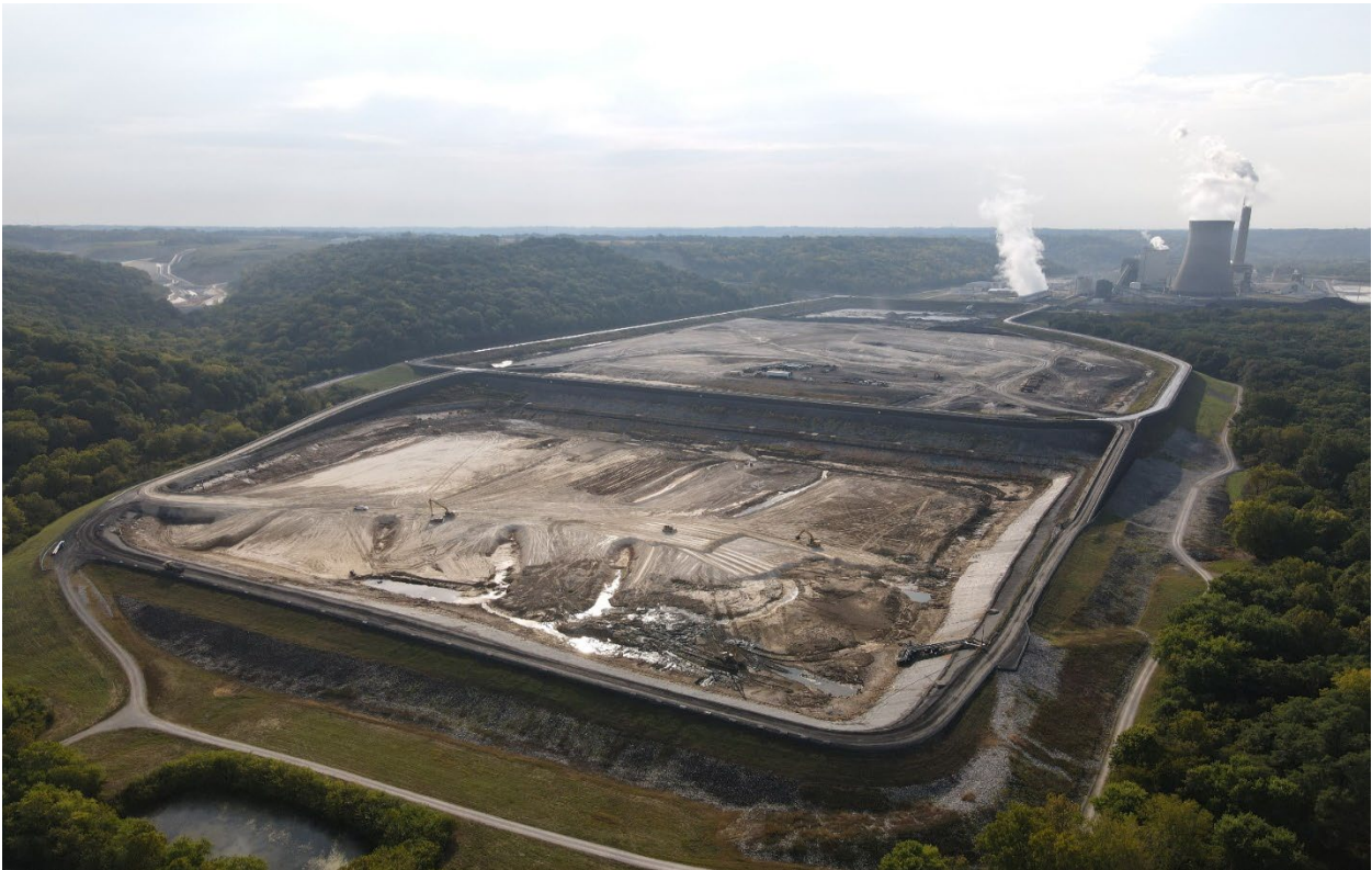
Trimble GSP – Looking South – September 2023
