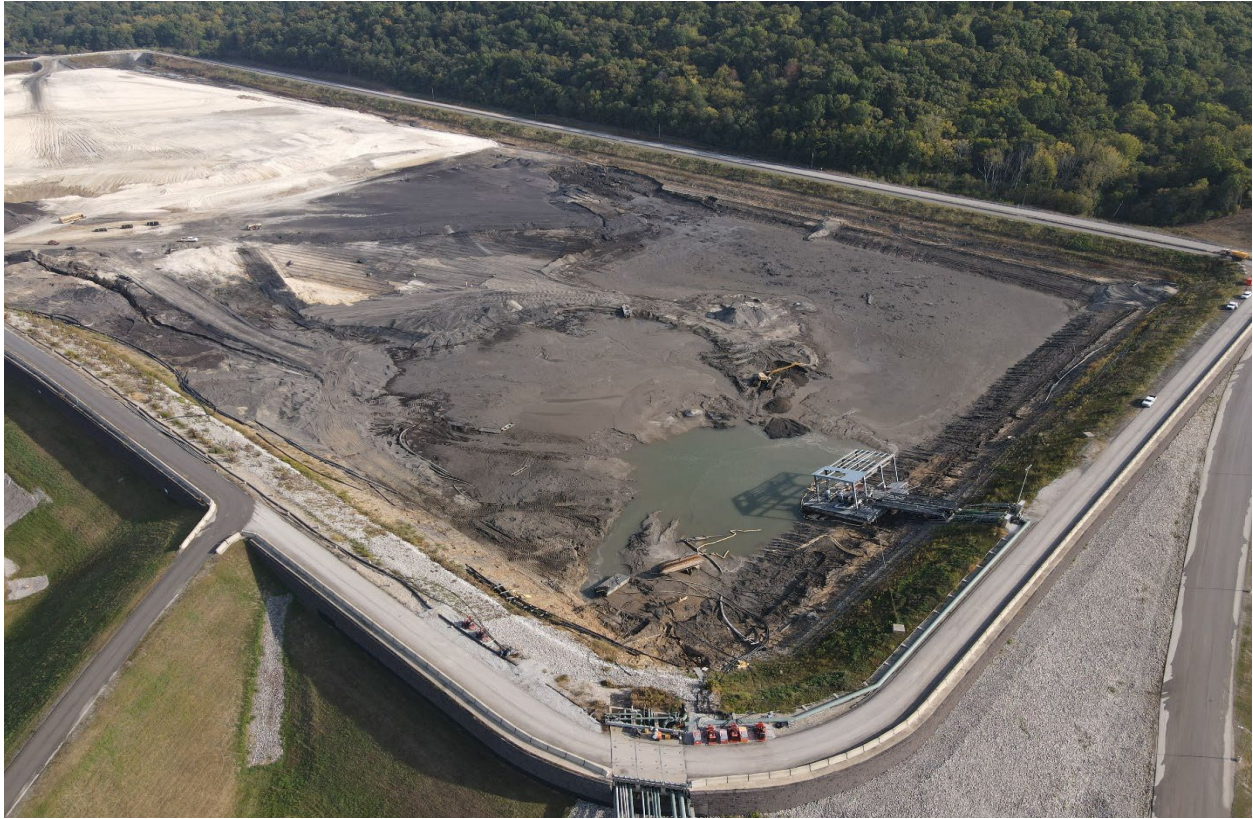
Trimble BAP – Looking Northeast – September 2023
