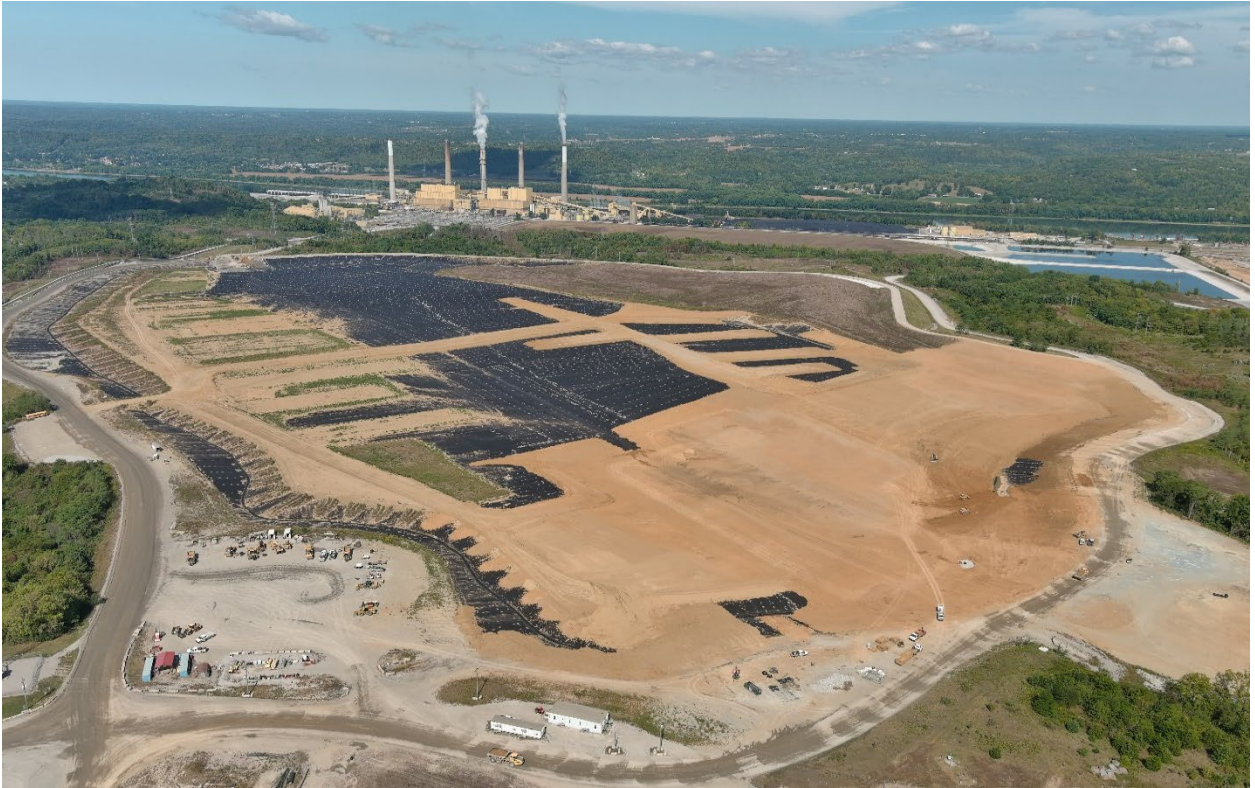
Phase III Ghent ATB #2 – September 2023
