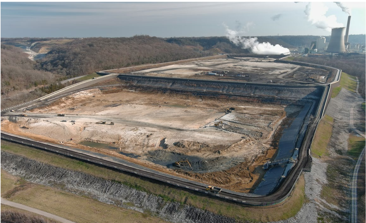
Trimble GSP – Looking South – December 2023
