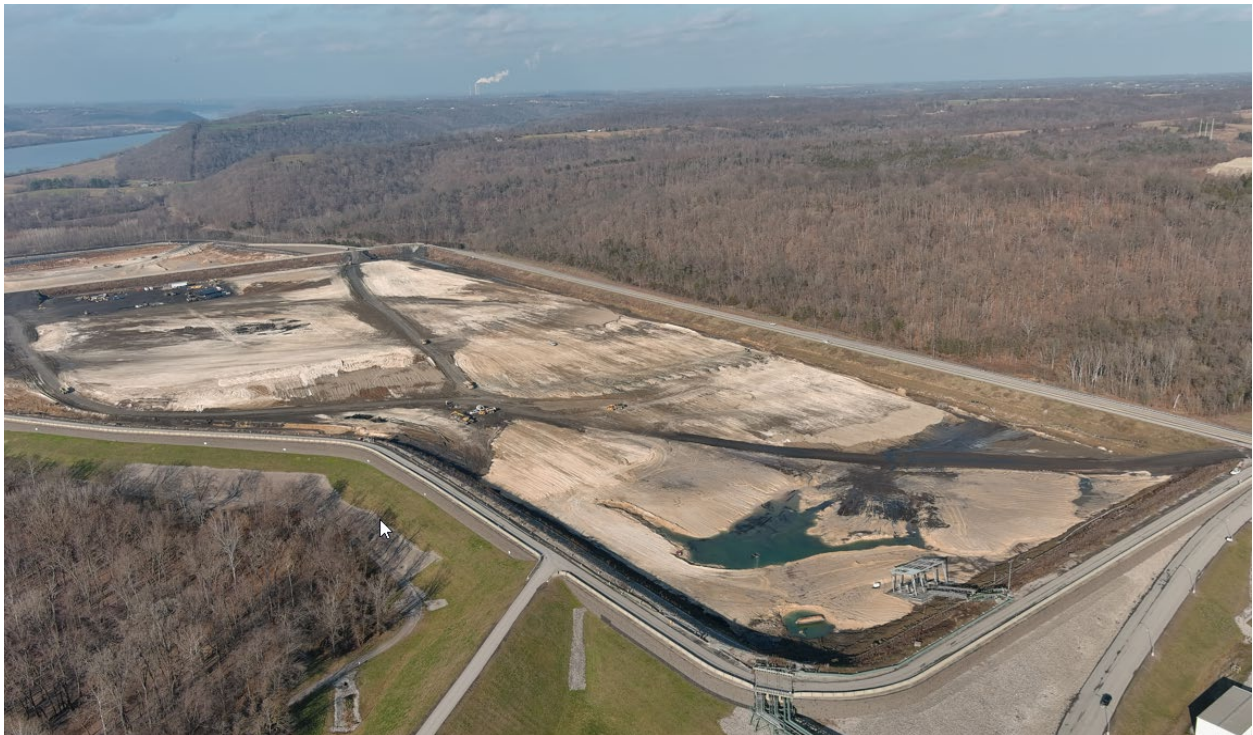
Trimble BAP – Looking Northeast – December 2023
