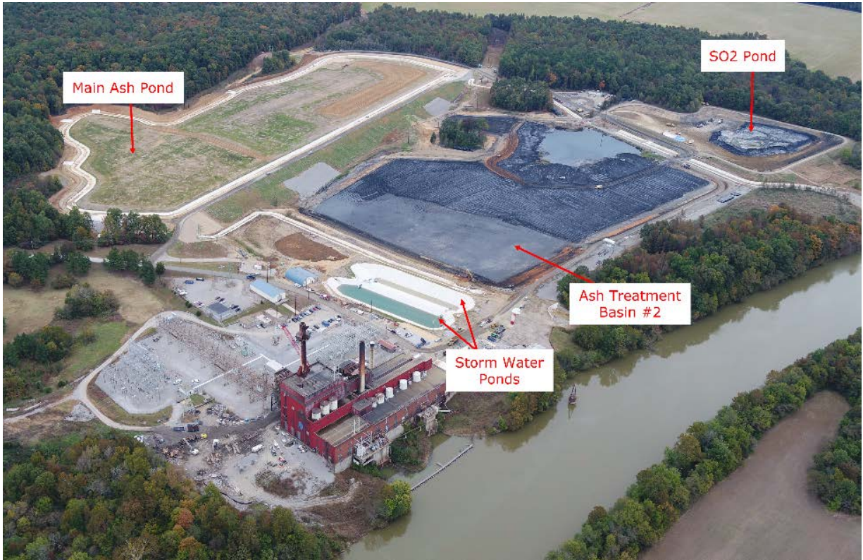
Green River CCR Impoundments – Site View – October 2018
