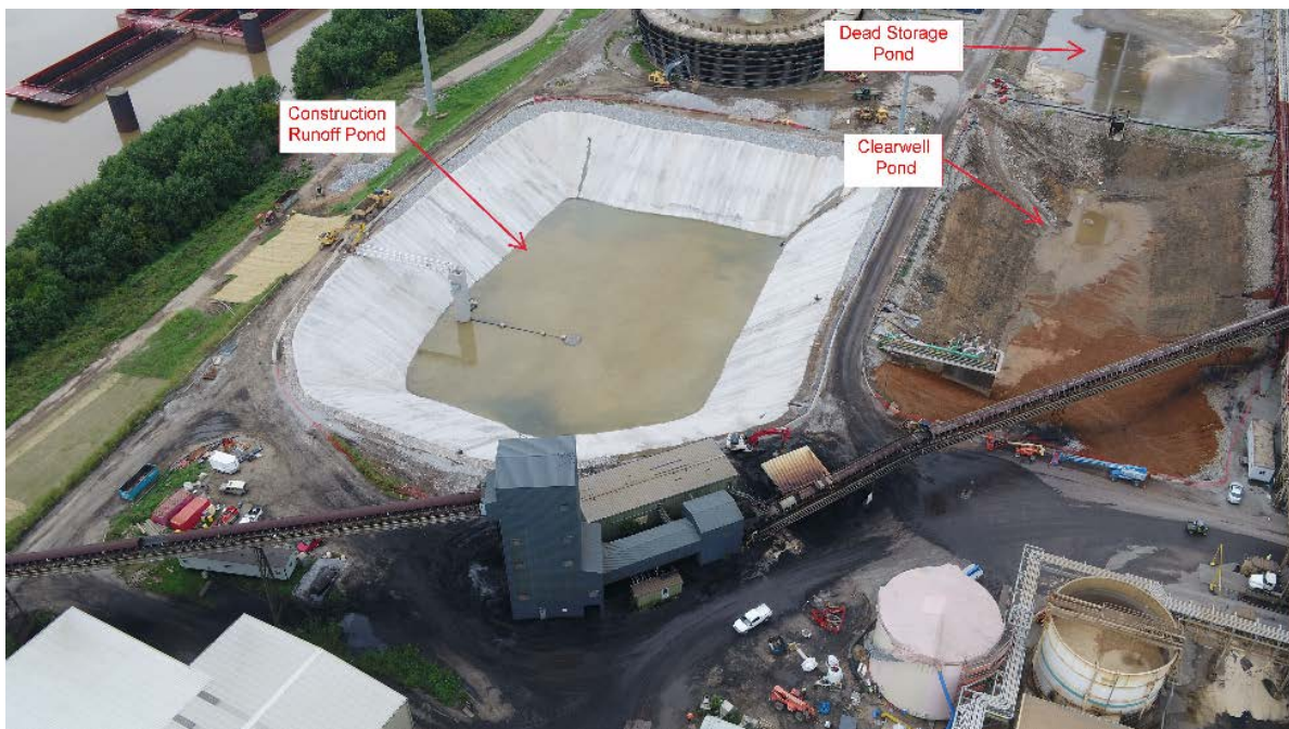
Mill Creek South Ponds – October 2018
