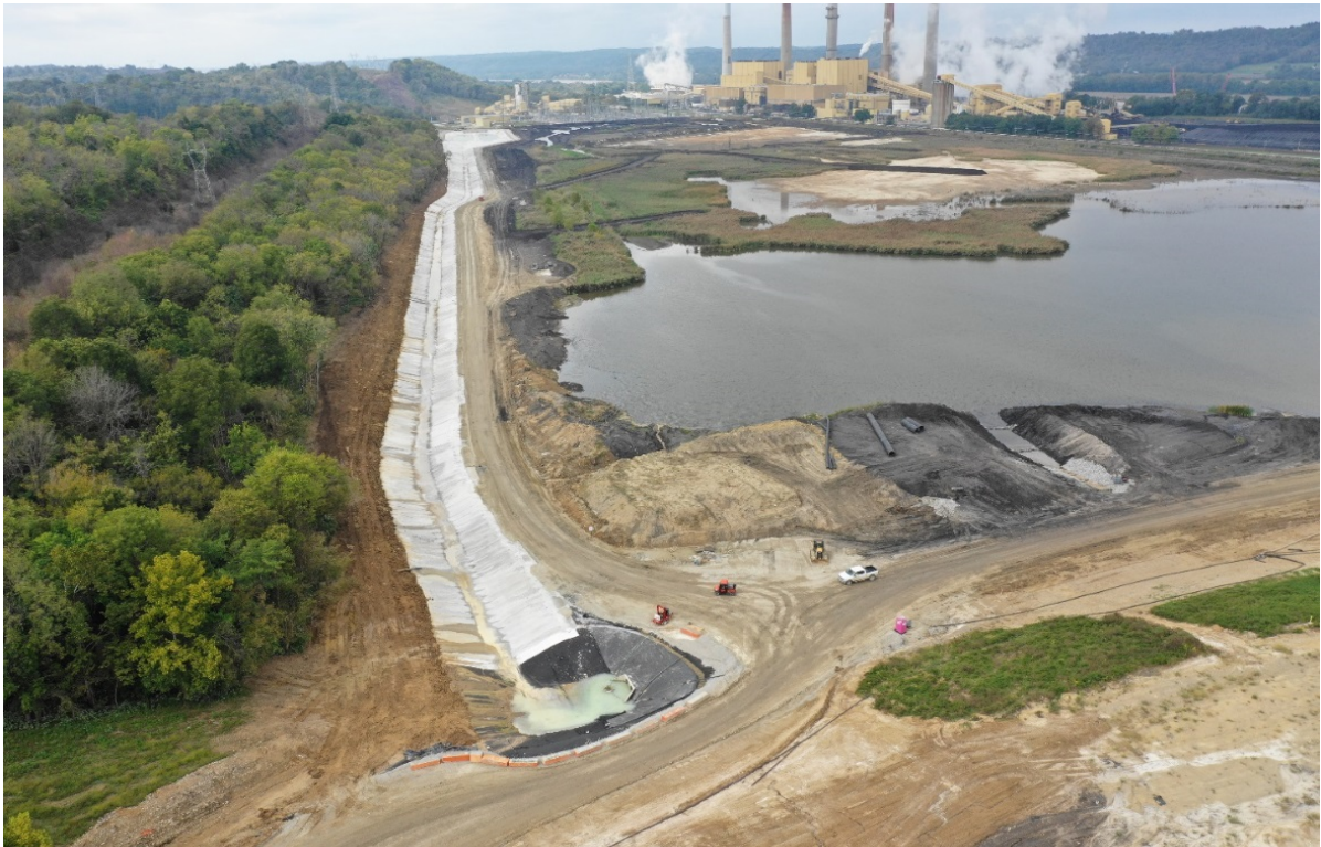
Ghent ATB #1 Cooling Channel – Looking West – October 2018
