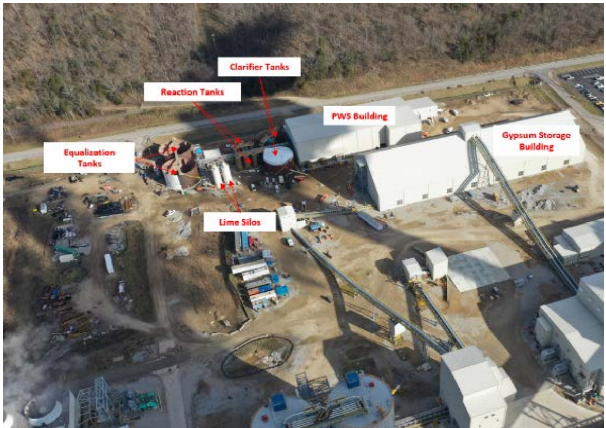
Trimble County PWS Facility – Site View Looking East – December 2018
