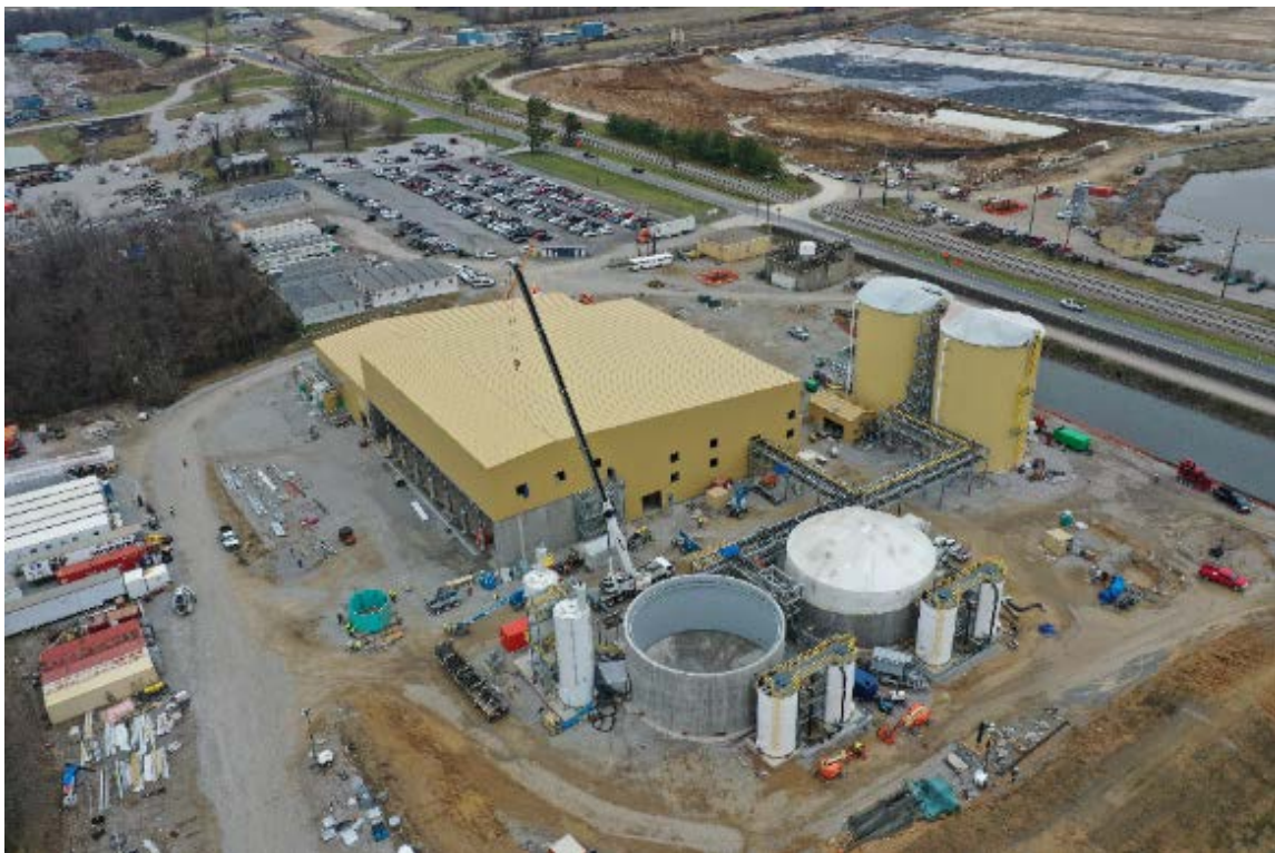
Ghent PWS Facility – Site View – January 2019
