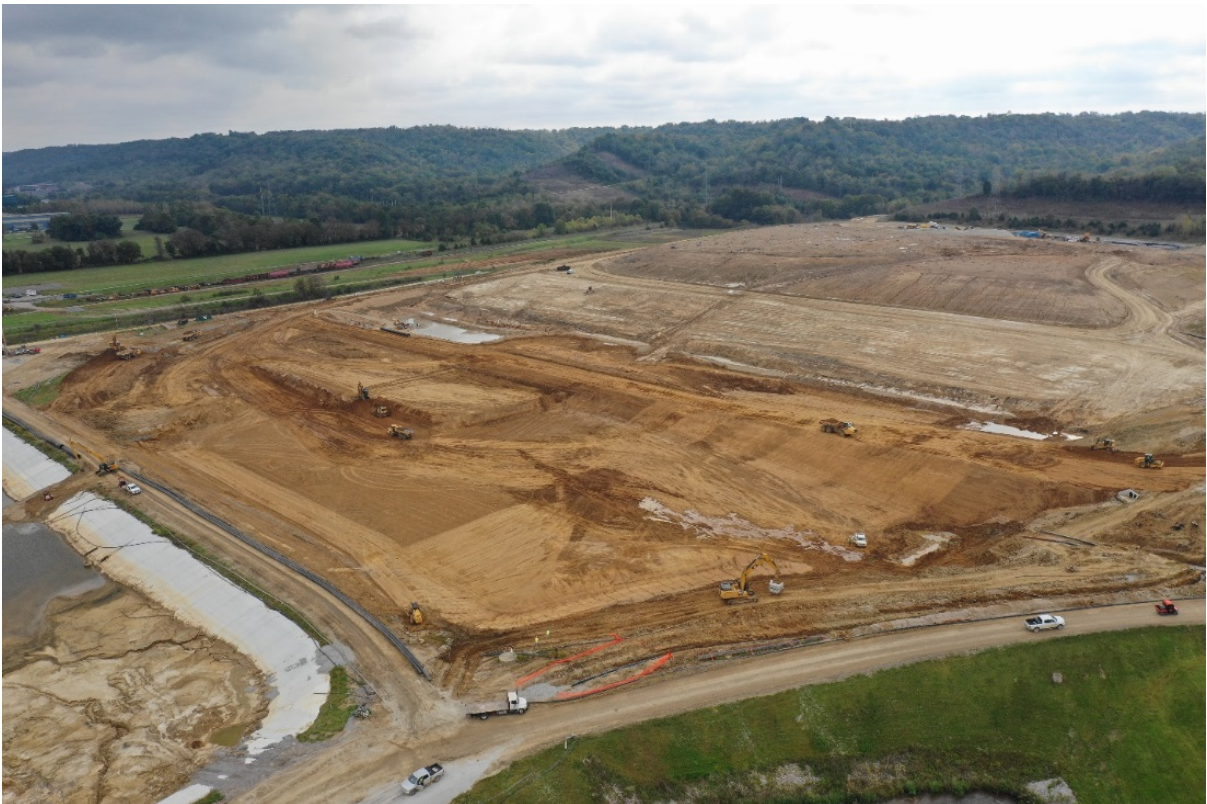
Ghent Gypsum Stack – Looking South – October 2018
