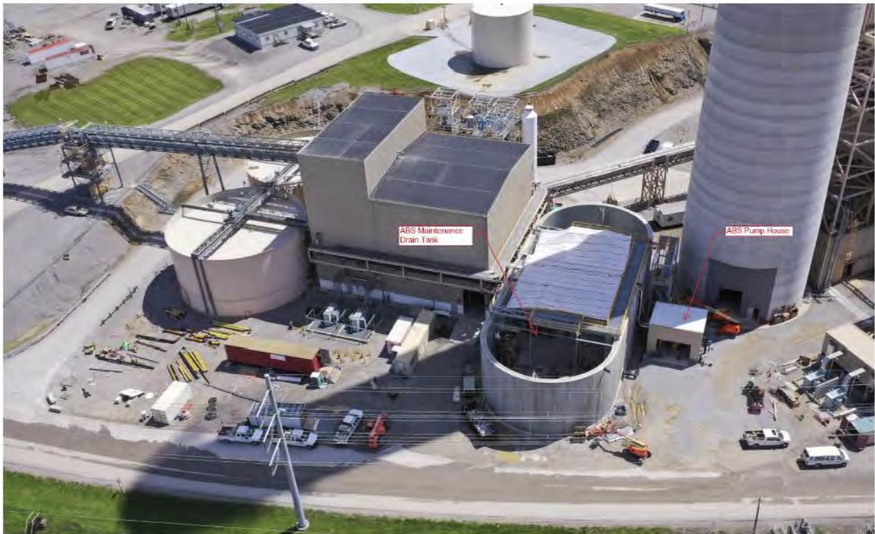
E.W. Brown ABS Maintenance Drain System – June 2019
