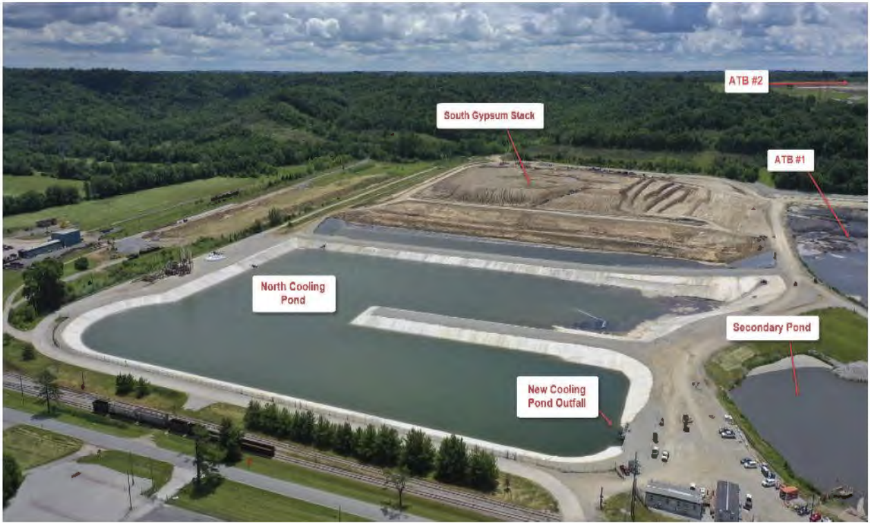
Ghent Gypsum Stack – Looking East – June 2019
