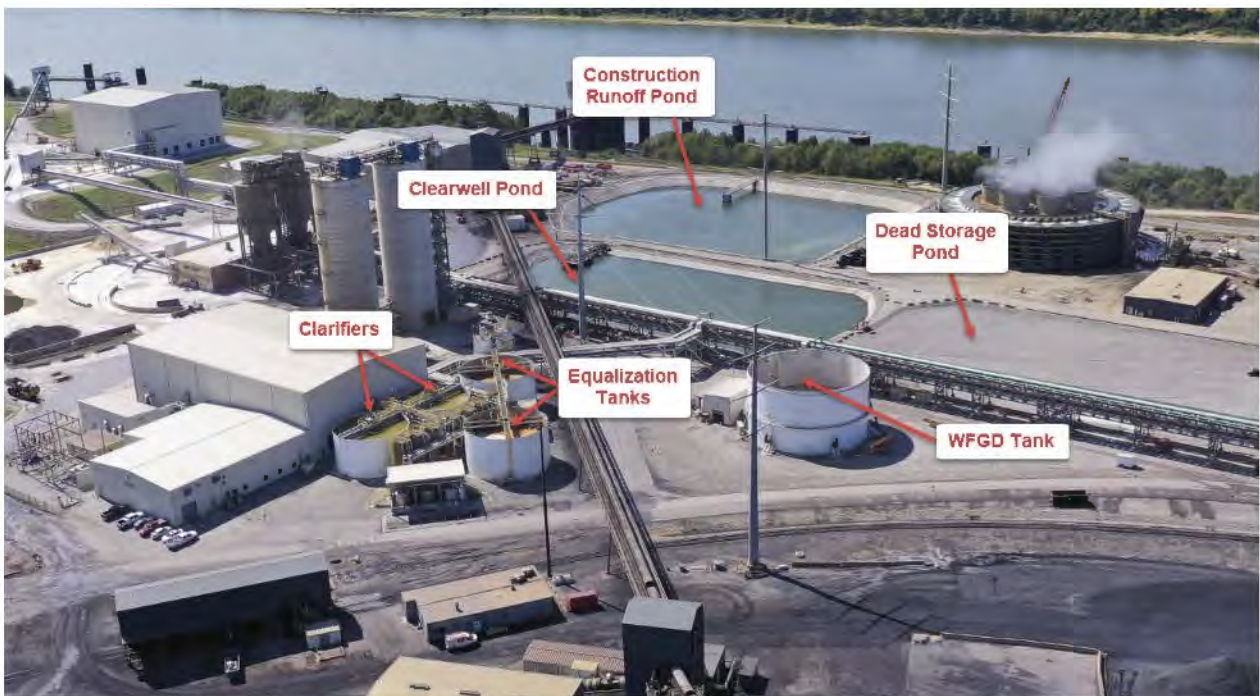
Mill Creek PWS Facility – Site View – September 2019
