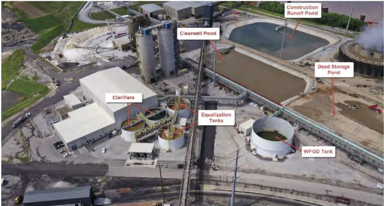
Mill Creek PWS Facility – Site View – June 2019
