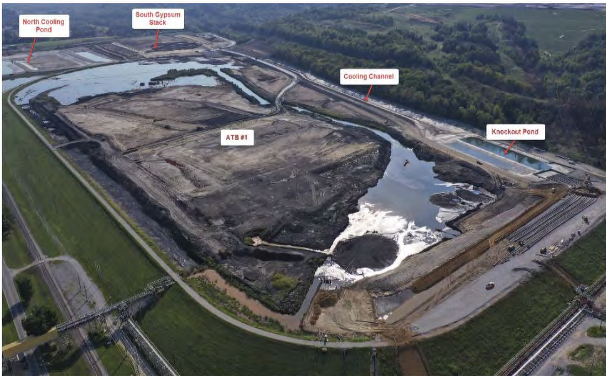
Ghent ATB #1 Cooling Channel – Looking East – September 2019
