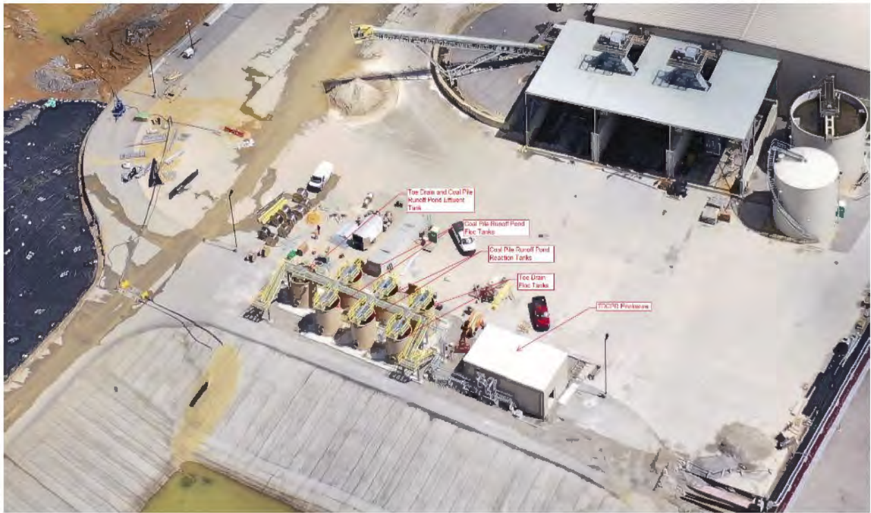
E.W. Brown Toe Drain and Coal Pile Runoff Treatment System – June 2019
