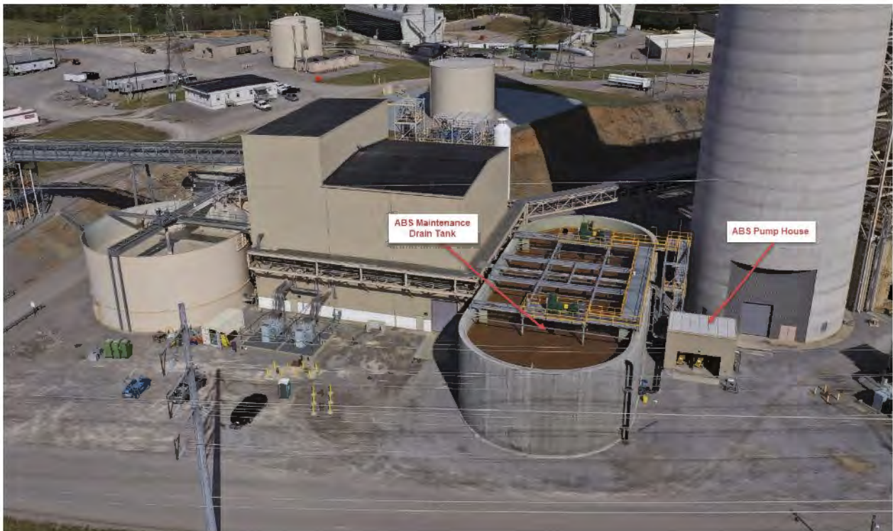
E.W. Brown ABS Maintenance Drain System – October 2019
