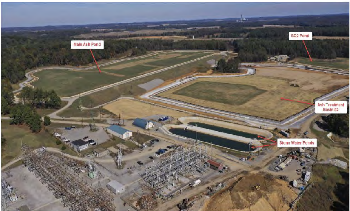
Green River CCR Impoundments – Site View – October 2019
