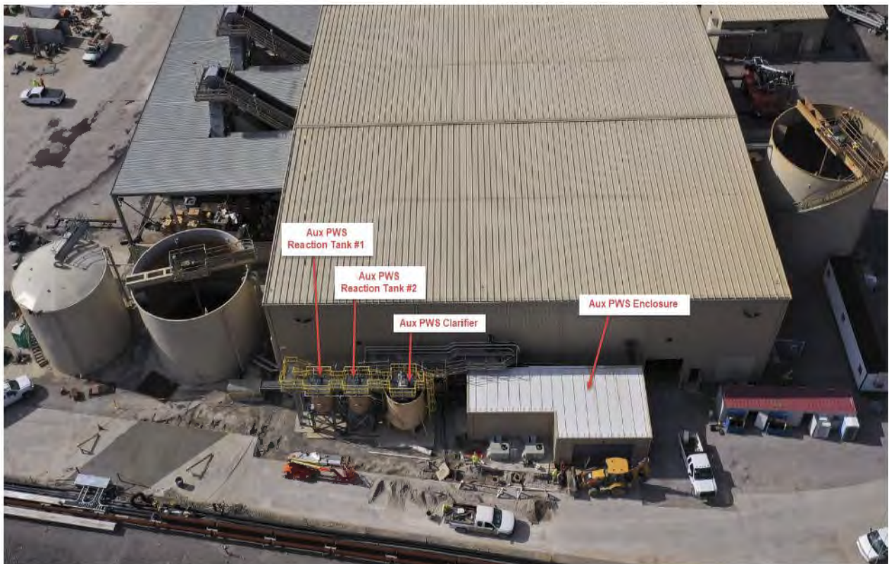
E.W. Brown PWS Treatment System – October 2019
