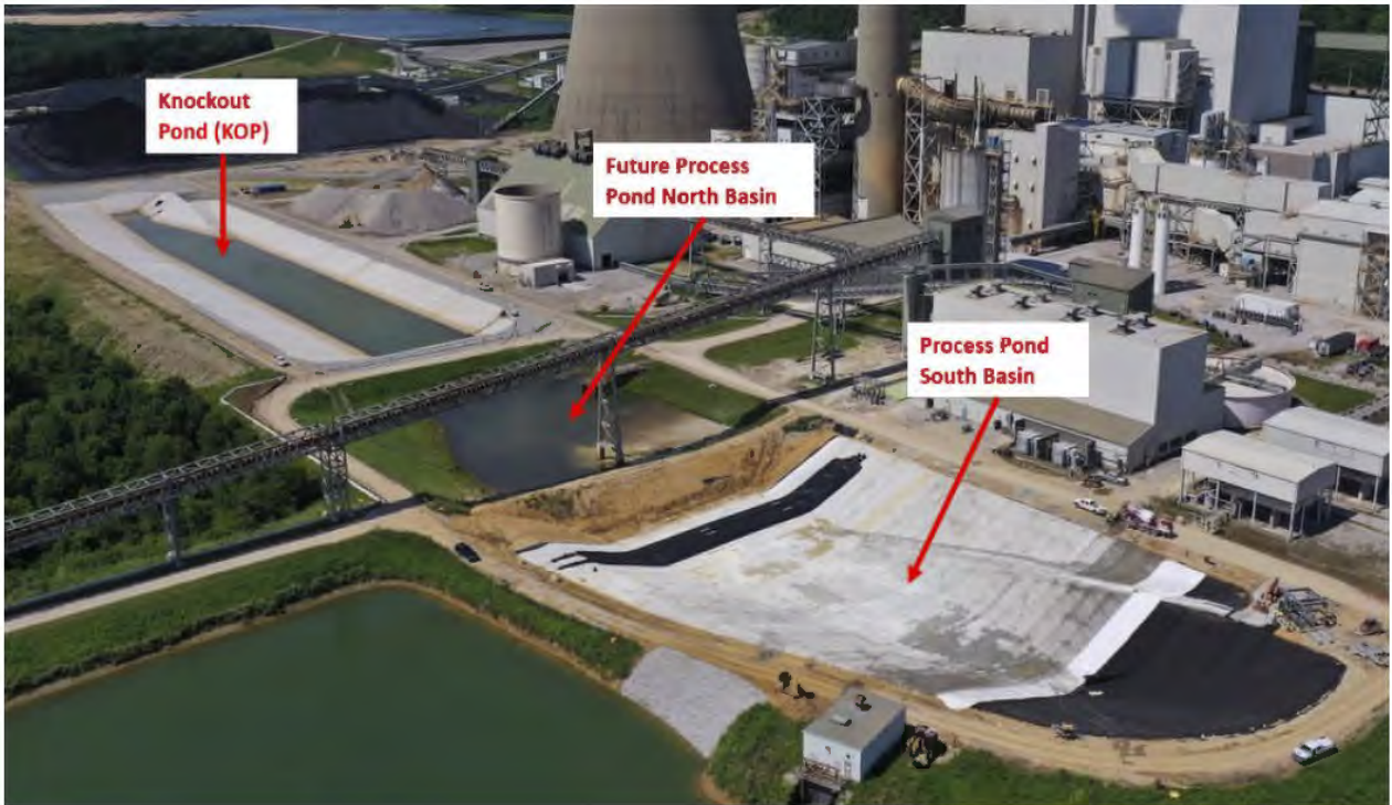
Trimble County Process Water Ponds – Looking Northeast – June 2019
