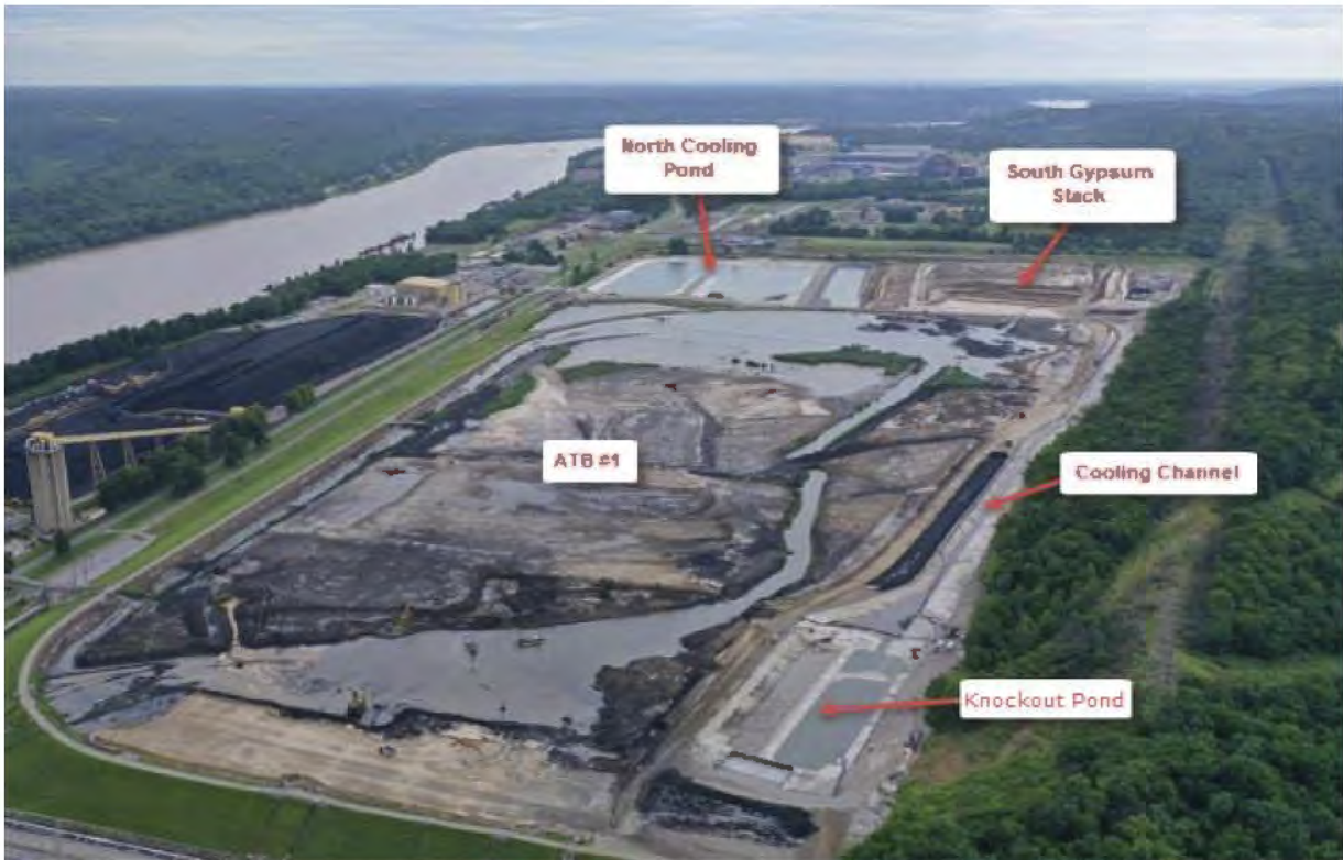
Ghent ATB #1 Cooling Channel – Looking West – June 2019
