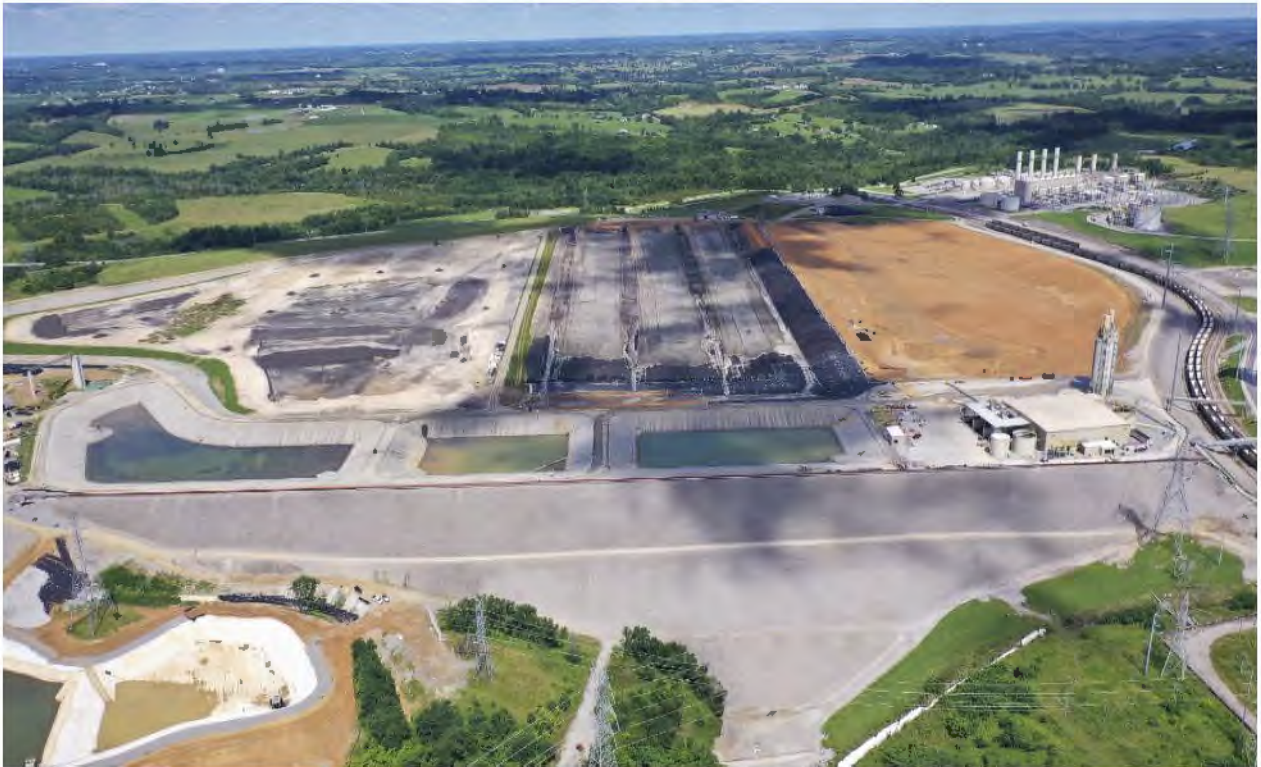
E.W. Brown Landfill Phase II and Closure – June 2019
