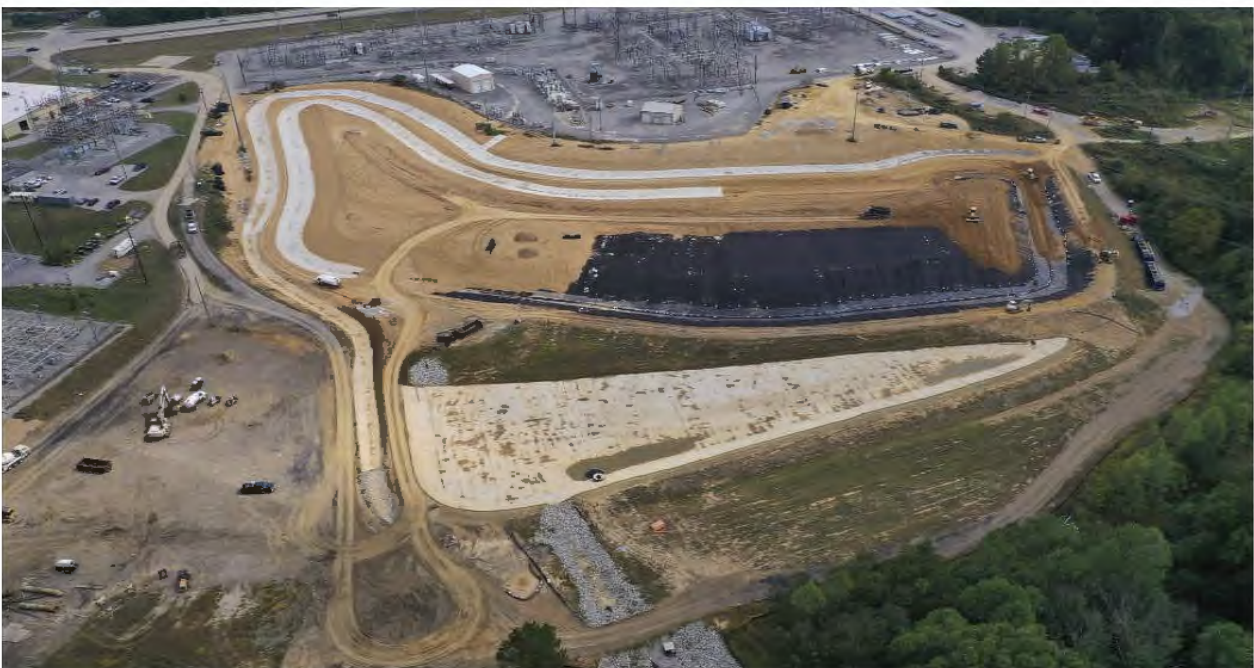
Pineville Ash Pond – September 2019
