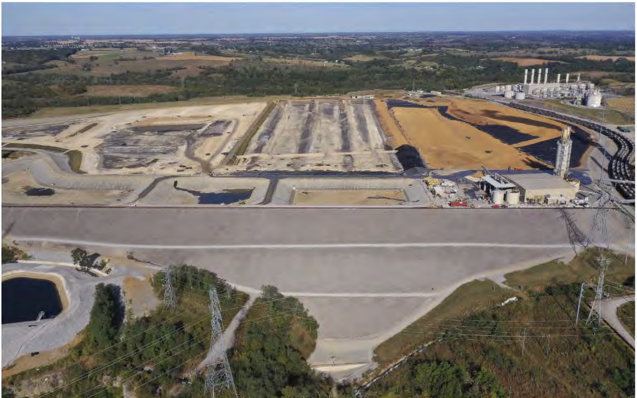
E.W. Brown Landfill Phase II and Closure – September 2019
