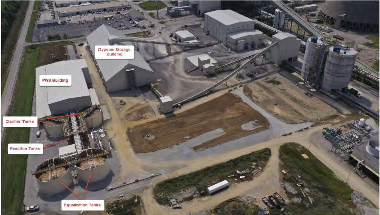
Trimble County PWS Facility – Site View Looking Southwest – September 2019
