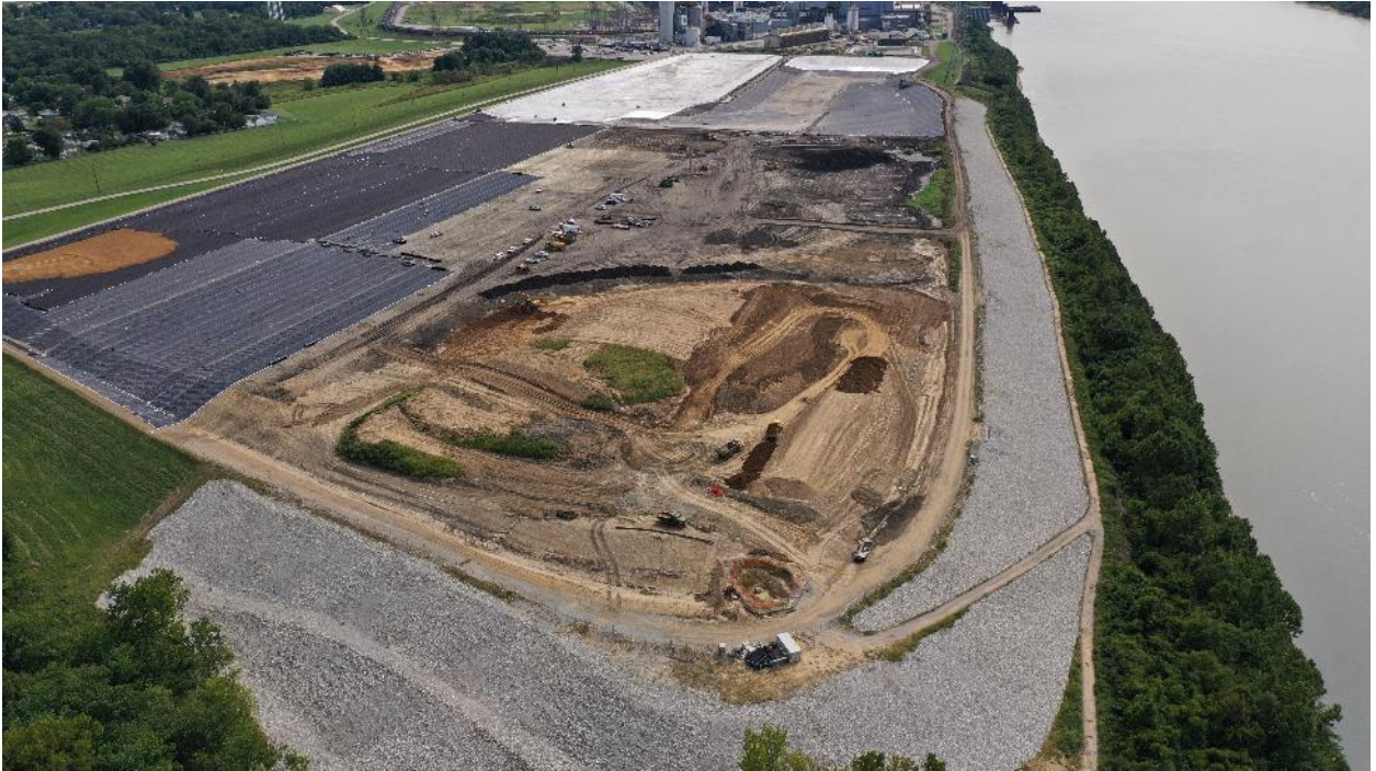
Mill Creek Main Ash Pond Closure – September 2020
