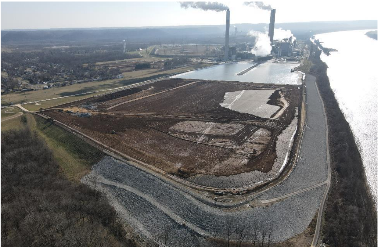
Mill Creek Main Ash Pond Closure – January 2021
