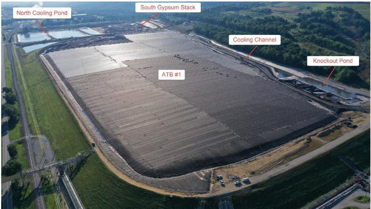
Ghent ATB #1 and Cooling Channel – Looking East – July 2020
