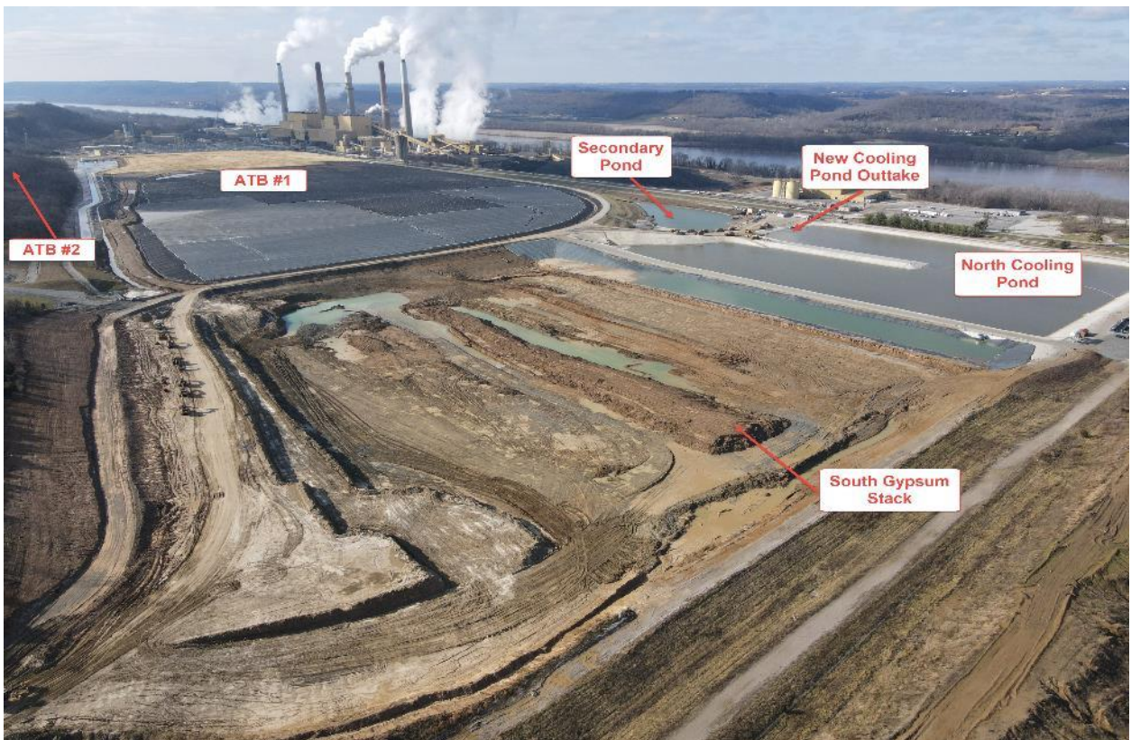
Ghent Gypsum Stack – Looking North – January 2021
