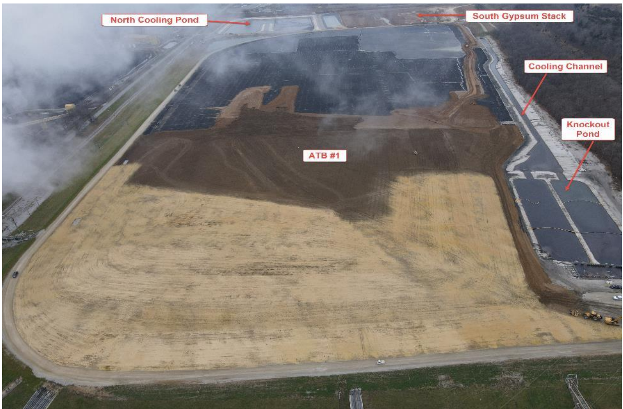
Ghent ATB #1 and Cooling Channel – Looking East – December 2020
