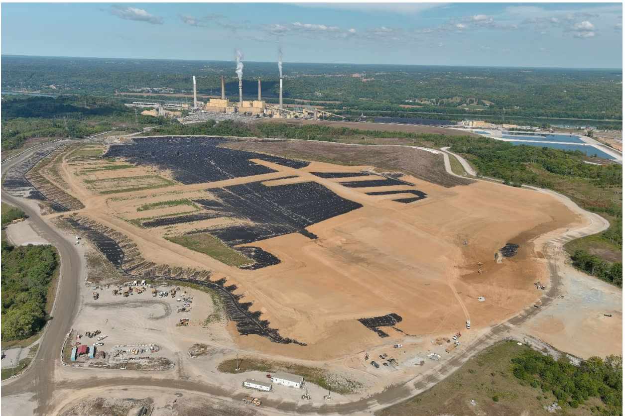
Phase III Ghent ATB #2 – September 2023
