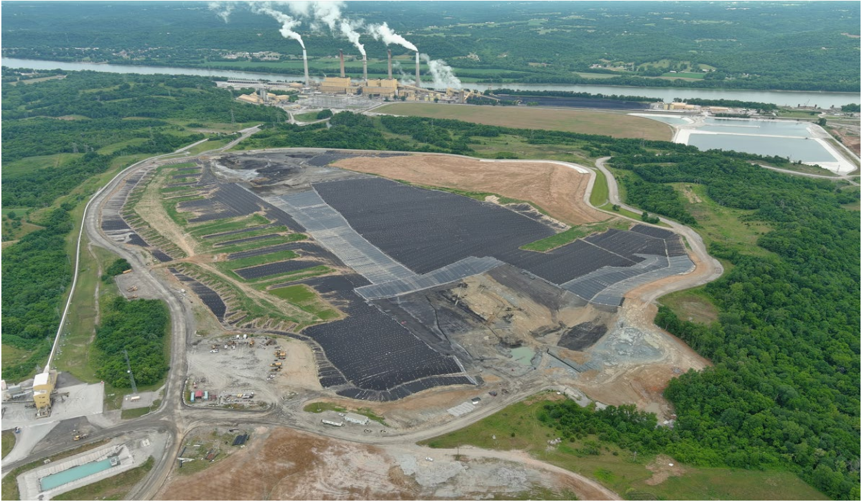
Phase III Ghent ATB #2 – June 2023
