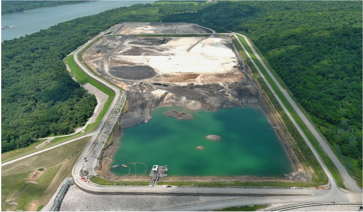
Trimble BAP – Looking North – July 2023
