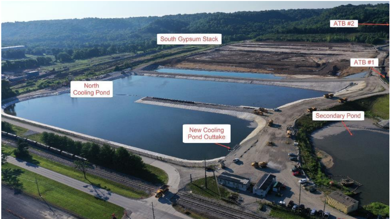
Ghent Gypsum Stack – Looking East – July 2020
