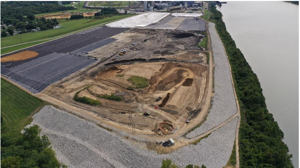
Mill Creek Main Ash Pond Closure – September 2020
