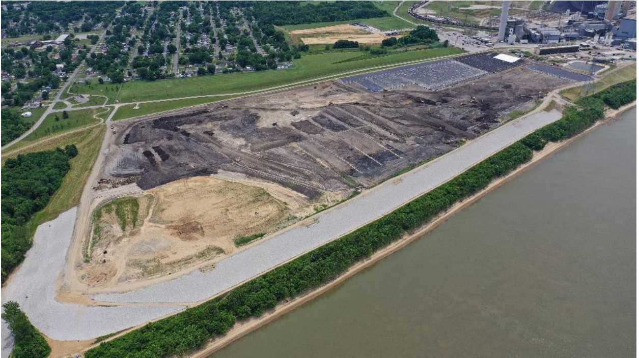
Mill Creek Main Ash Pond Closure – June 2020
