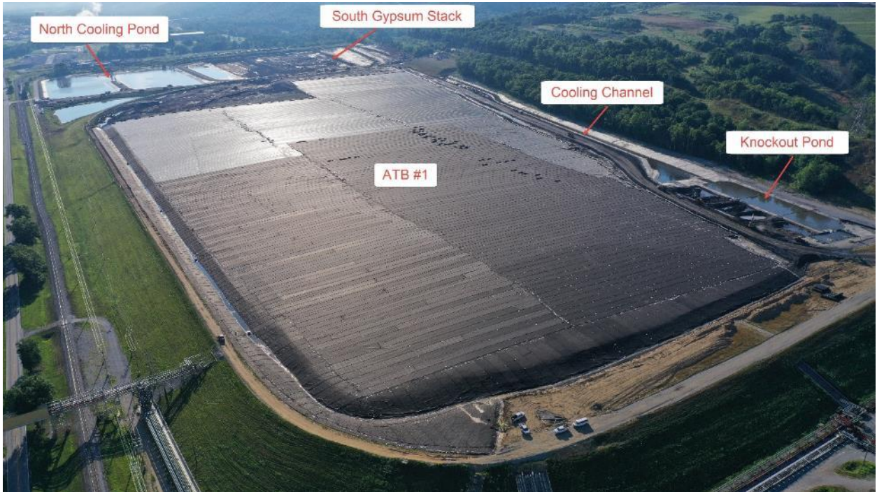
Ghent ATB #1 and Cooling Channel – Looking East – July 2020
