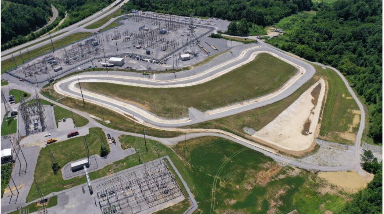
Pineville Ash Pond – July 2020 – Completed
