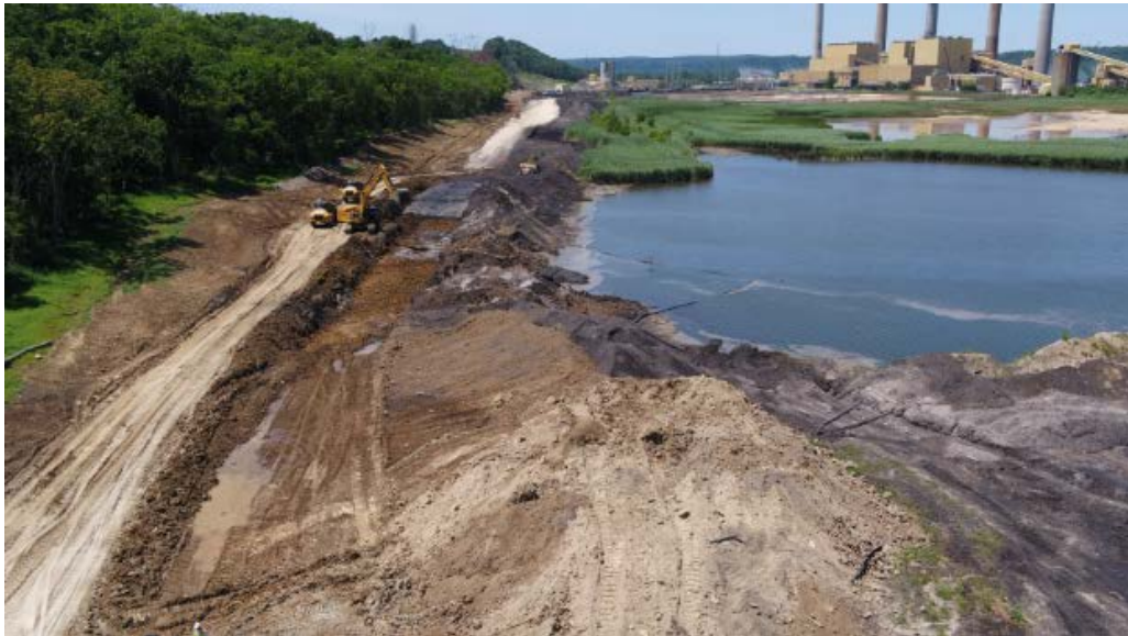
Ghent ATB #1 Cooling Channel – Looking West – Photo from the July 2018 Report
