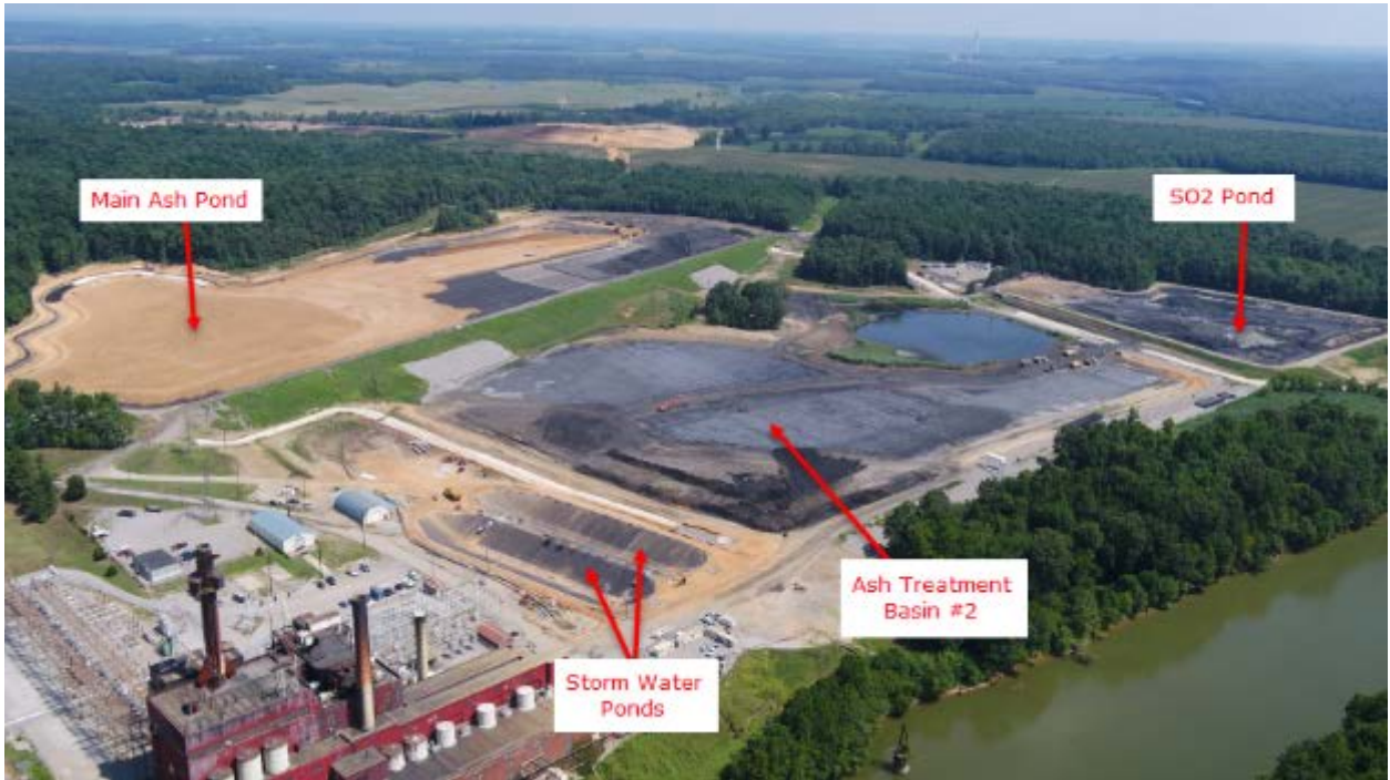
Green River CCR Impoundments – Site View - Photo from the July 2018 Report
