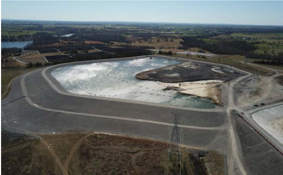
E.W. Brown Aux Pond – Pre-Construction – Photo from the July 2018 Report
