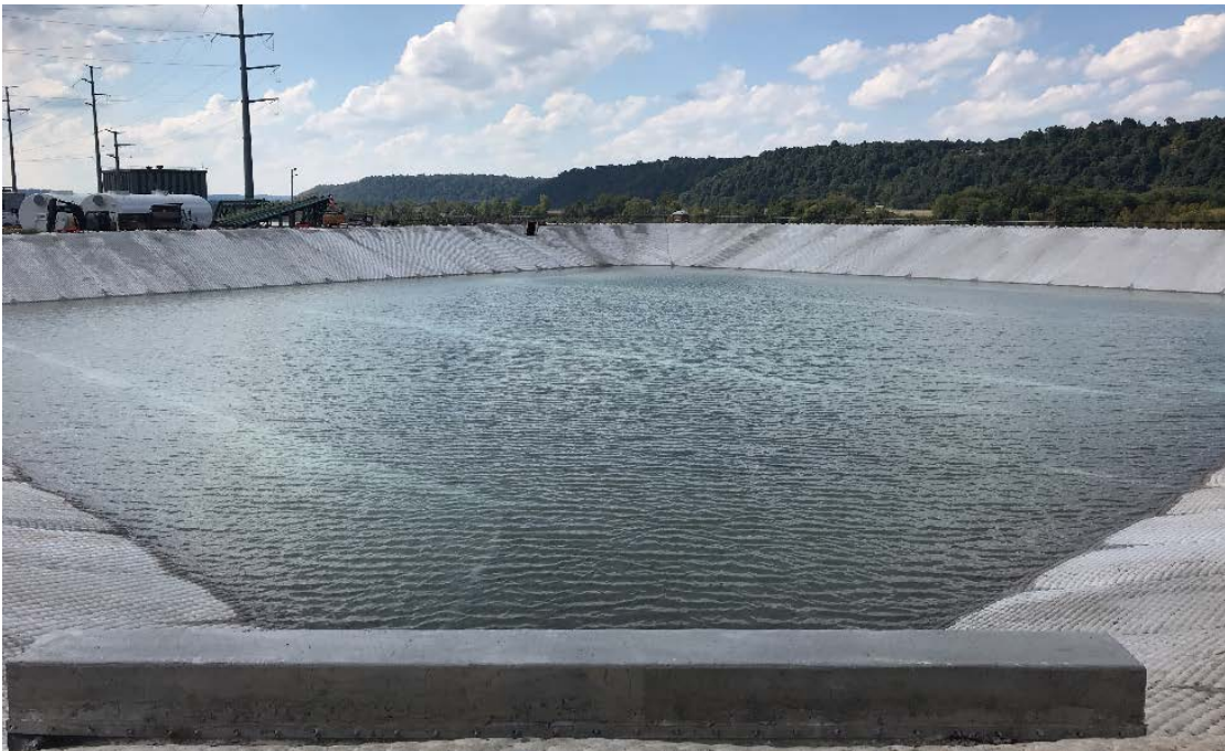
Mill Creek Knock-Out Pond – October 2018
