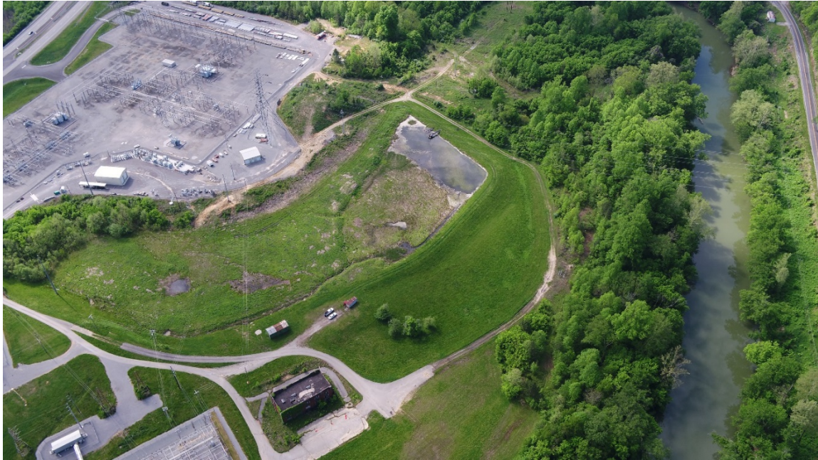
Pineville Ash Pond – Photo from July 2018 Report
