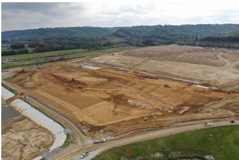
Ghent Gypsum Stack – Looking South – October 2018
