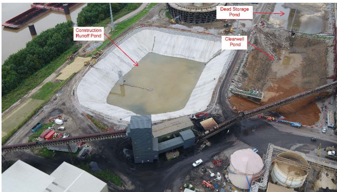
Mill Creek South Ponds – October 2018
