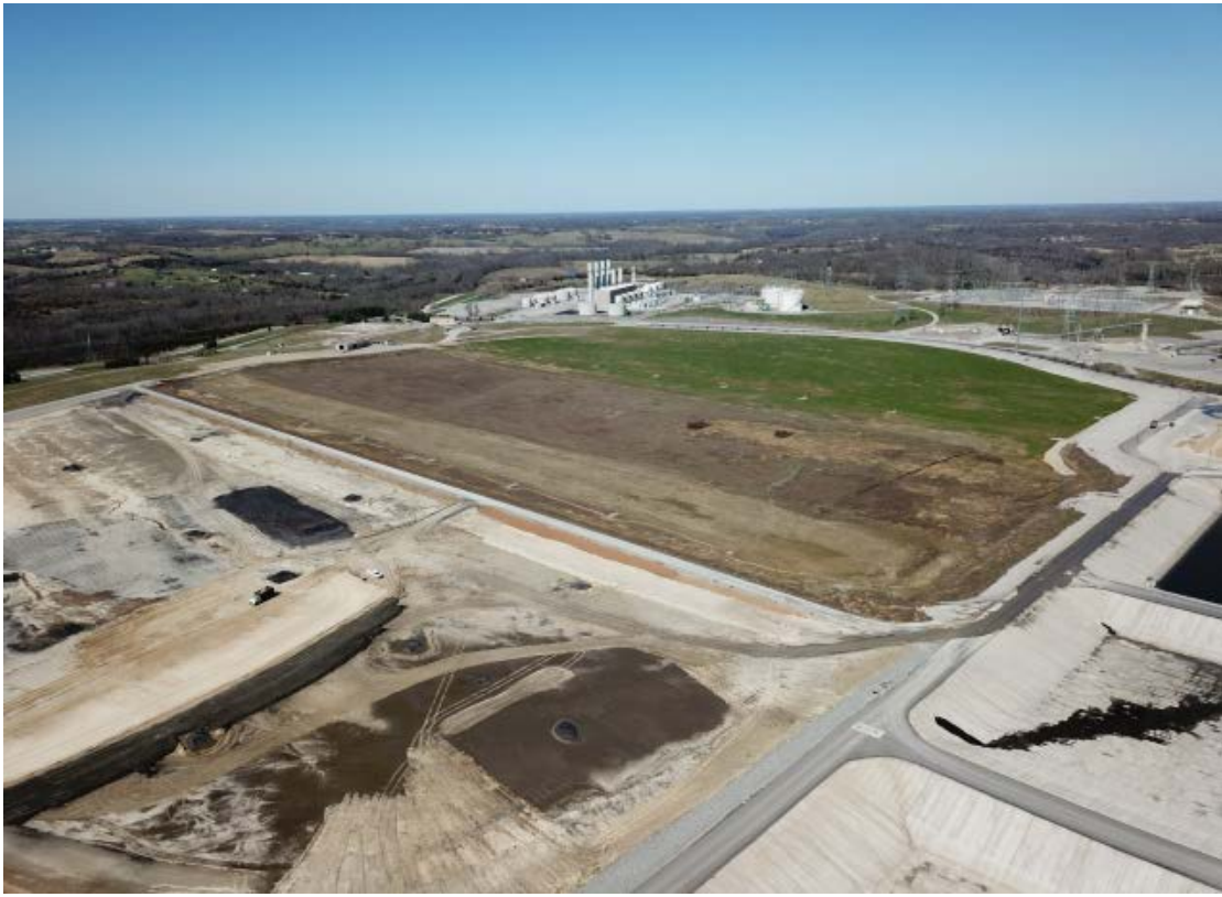
E.W. Brown Landfill Phase II and Closure – Pre-Construction – July 2018 Report
