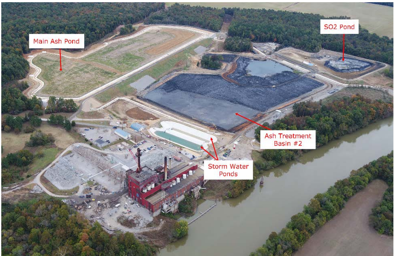
Green River CCR Impoundments – Site View – October 2018
