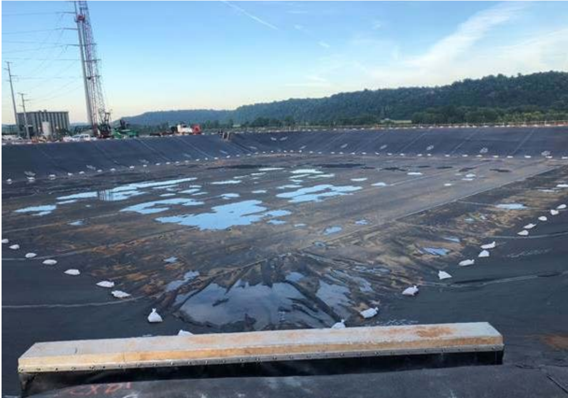
Mill Creek Knock-Out Pond – Photo from the July 2018 Report
