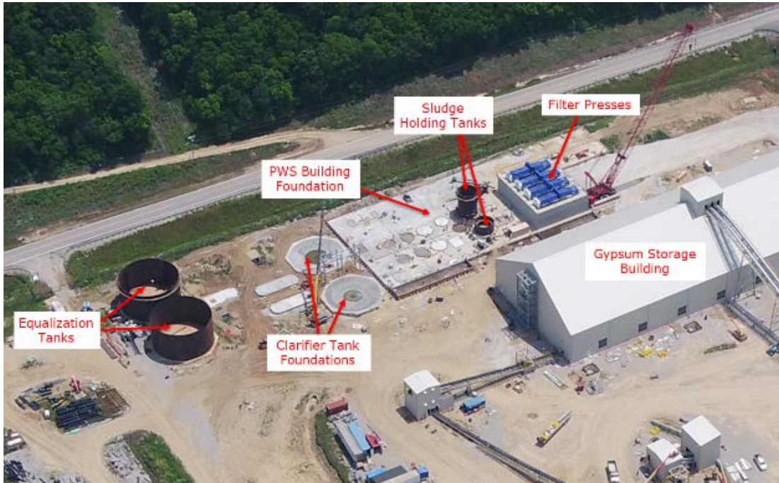
Trimble County PWS Facility – Site View – Photo from the July 2018 Report
