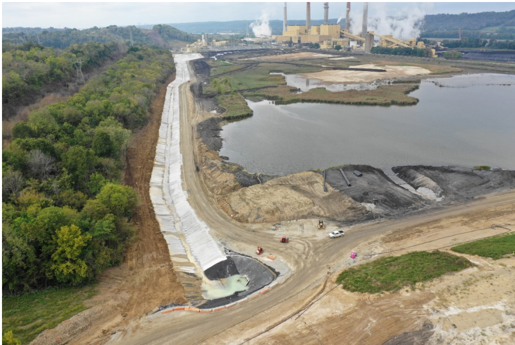
Ghent ATB #1 Cooling Channel – Looking West – October 2018
