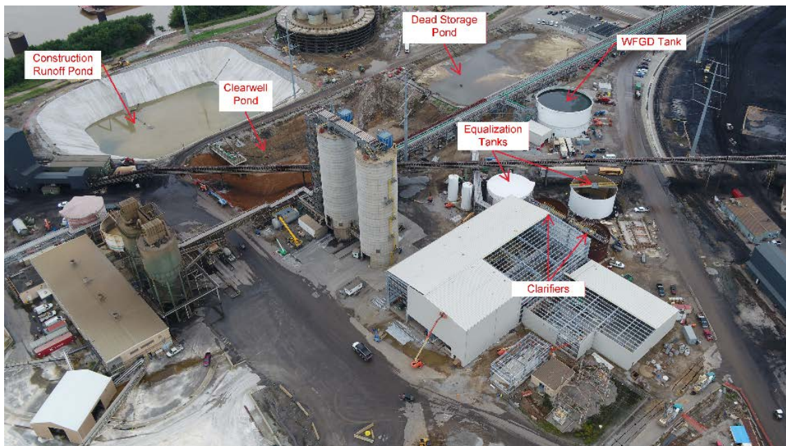
Mill Creek PWS Facility – Site View – October 2018
