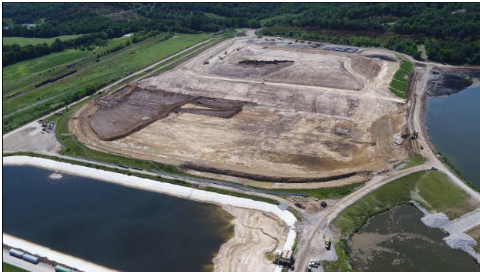
Ghent Gypsum Stack – Looking South – Photo from the July 2018 Report
