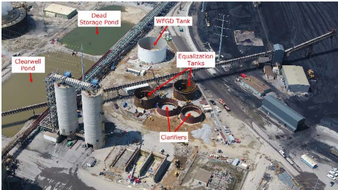
Mill Creek PWS Facility – Site View – Photo from the July 2018 Report
