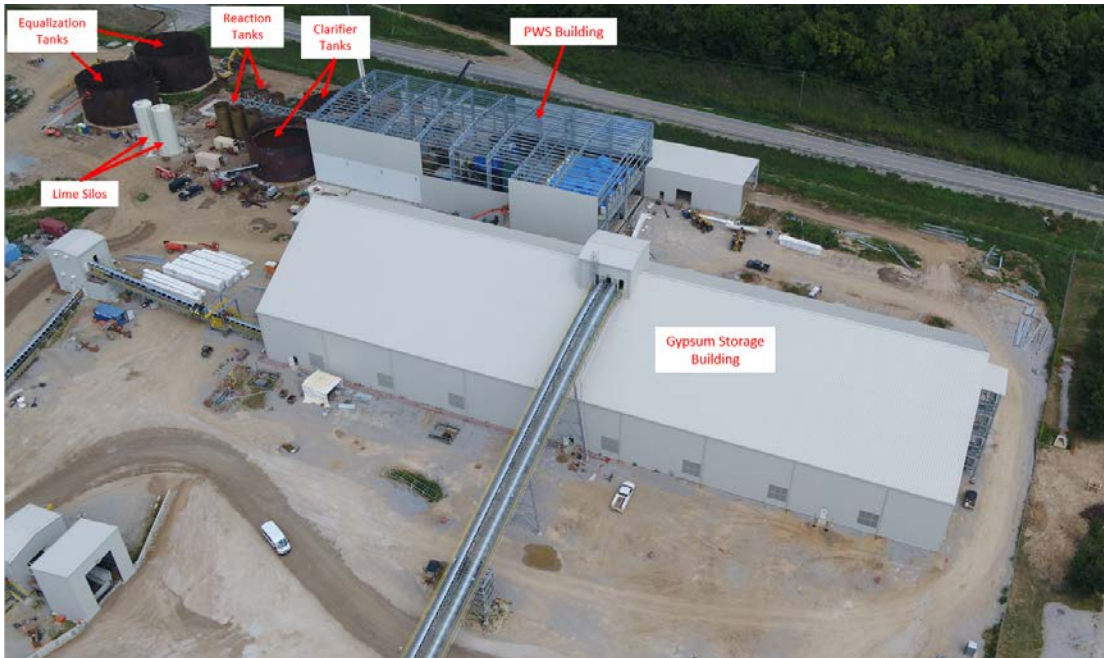
Trimble County PWS Facility – Site View Looking West – October 2018
