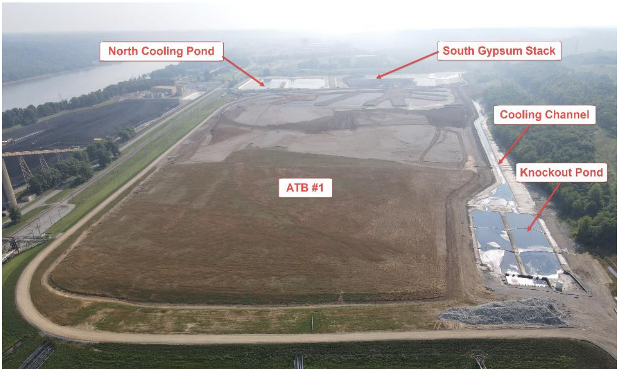
Ghent ATB #1 and Cooling Channel – Looking East – June 2021
