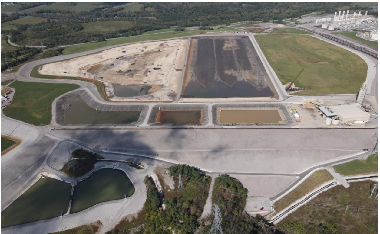
E.W. Brown Landfill Phase II and Closure – October 2021
