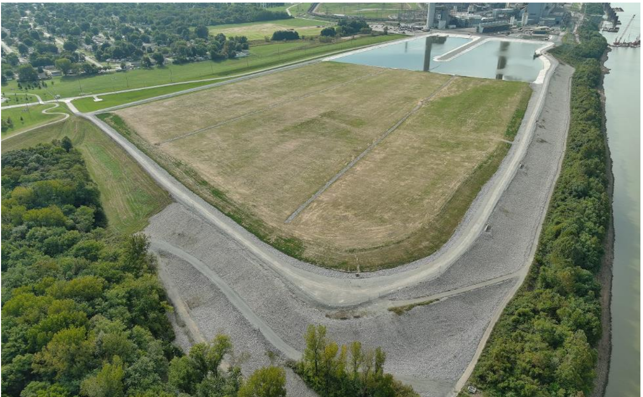
Mill Creek Main Ash Pond Closure – October 2021
