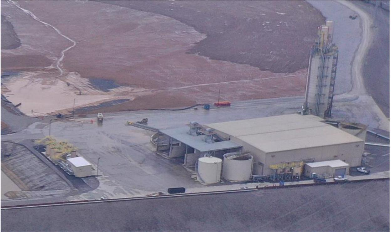
*E.W. Brown Toe Drain and Coal Pile Runoff Treatment System – March 2020*
