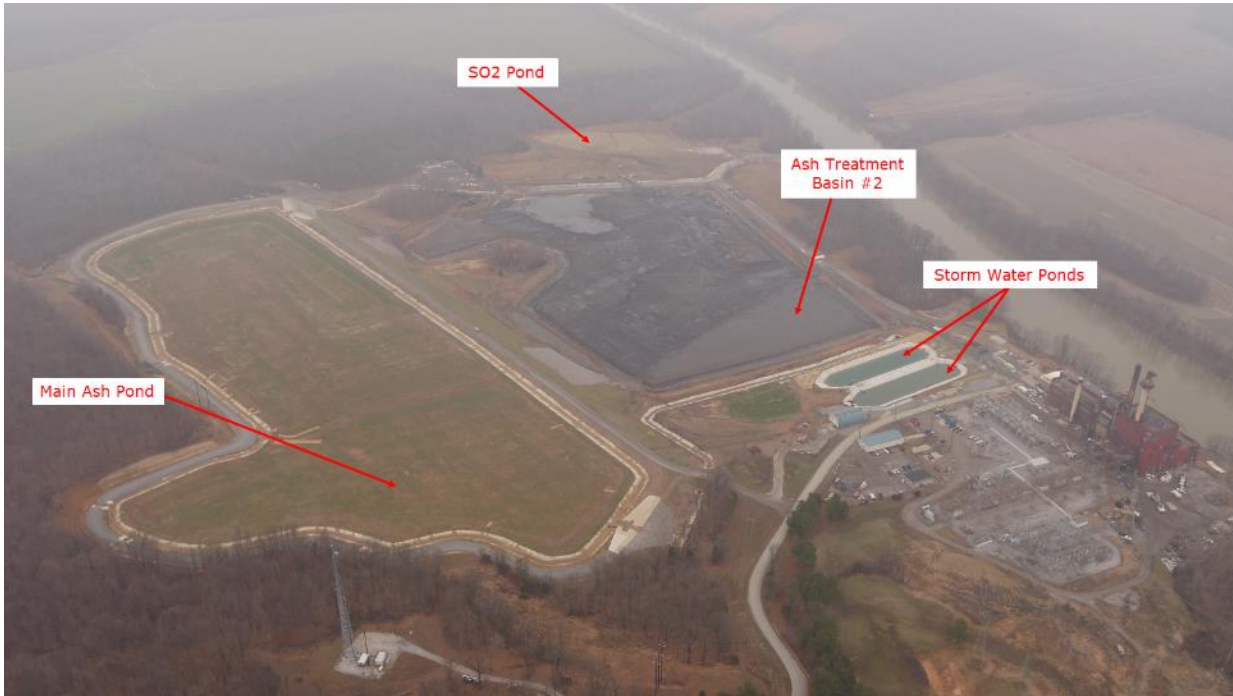
Green River CCR Impoundments – Site View – January 2019
