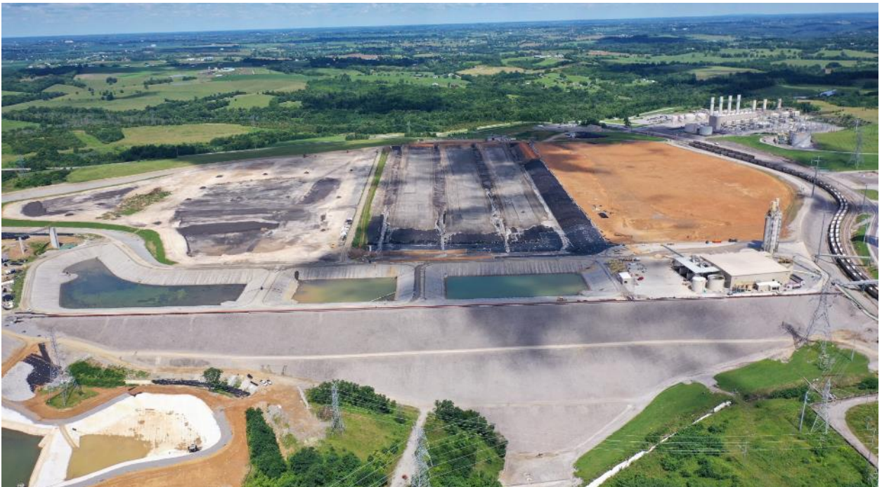
E.W. Brown Landfill Phase II and Closure – June 2019
