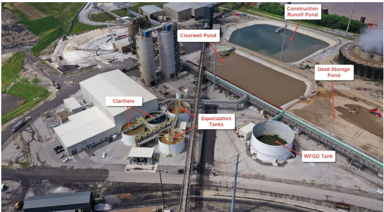
Mill Creek PWS Facility – Site View – June 2019
