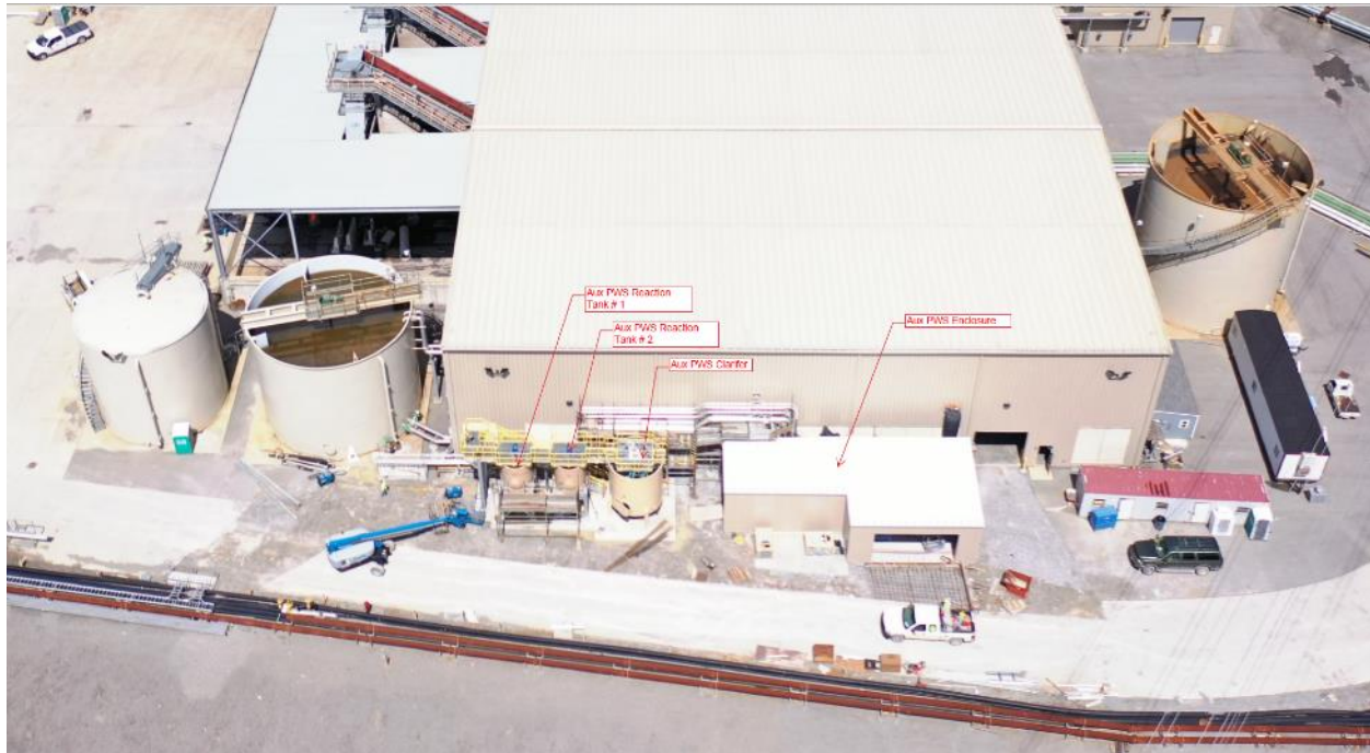
E. W. Brown PWS Treatment System – June 2019
