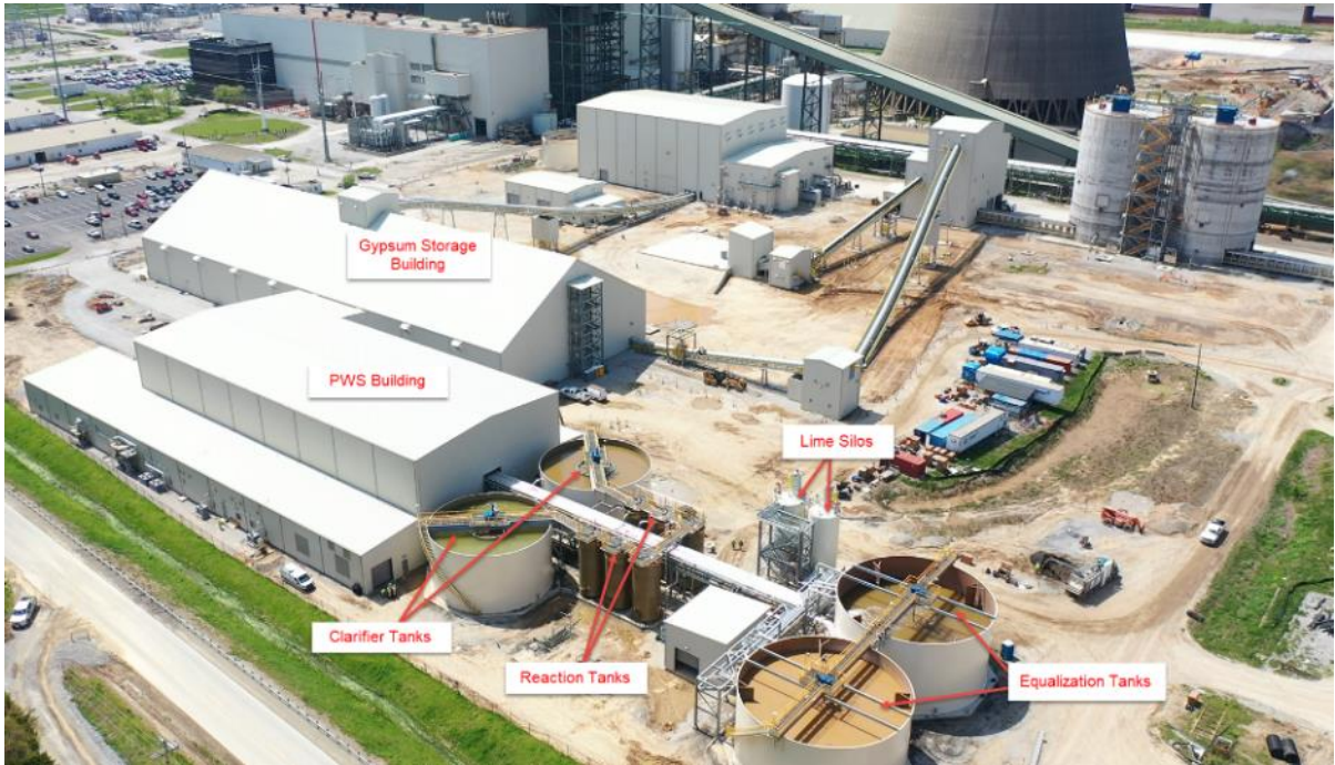
Trimble County PWS Facility – Site View Looking West – April 2019
