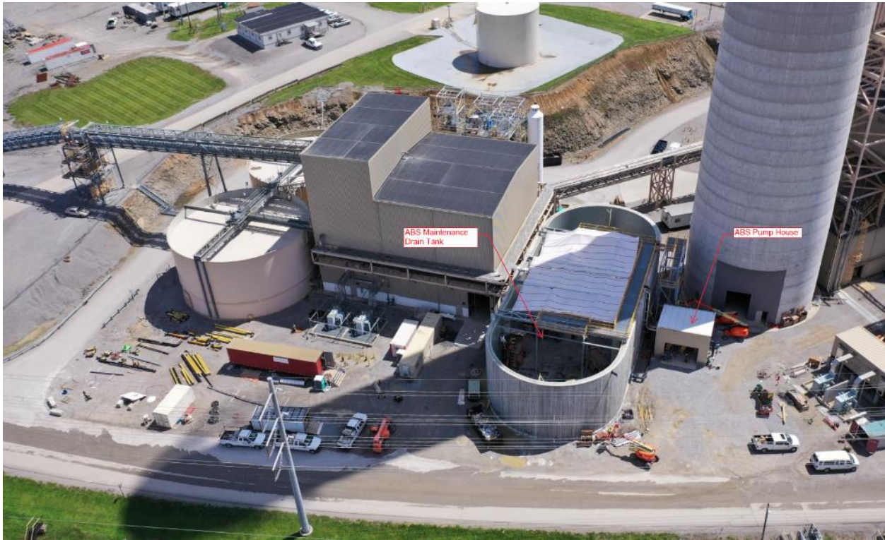
E.W. Brown ABS Maintenance Drain System – June 2019
