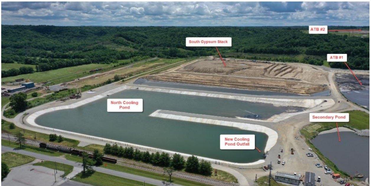
Ghent Gypsum Stack – Looking East – June 2019
