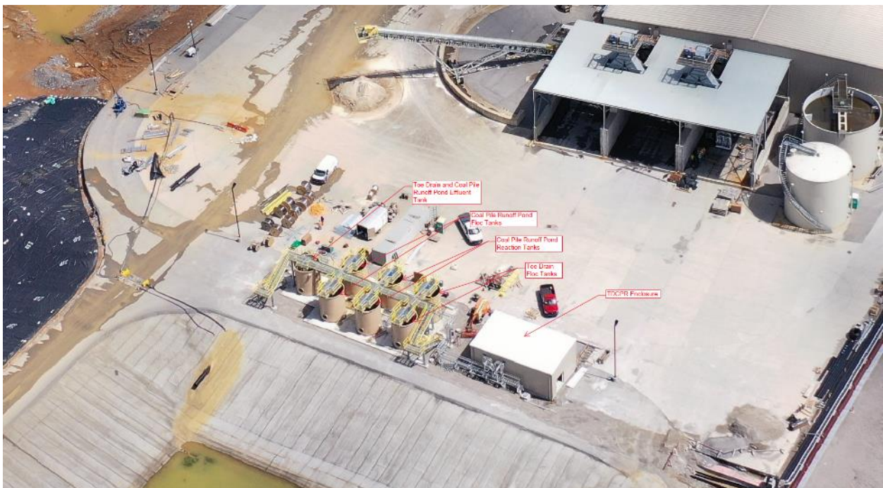
E.W. Brown Toe Drain and Coal Pile Runoff Treatment System – June 2019
