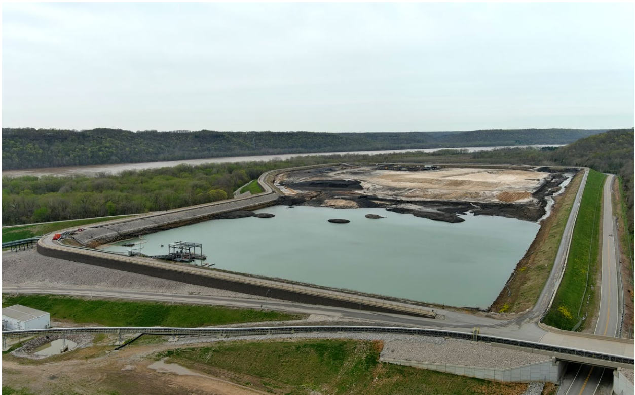
Trimble BAP – Looking North – April 2023
