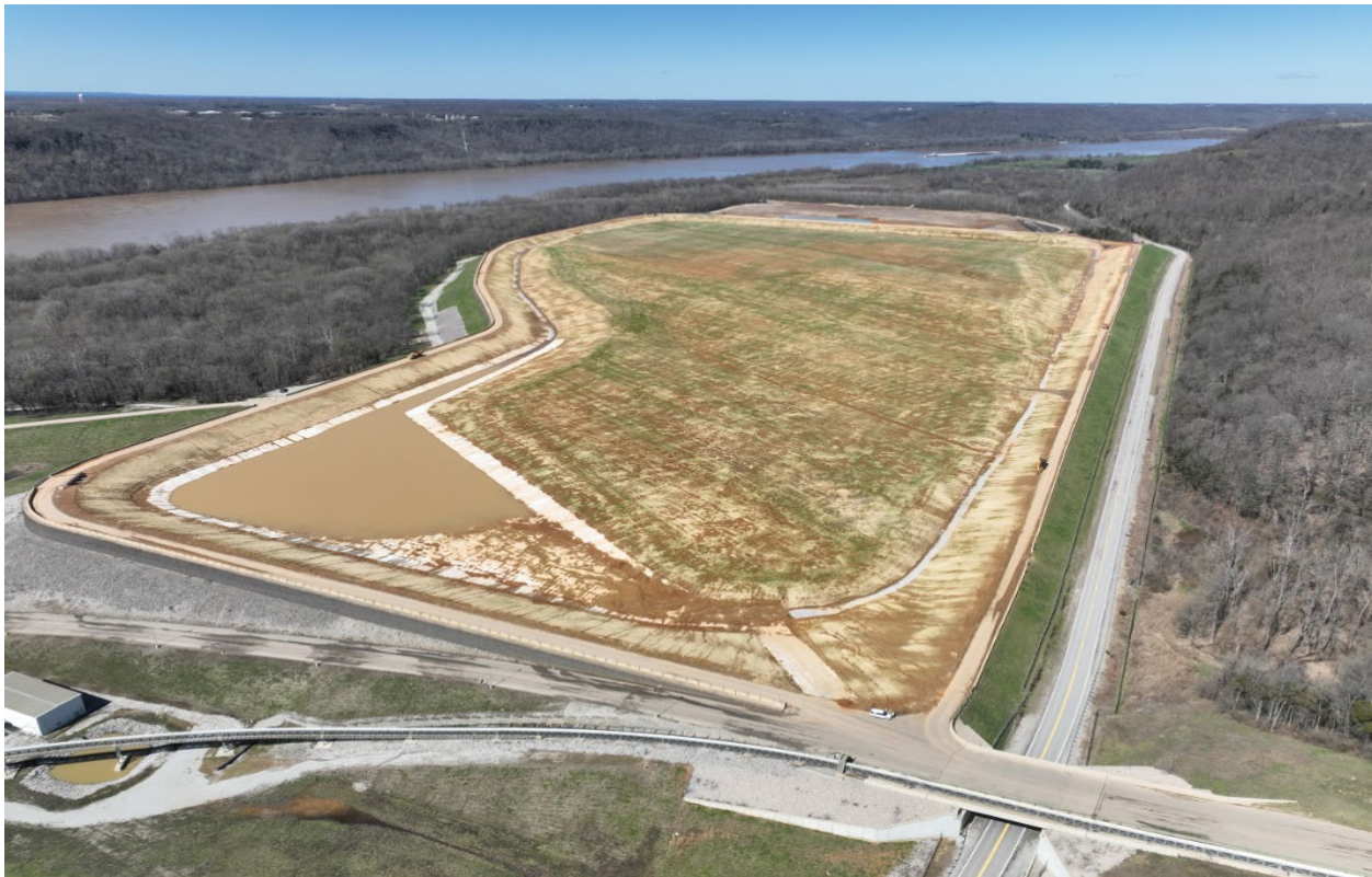
Trimble BAP – Looking Northeast – April 2026
