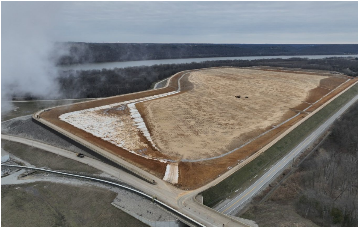
Trimble BAP – Looking Northeast – January 2026
