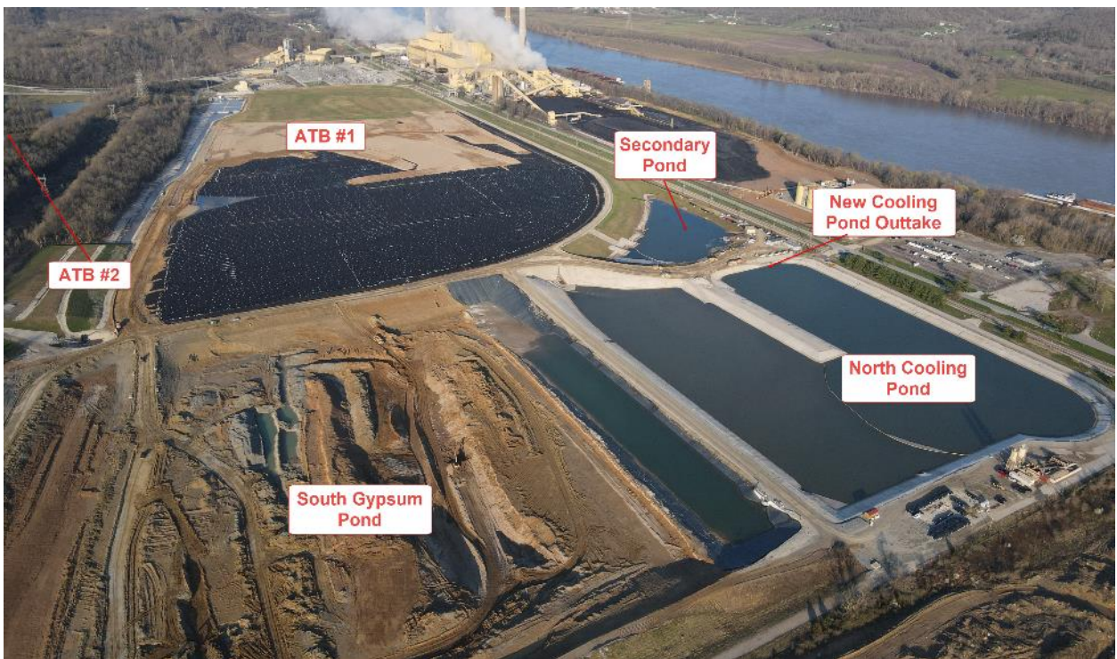
Ghent ATB #1 – Looking West – March 2021
