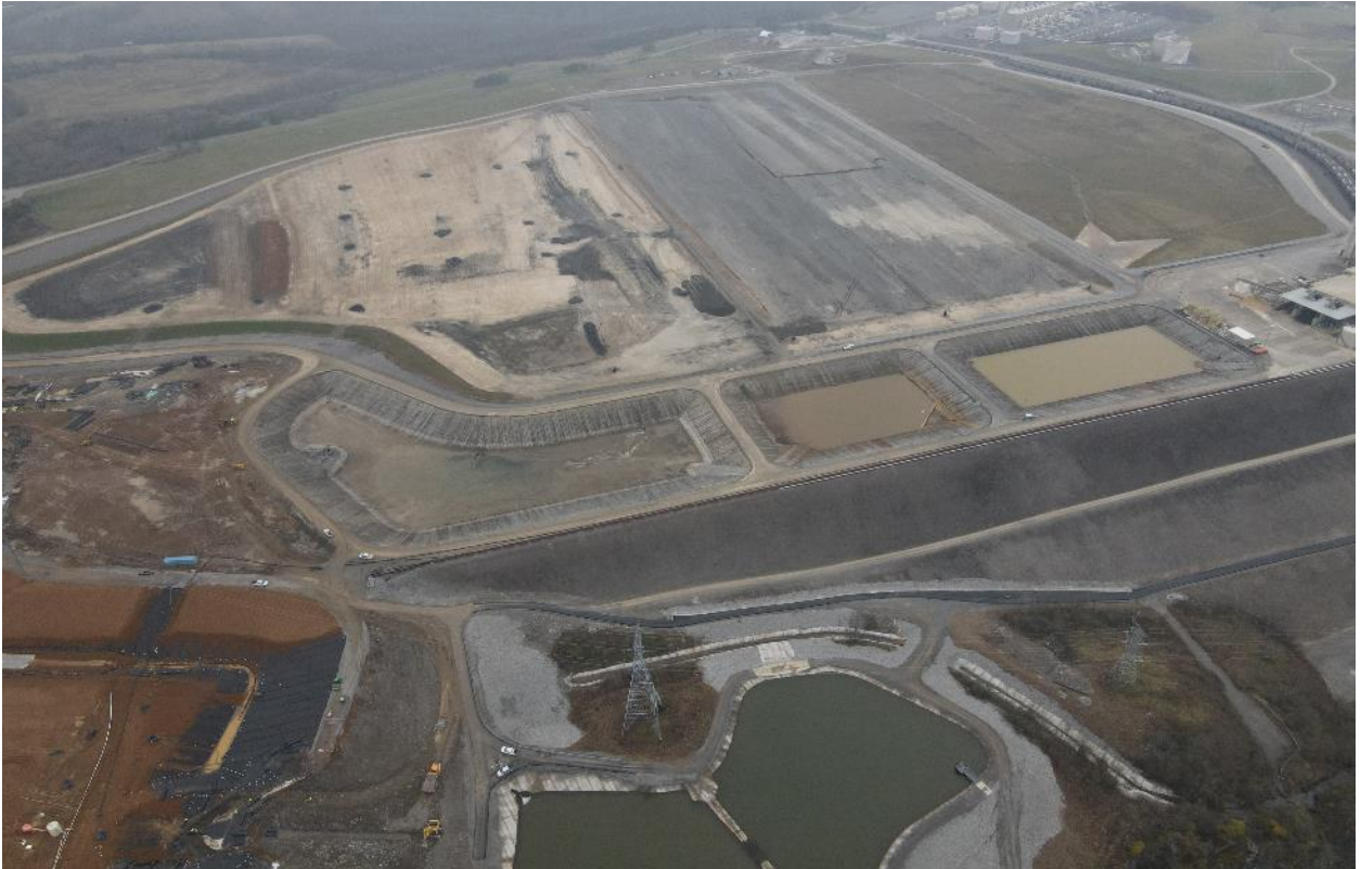
E.W. Brown Landfill Phase II and Closure – December 2020
