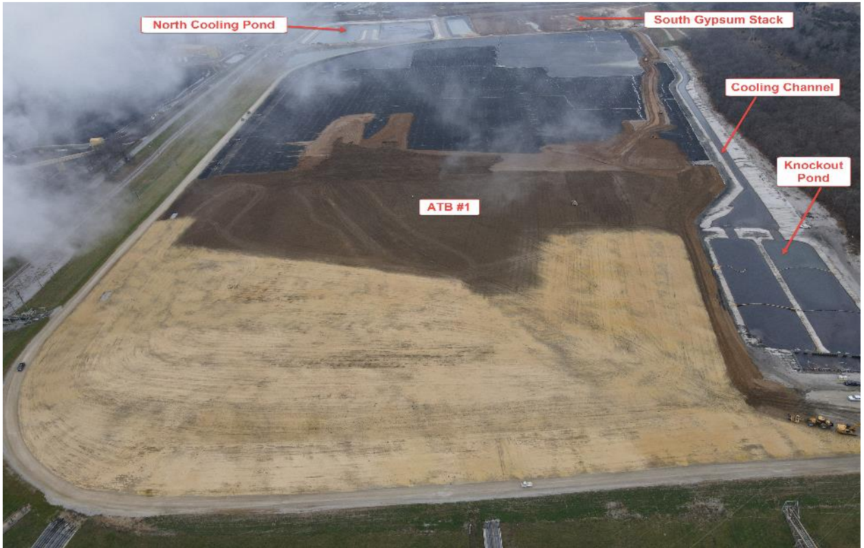
Ghent ATB #1 and Cooling Channel – Looking East – December 2020
