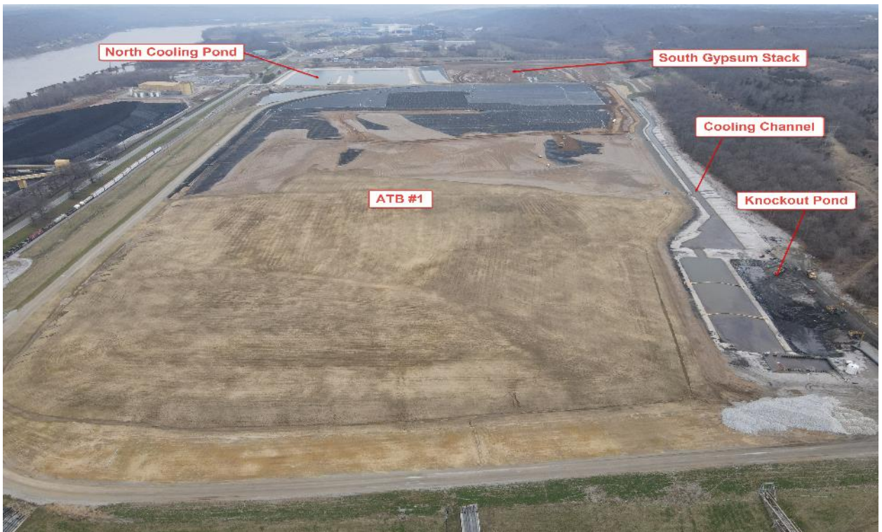
Ghent ATB #1 and Cooling Channel – Looking East – March 2021
