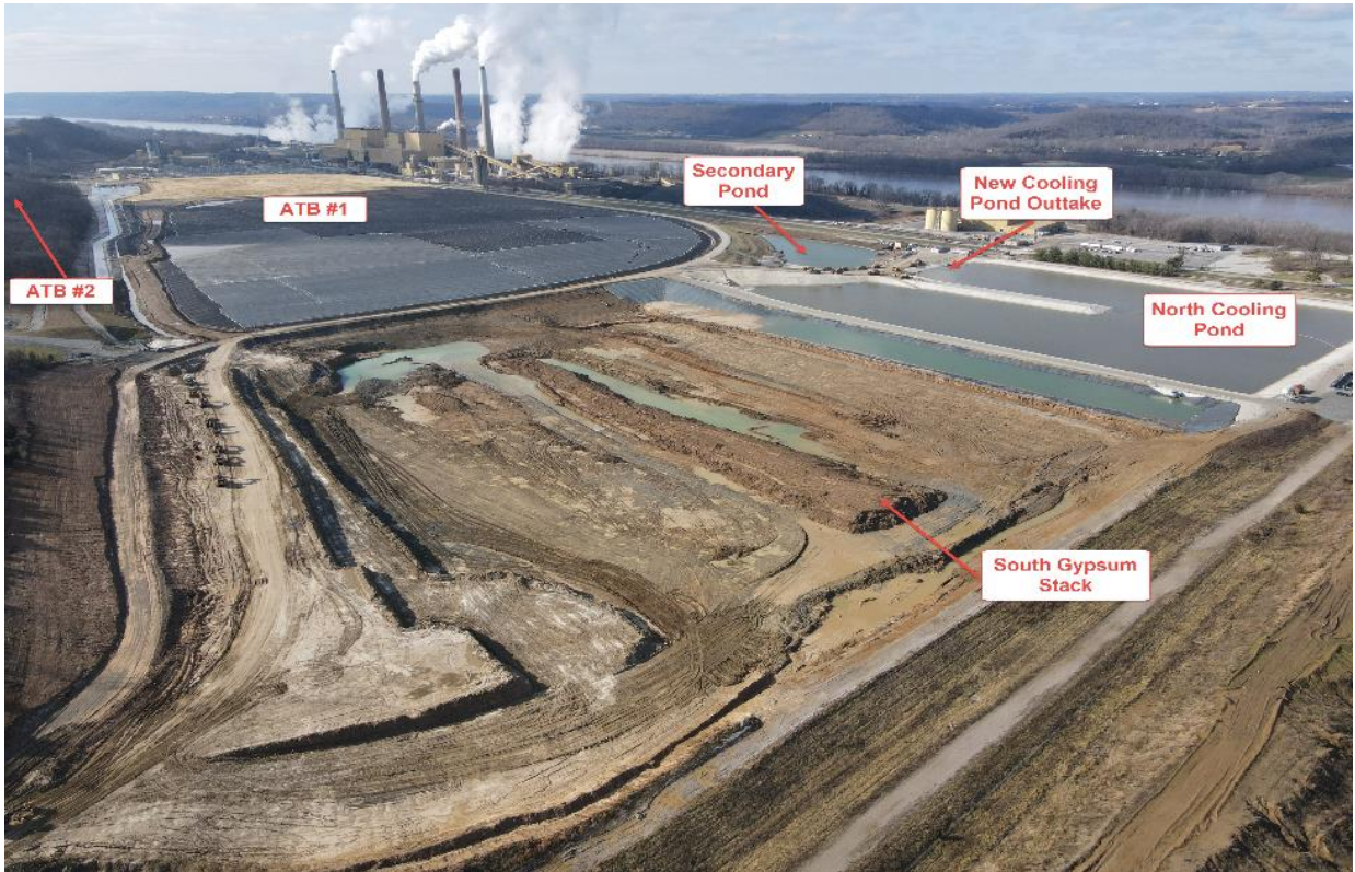
Ghent Gypsum Stack – Looking North – January 2021
