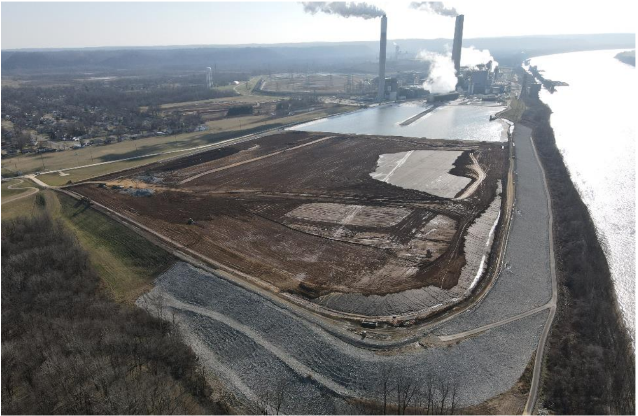
Mill Creek Main Ash Pond Closure – January 2021
