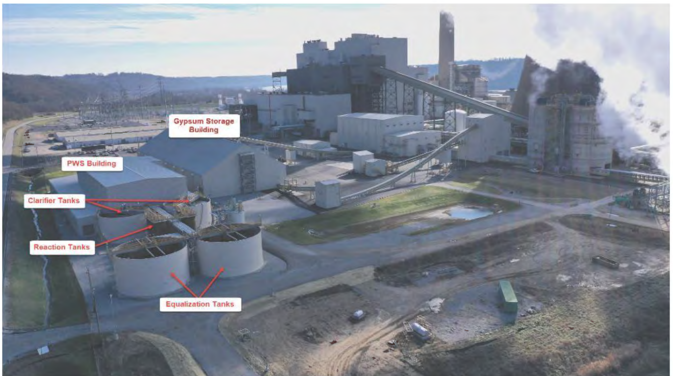
Trimble County PWS Facility – Site View Looking Southwest – December 2019 – No Change for March 2020
