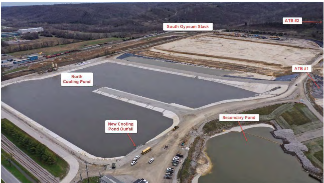
Ghent Gypsum Stack – Looking East – March 2020
