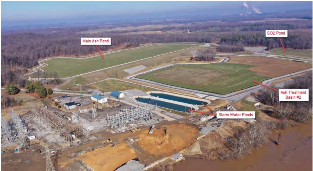
Green River CCR Impoundments – Site View – December 2019
