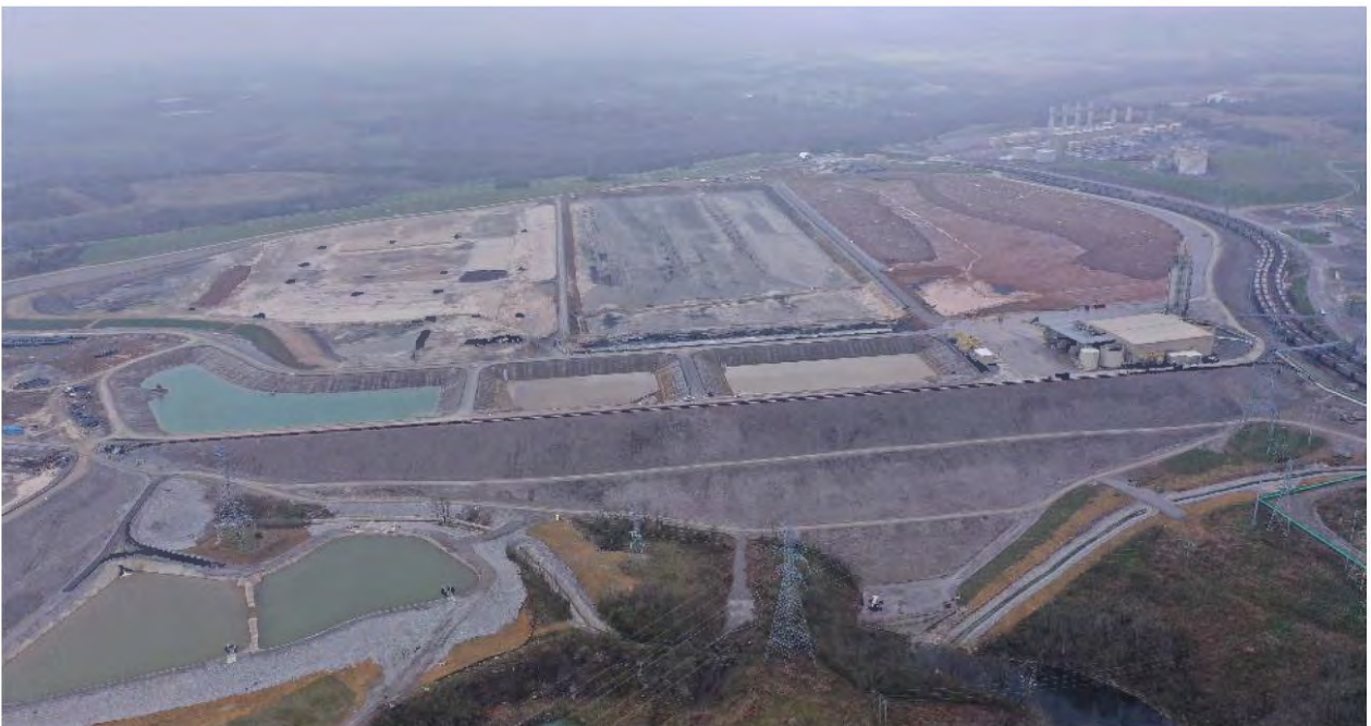
E.W. Brown Landfill Phase II and Closure – March 2020
