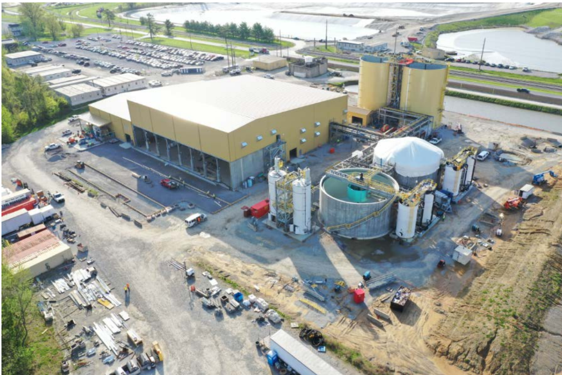
Ghent PWS Facility – Site View – April 2019
