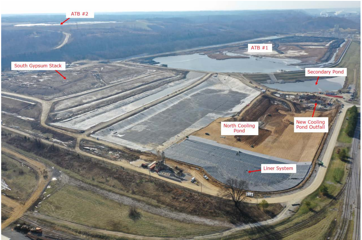
Ghent Gypsum Stack – Looking South – January 2019
