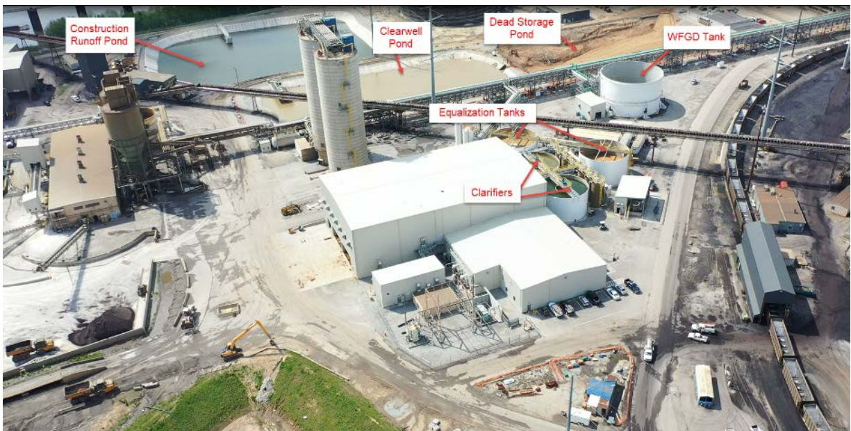
Mill Creek PWS Facility – Site View – April 2019
