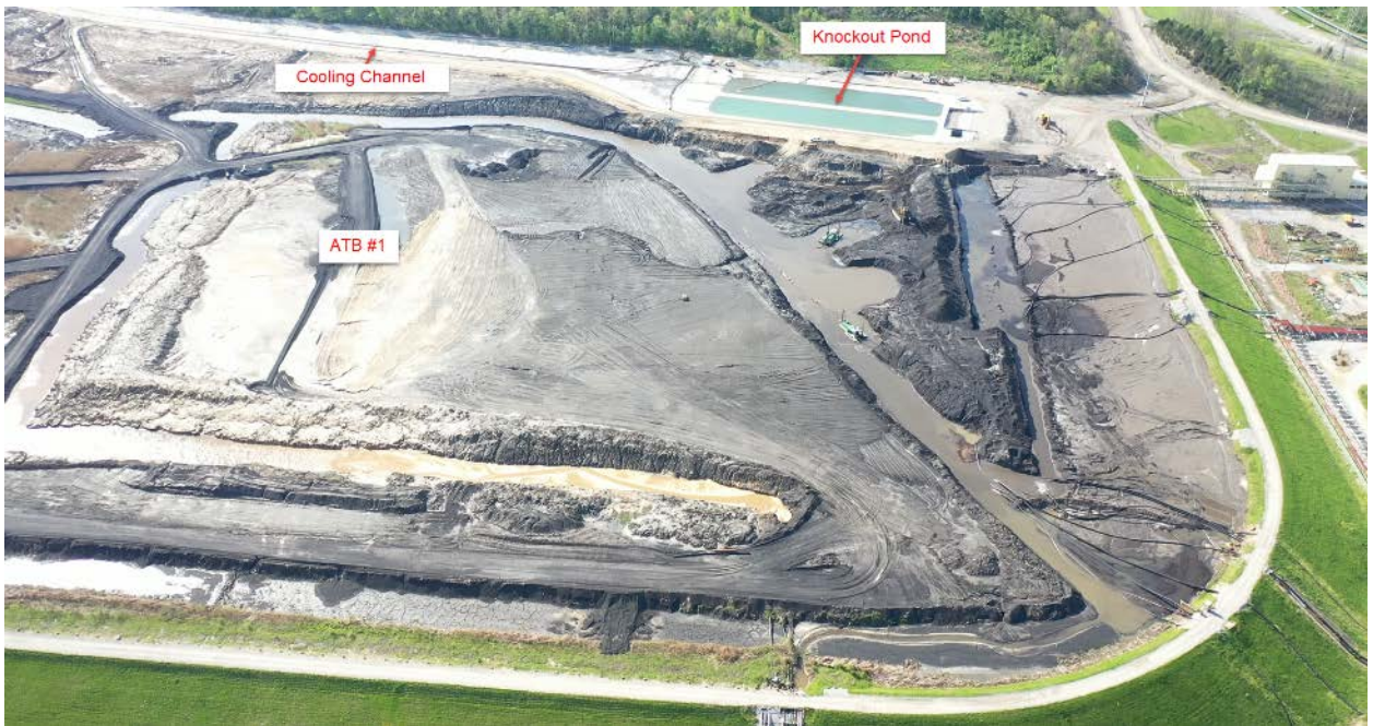
Ghent ATB #1 Cooling Channel – Looking North – April 2019
