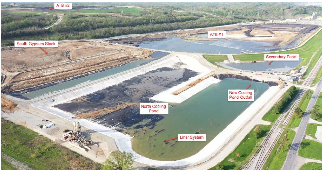
Ghent Gypsum Stack – Looking South – April 2019
