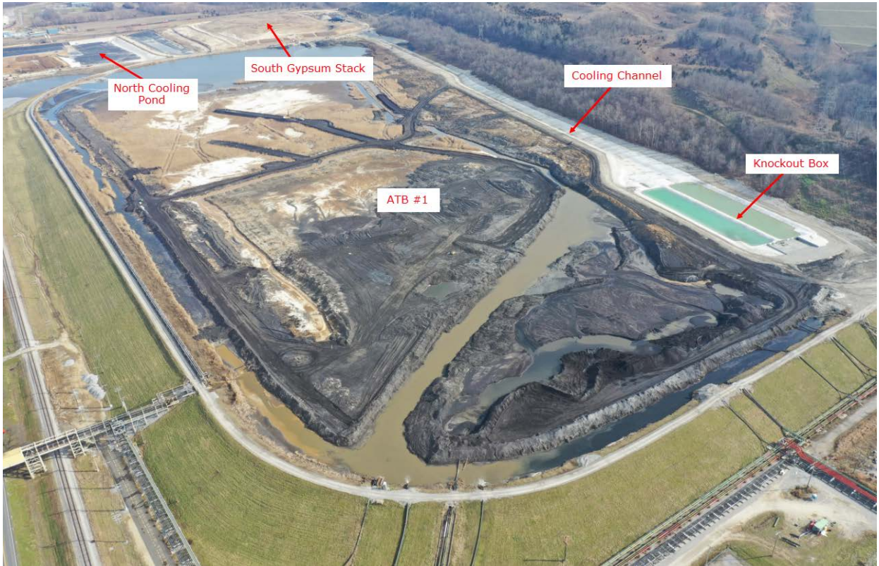
Ghent ATB #1 Cooling Channel – Looking West – January 2019
