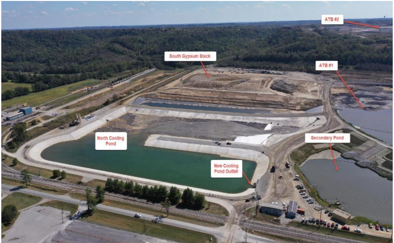
Ghent Gypsum Stack – Looking East – September 2019
