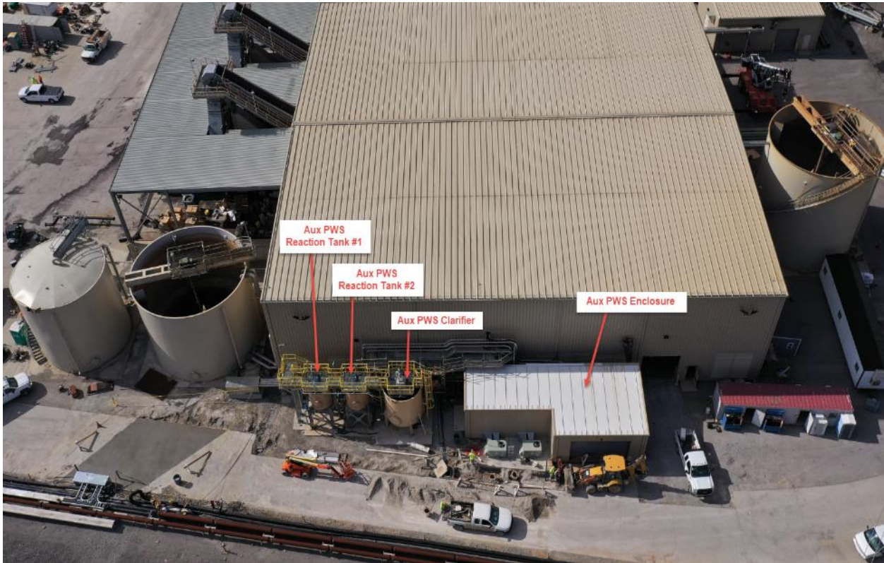
E.W. Brown PWS Treatment System – October 2019
