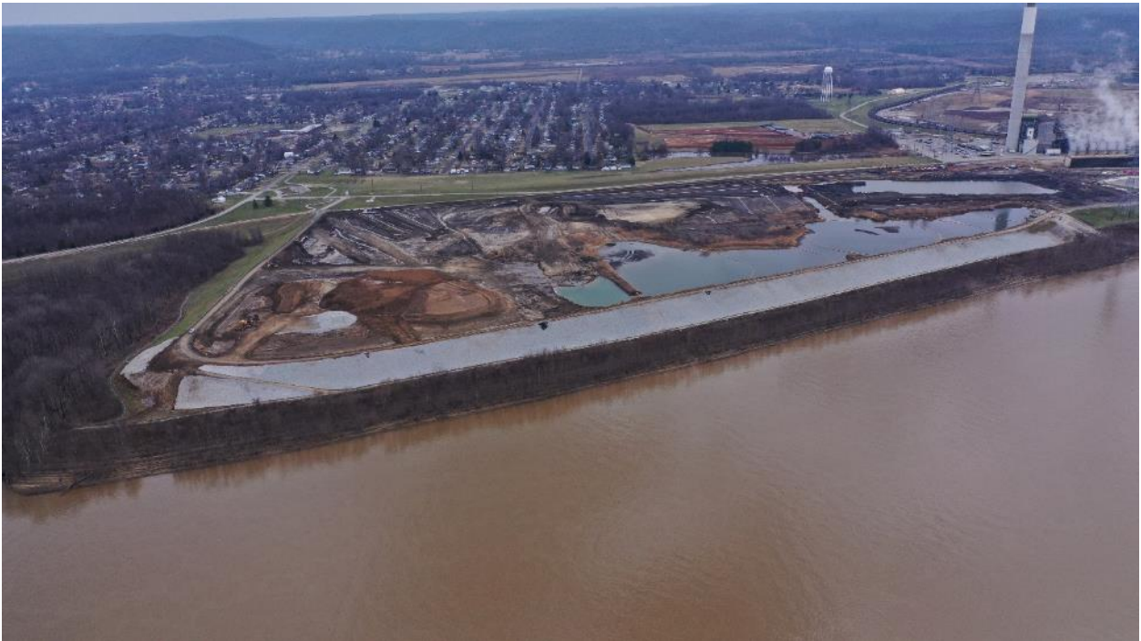
Mill Creek Main Ash Pond Closure – December 2019
