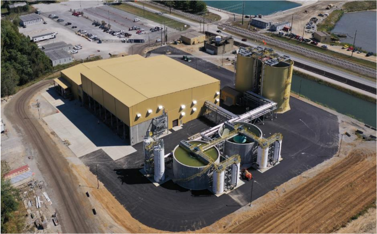
Ghent PWS Facility – Site View – October 2019 – No Change
