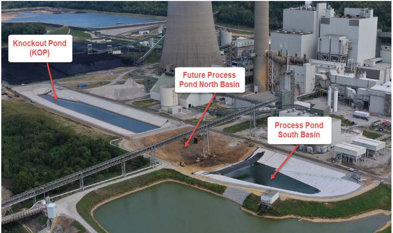
Trimble County Process Water Ponds – Looking Northeast – September 2019
