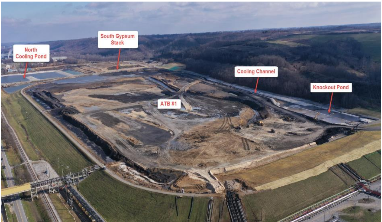
Ghent ATB #1 Cooling Channel – Looking East – December 2019
