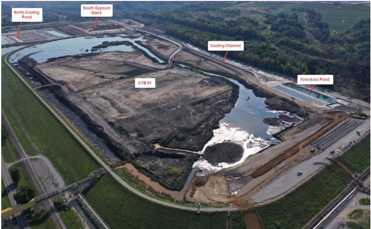
Ghent ATB #1 Cooling Channel – Looking East – September 2019
