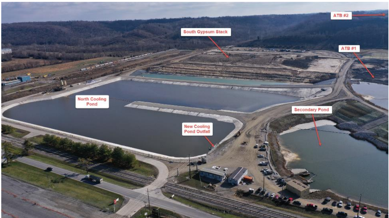
Ghent Gypsum Stack – Looking East – December 2019
