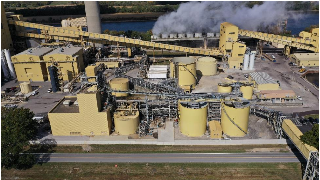
Ghent PWS Tank Farm – Site View – October 2019
