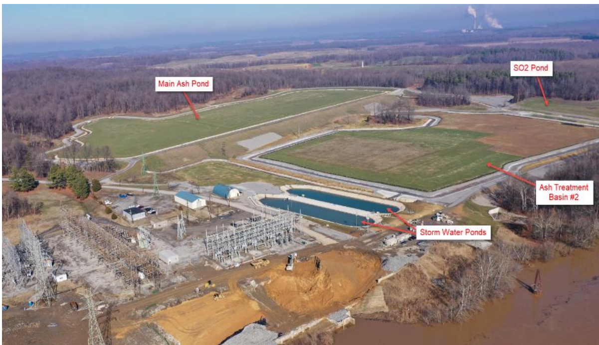
Green River CCR Impoundments – Site View – December 2019
