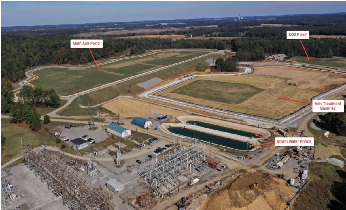
Green River CCR Impoundments – Site View – October 2019
