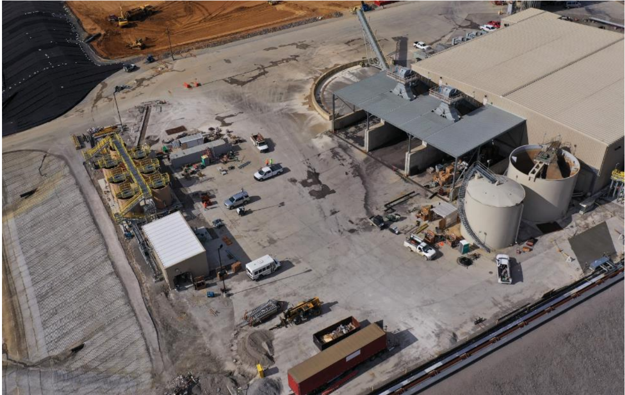
E.W. Brown Toe Drain and Coal Pile Runoff Treatment System – October 2019
