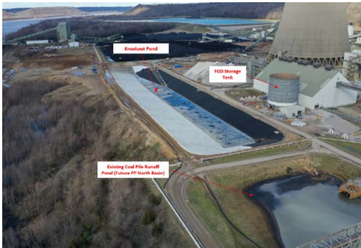
Trimble County PWP – Knockout Pond Overview – January 2019
