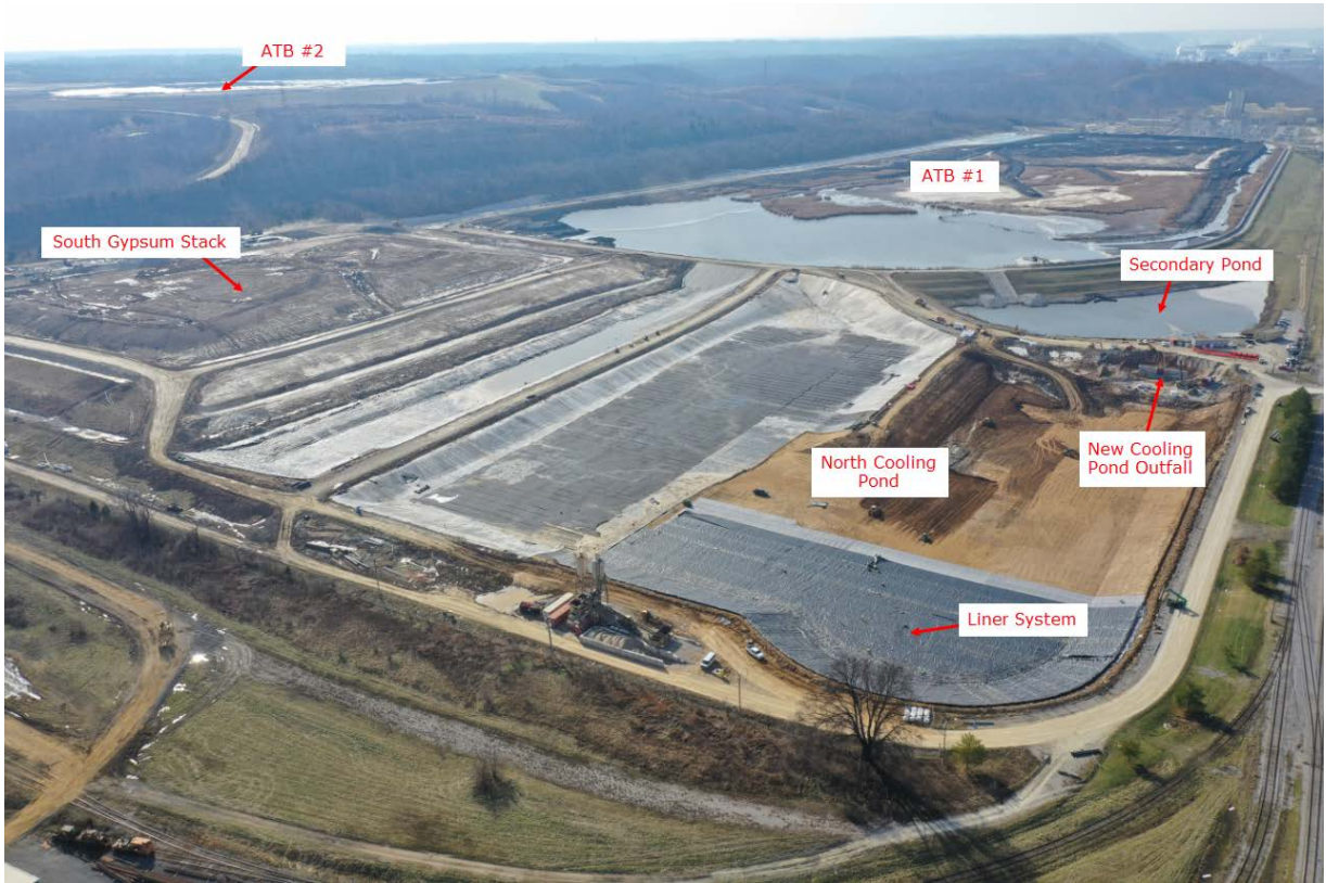
Ghent Gypsum Stack – Looking South – January 2019
