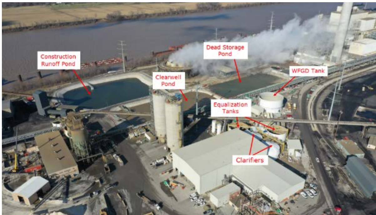
Mill Creek PWS Facility – Site View – January 2019
