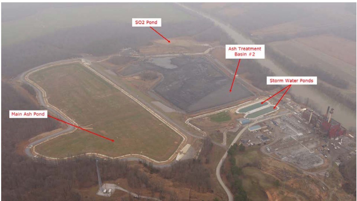
Green River CCR Impoundments – Site View – January 2019
