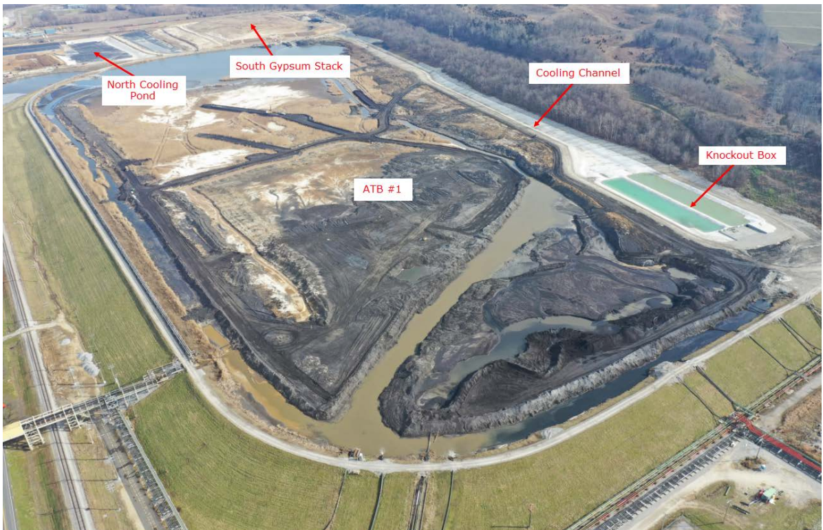
Ghent ATB #1 Cooling Channel – Looking West – January 2019
