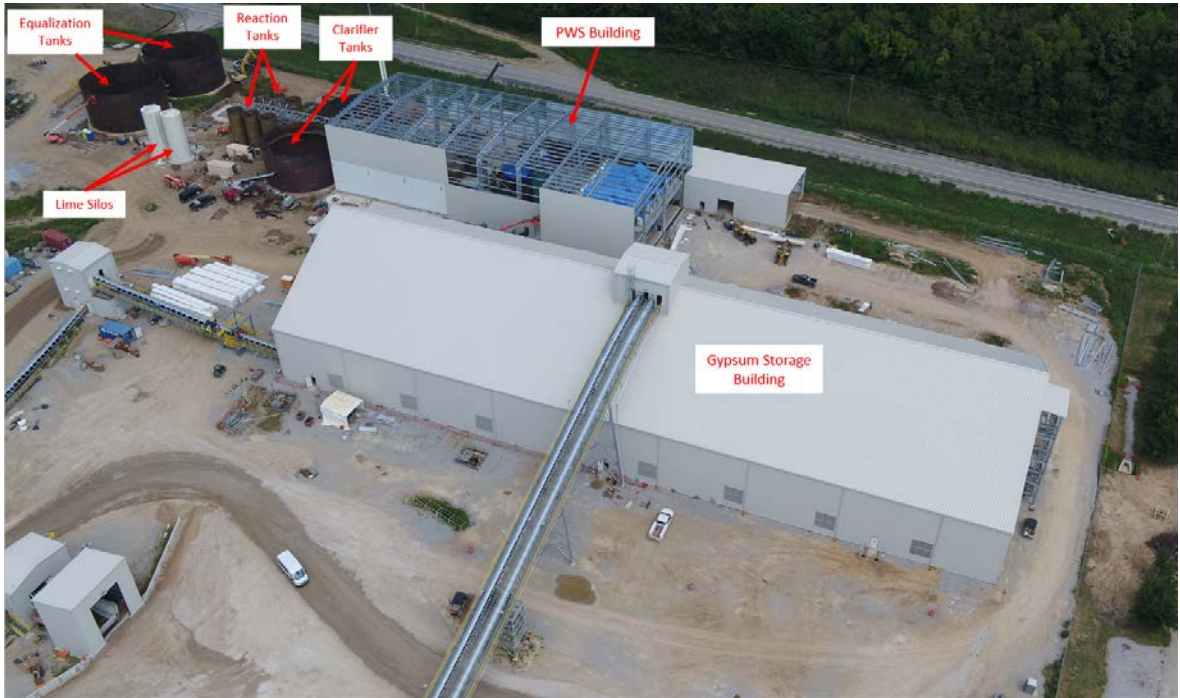
Trimble County PWS Facility – Site View Looking East – October 2018
