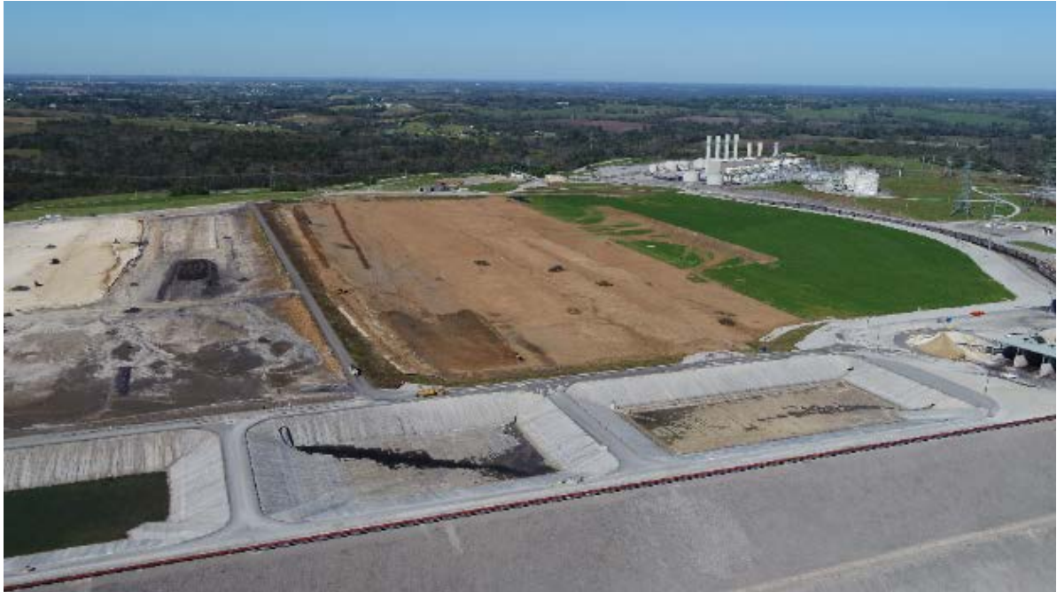
E.W. Brown Landfill Phase II and Closure – October 2018
