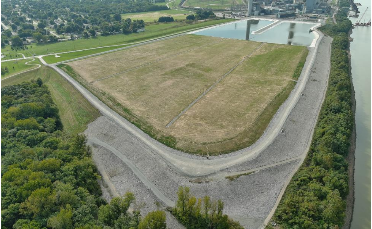
Mill Creek Main Ash Pond Closure – October 2021
