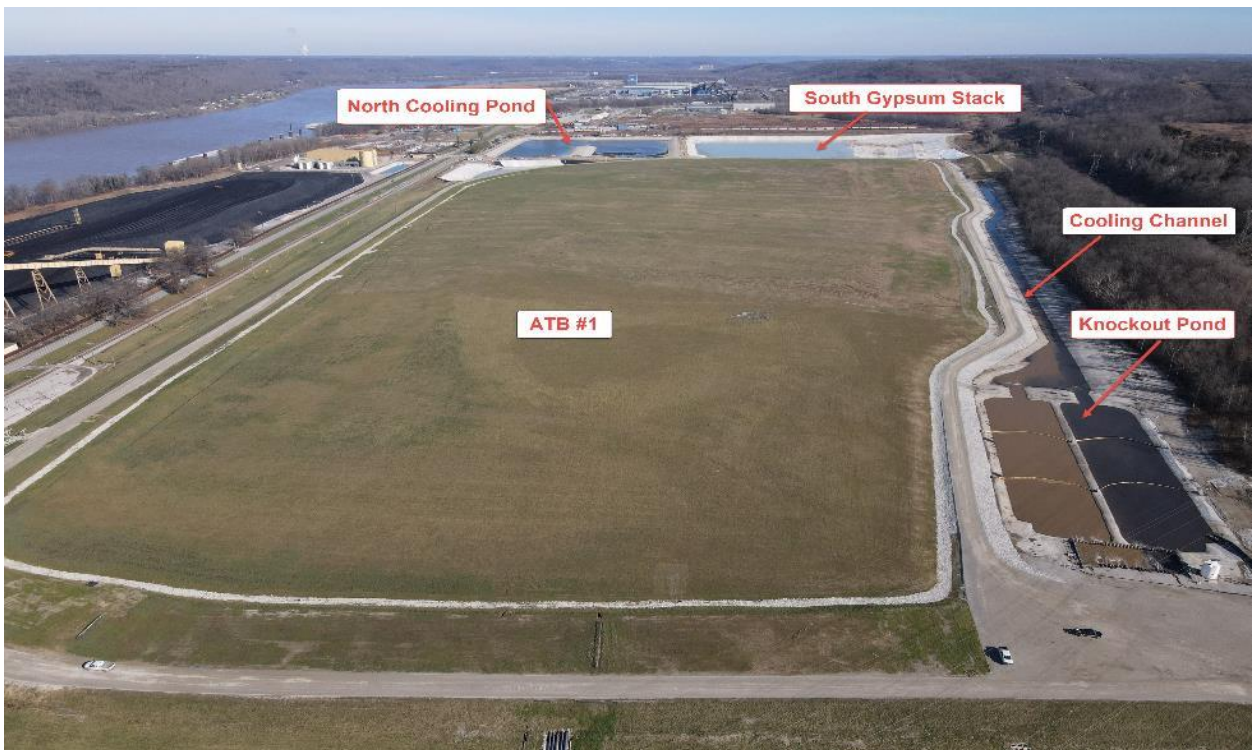
Gwent ATB #1 and Cooling Channel – Looking East – January 2022
