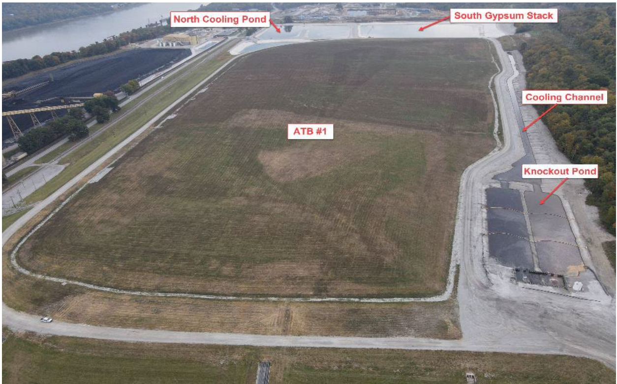
Phase II Ghent ATB #1 and Cooling Channel – Looking East – October 2022
