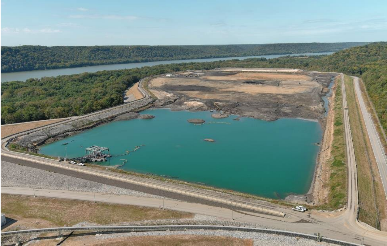
Trimble BAP – Looking North – October 2022
