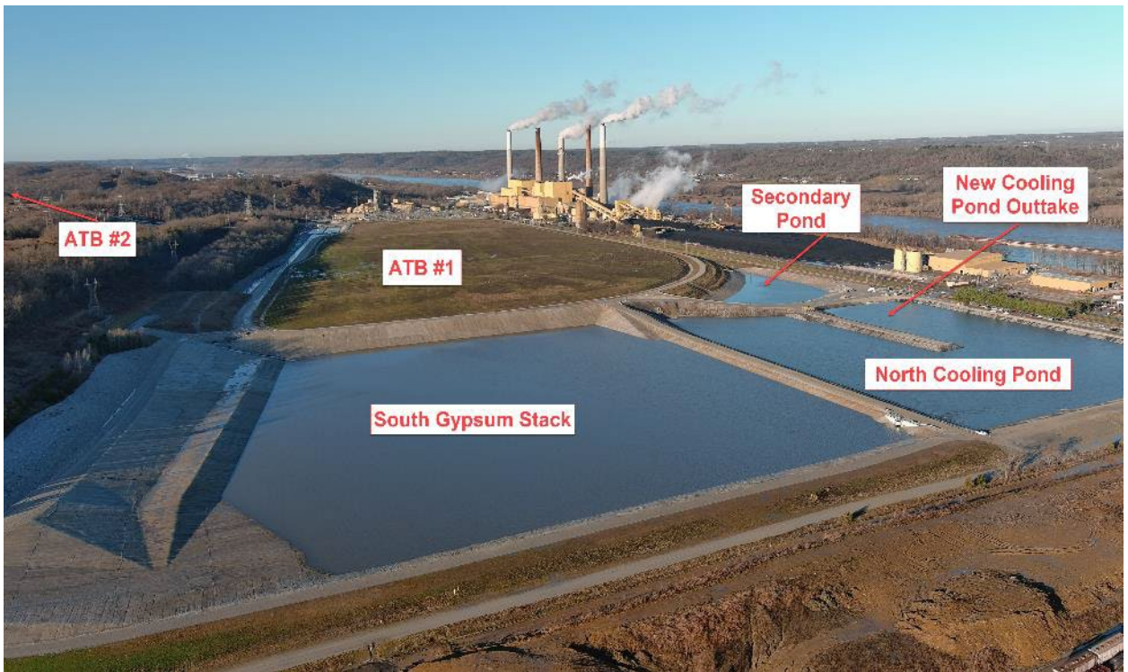
Phase II Ghent ATB #1 – Looking West – December 2022
