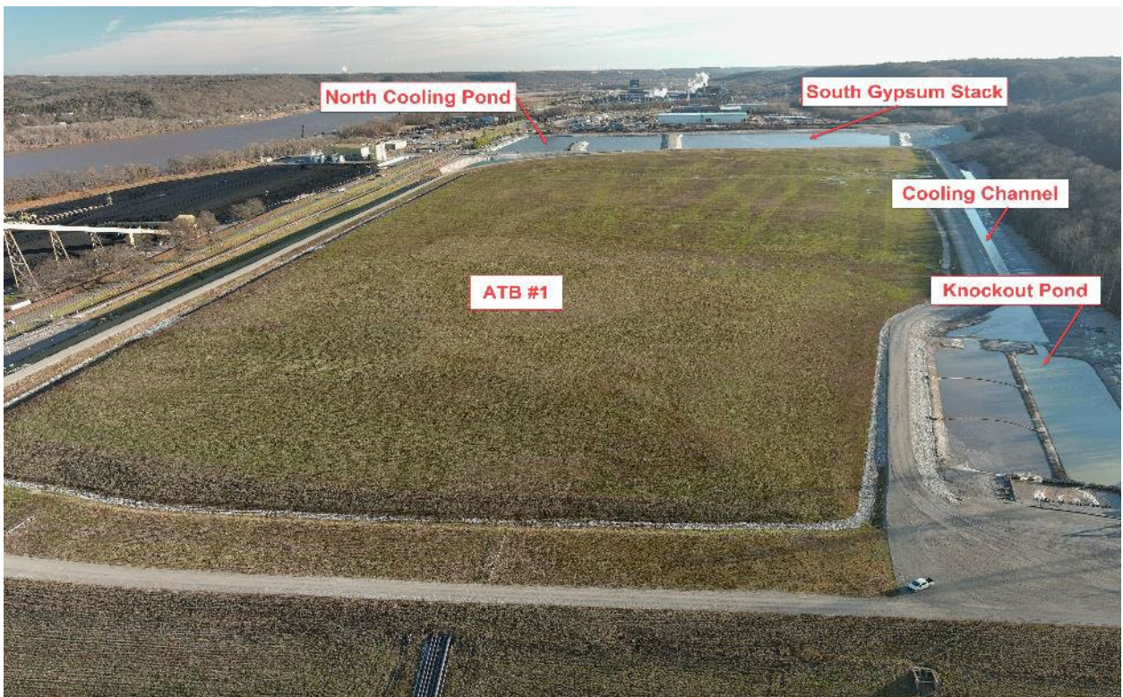
Phase II Ghent ATB #1 and Cooling Channel – Looking East – January 2023
