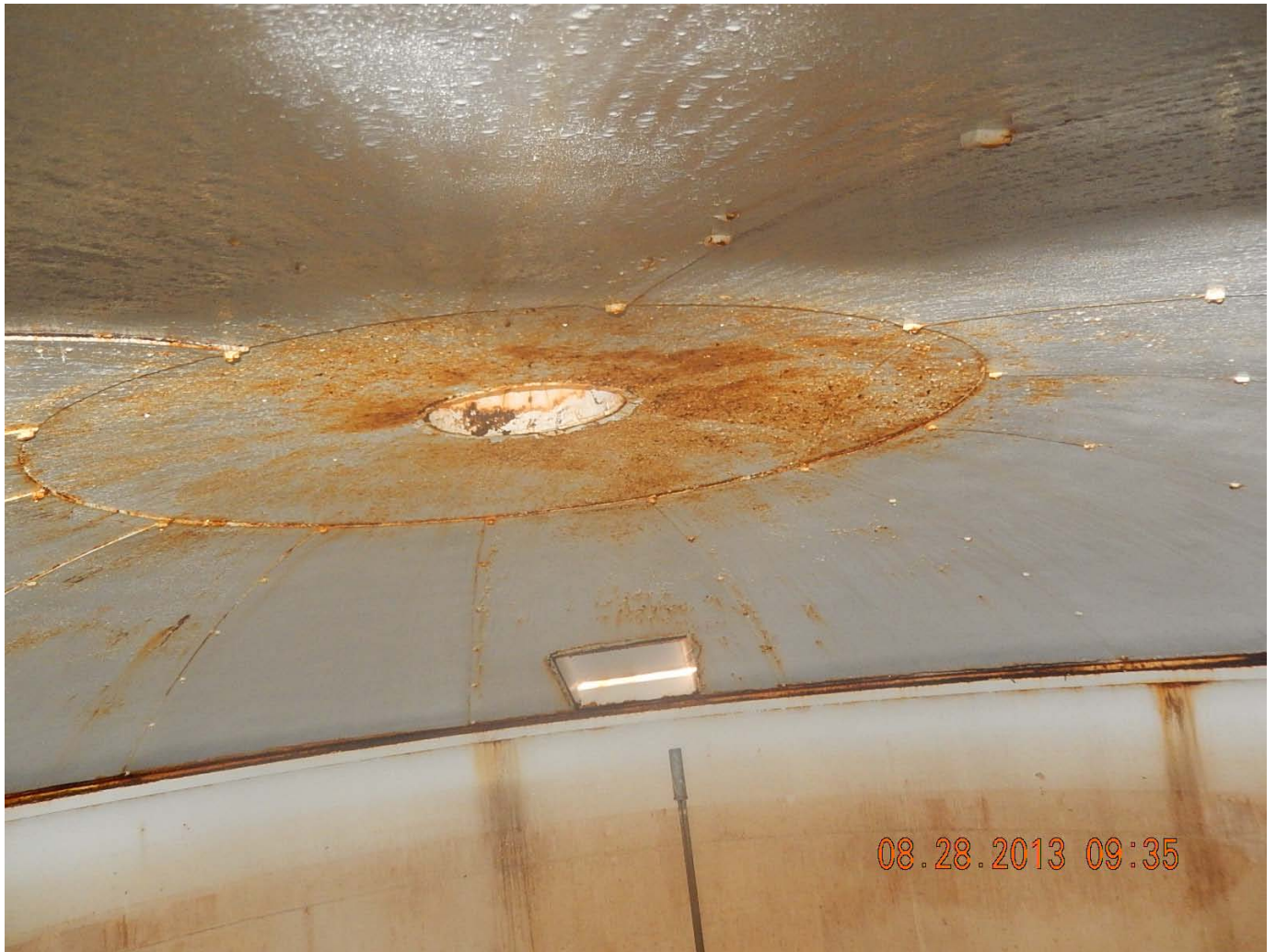
Interior roof and sidewall connection
