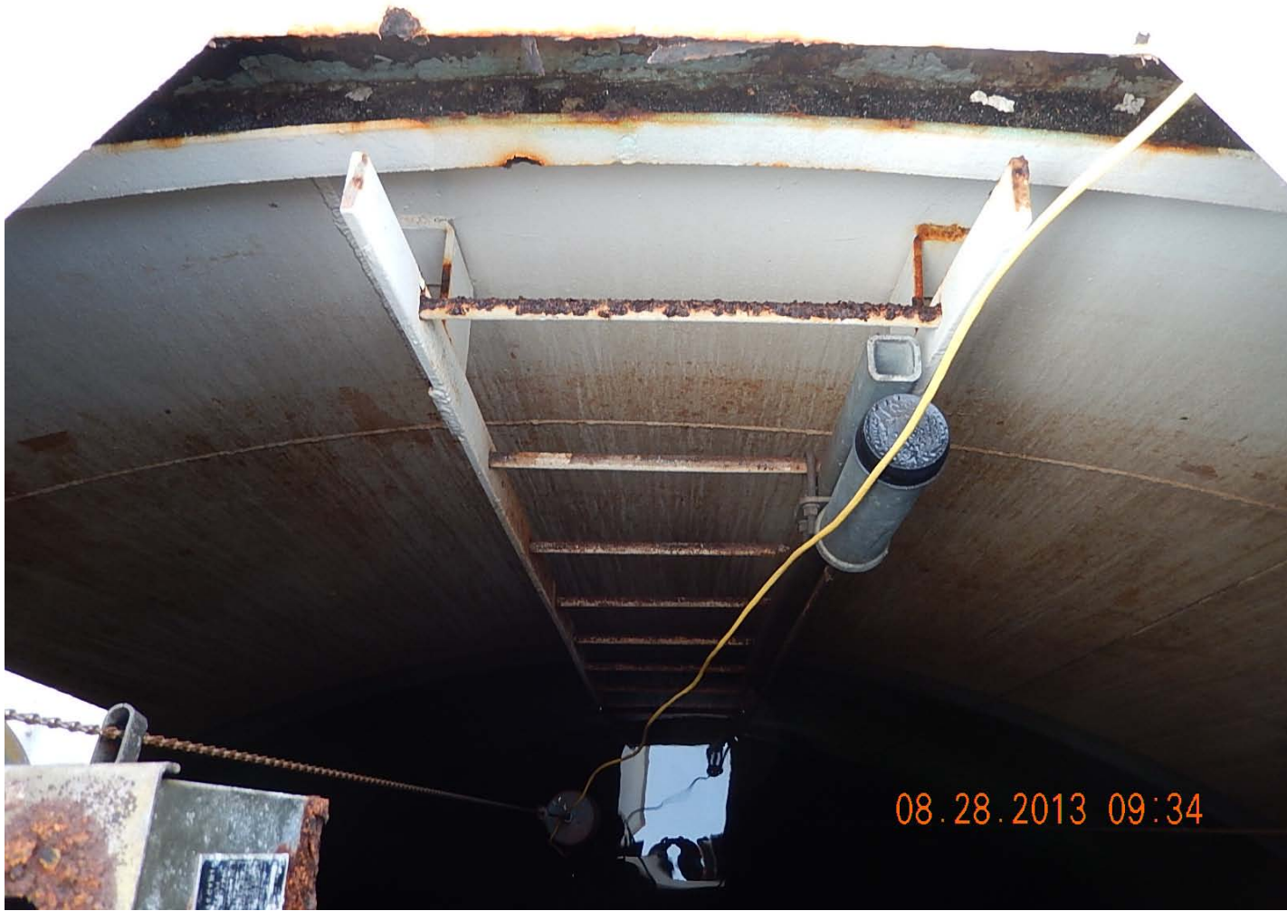
Interior ladder and steel above the high water line
