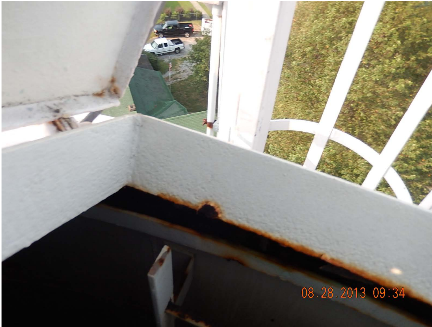
Roof manway, ladder cage
