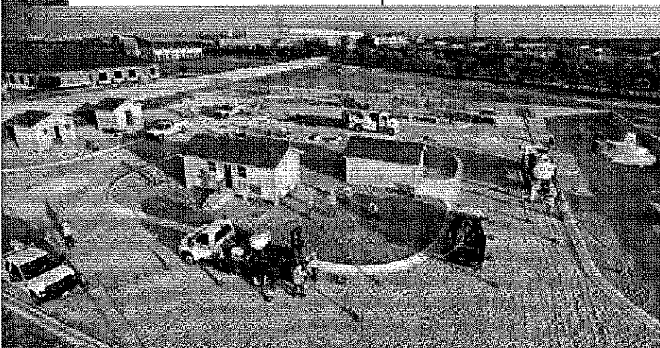
LEFT: Gas City at the company's Charles K. Vaughan Center simulates a mini-community with buildings, streets, pipelines and other utility infrastructure. Employees practice what they learn in the center's classrooms in hands-on situations. Called the finest facility of its kind, the center underscores Atmos Energy's commitment to advancing safe and reliable service.
