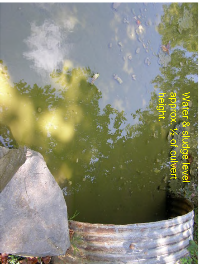
Note brownish grey sludge in waterway. Sludge level at the culvert was slightly lower than the water level.
