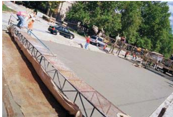
Figure 3-5: Fly ash concrete finishing
