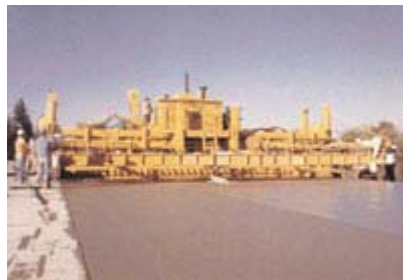
Figure 3-1: Fly ash improves workability for pavement concrete.
