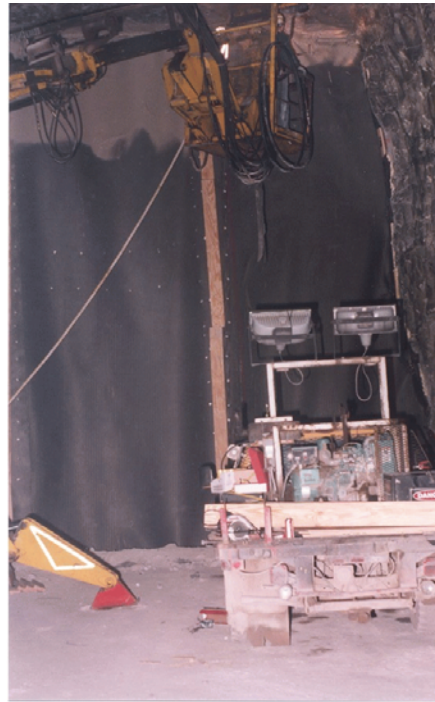
Figure 8. Fabric-grid material sprayed with cementitious material.
