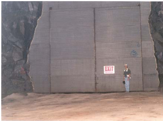
Figure 7. Stopping made for corrugated steel panels reinforced with a steel frame.
