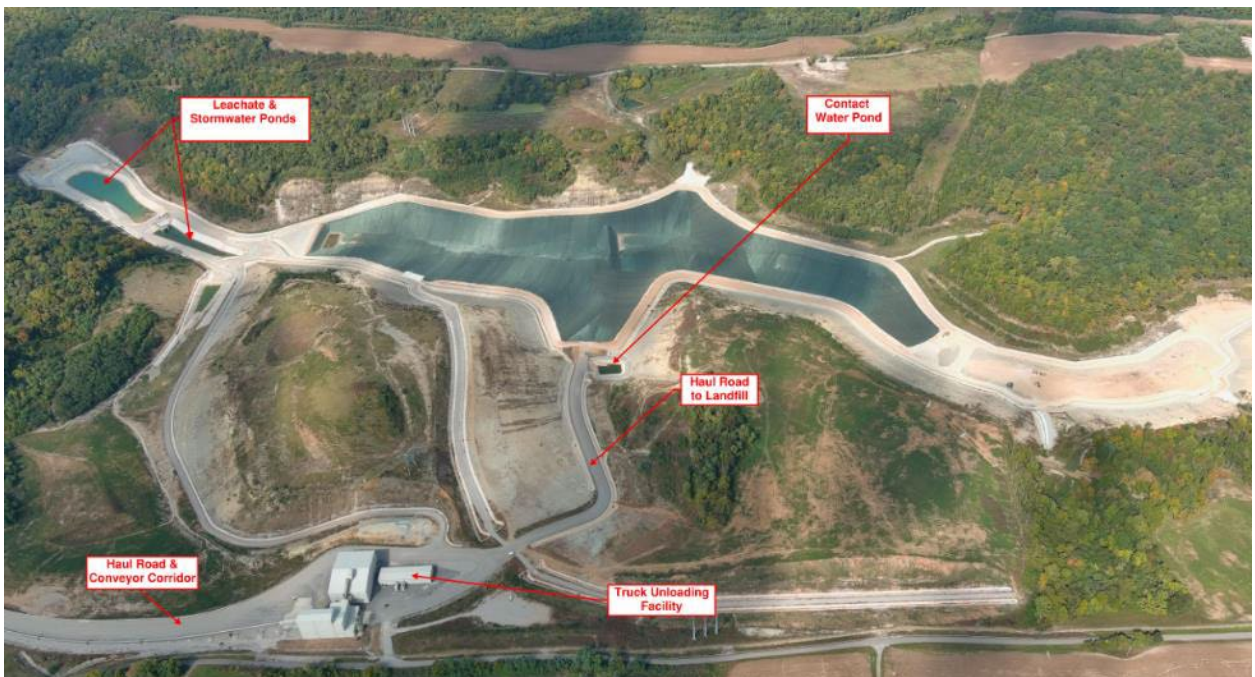
CCR Landfill Overview – View Looking North October 2022
