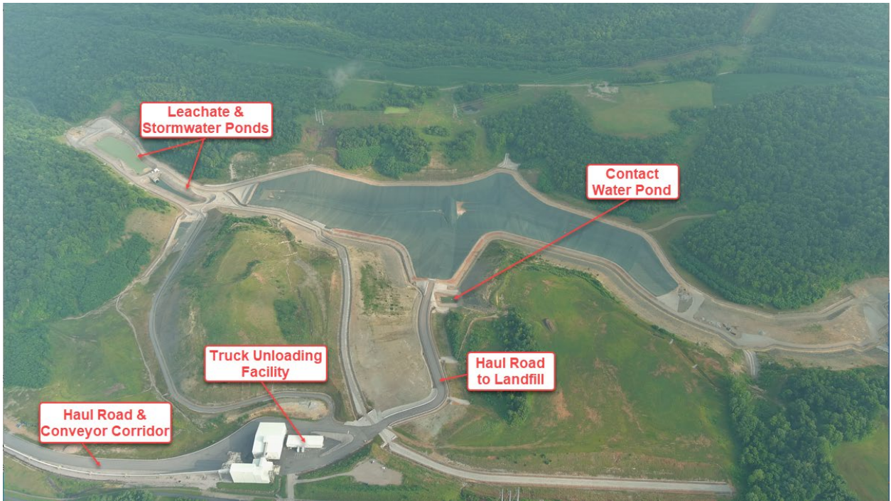
CCR Landfill Overview – View Looking North – June 2023 – No Changes
