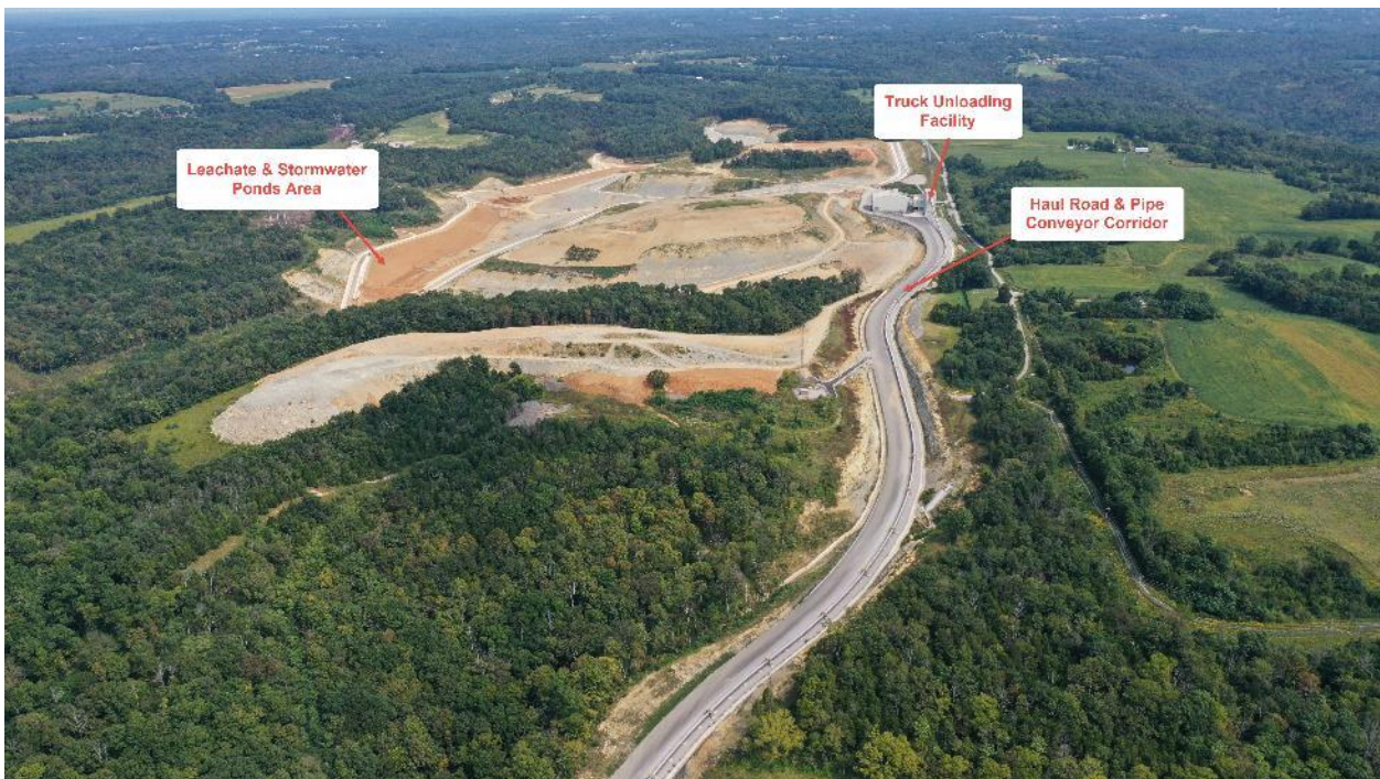
CCR Landfill Overview – View Looking Toward Station (Looking East) – September 2020
