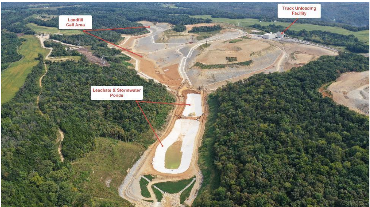
CCR Landfill Overview – View Looking South West – September 2020
