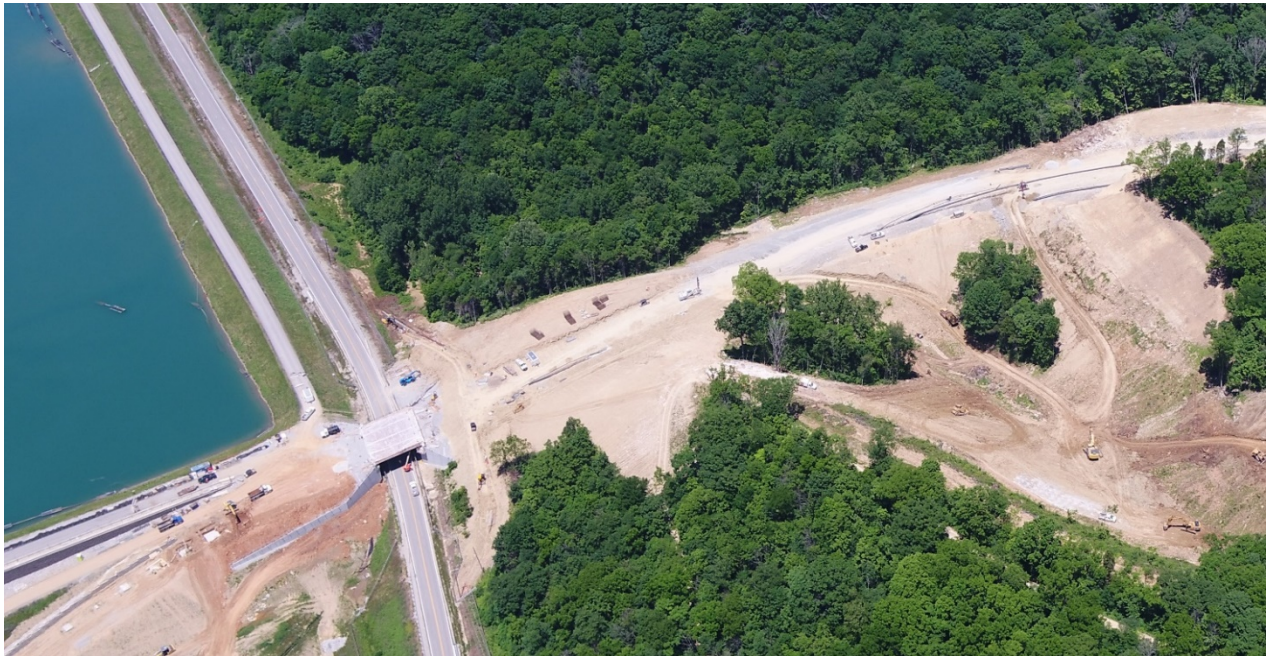
CCR Transport Corridor – View of Bridge over KY 1838 to Landfill (Looking North) – June 2018
