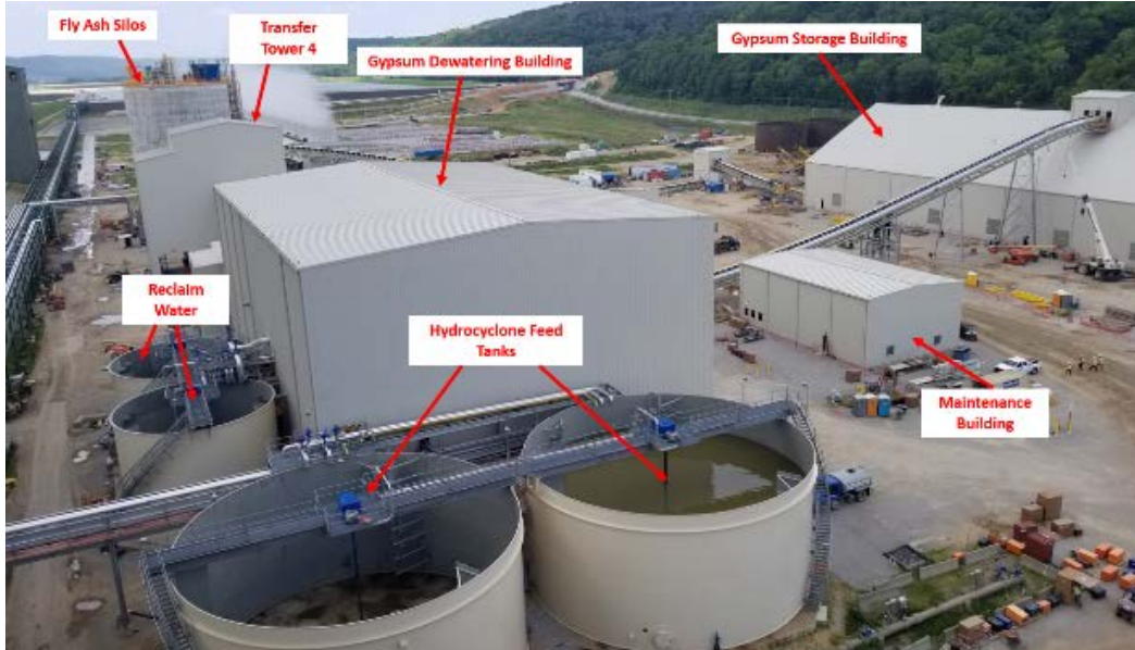
CCRT Project Area Looking North – June 2018
