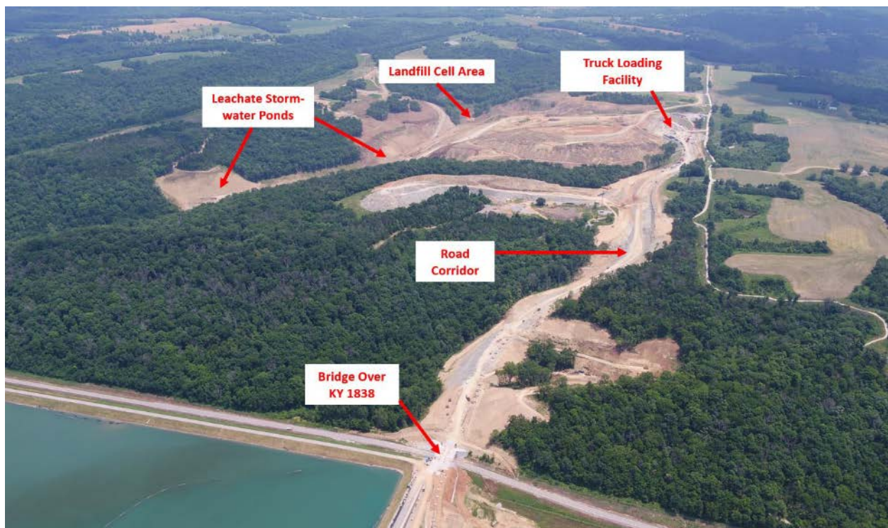
CCR Landfill Overview – View from Station (Looking East) – June 2018
