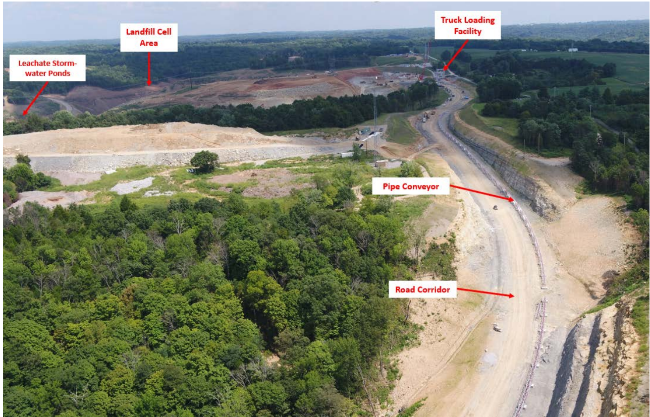
CCR Landfill Overview – View from Station (Looking East) – End of August 2018
