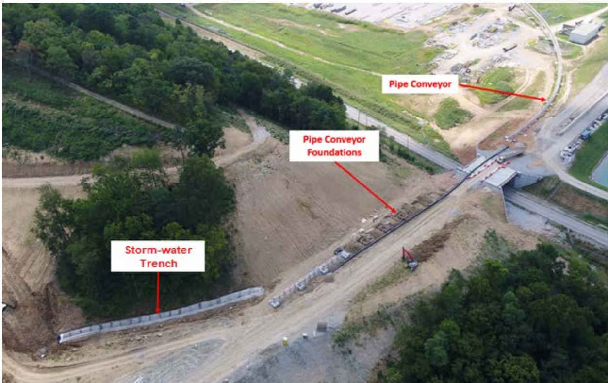
CCRT Transport Corridor – View of Bridge Over KY 1838 to Landfill (Looking West) – End of August 2018
