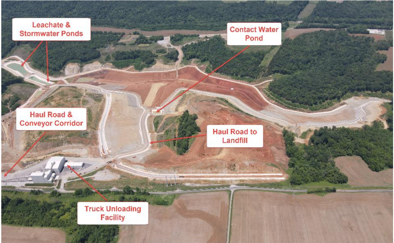
CCR Landfill Overview – View Looking North June 2021
