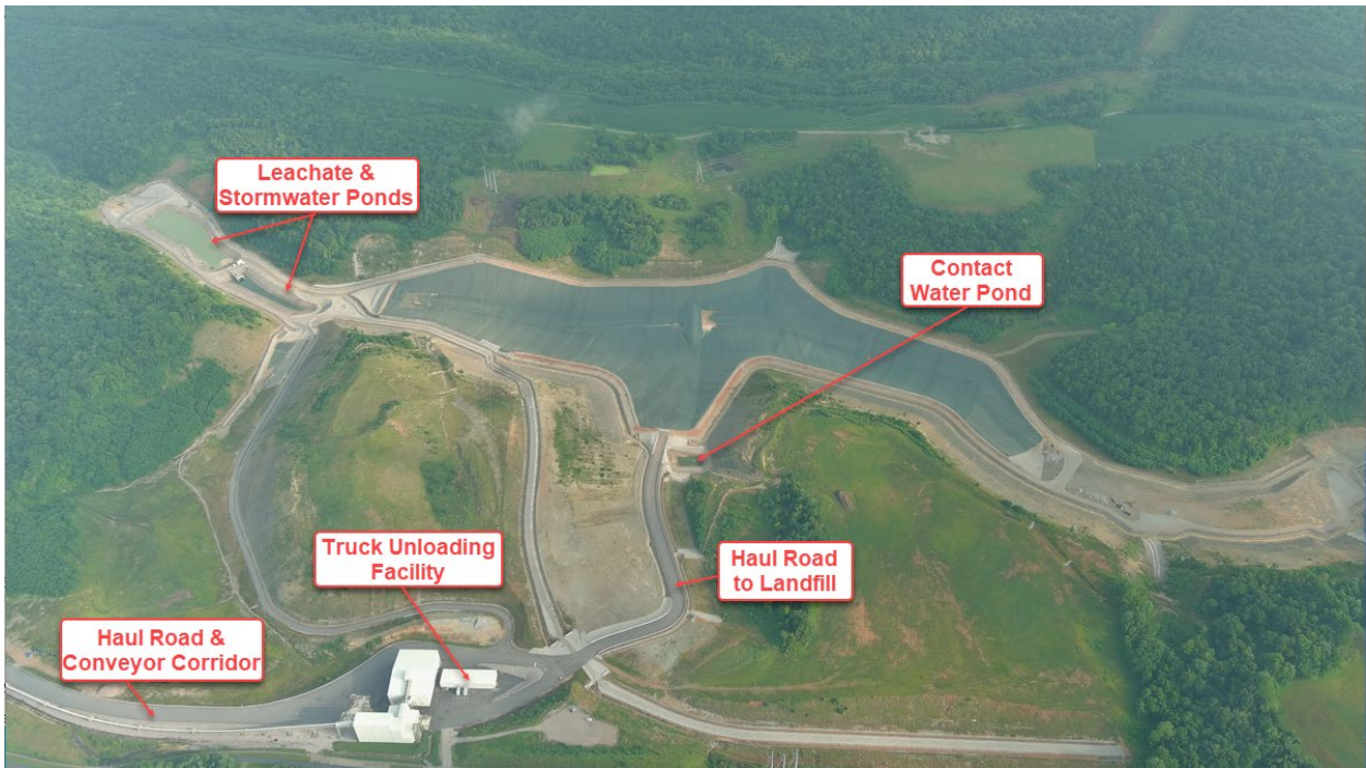
CCR Landfill Overview – View Looking North – June 2023
