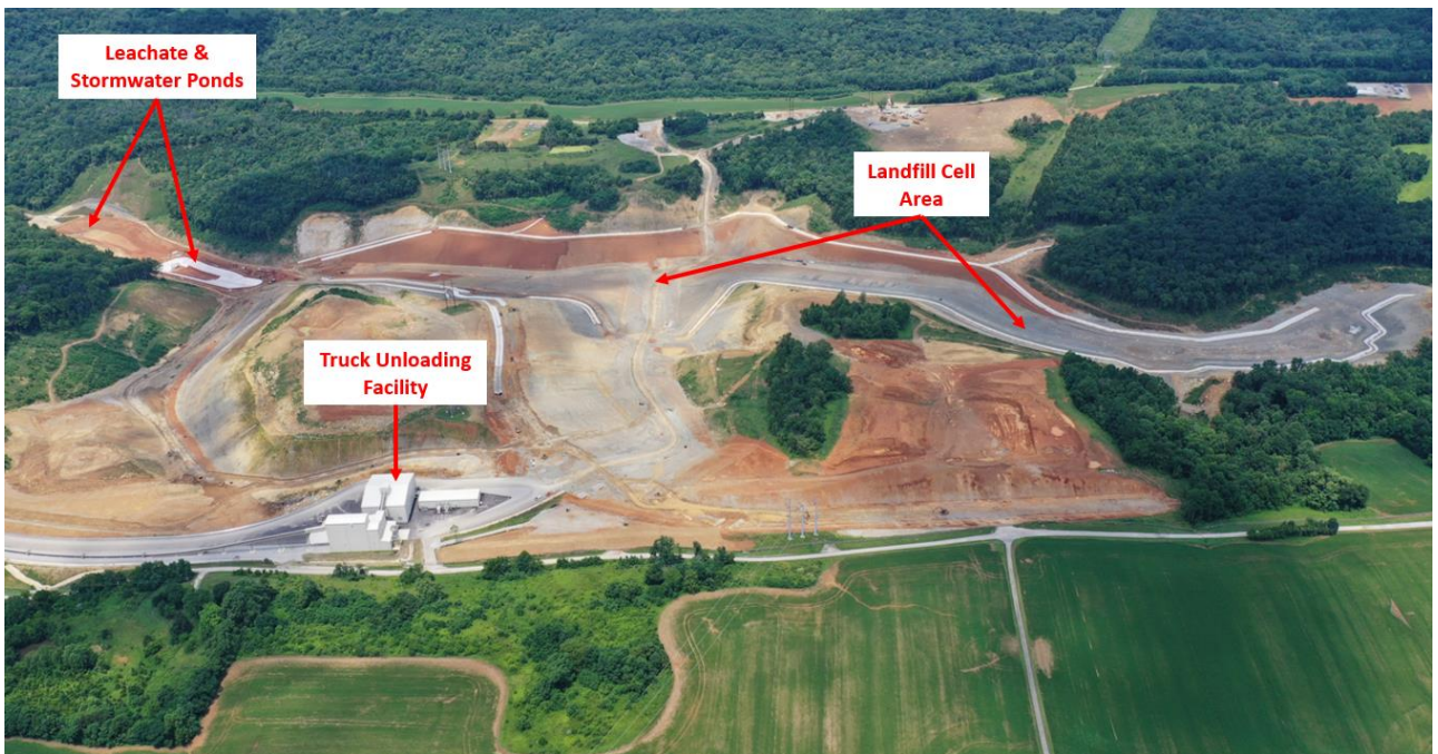
CCR Landfill Overview – View Looking North East – June 2020
