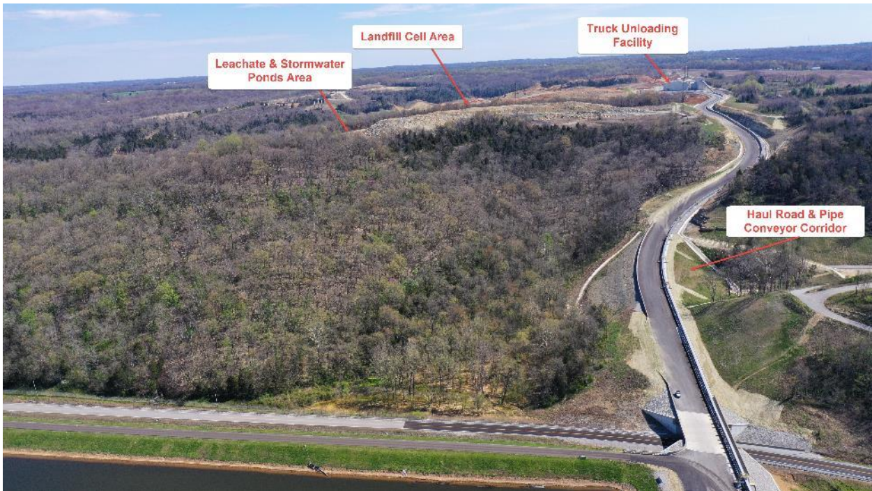
CCR Landfill Overview – View from Station (Looking East) – March 2020
