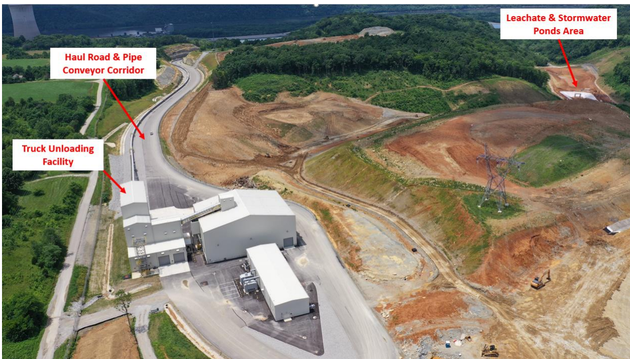
CCR Landfill Overview – View Looking Toward Station (Looking West) – June 2020
