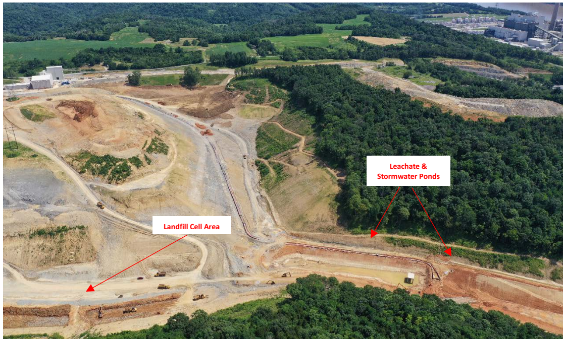
CCR Landfill Overview – View toward Station (Looking South West) – June 2019
