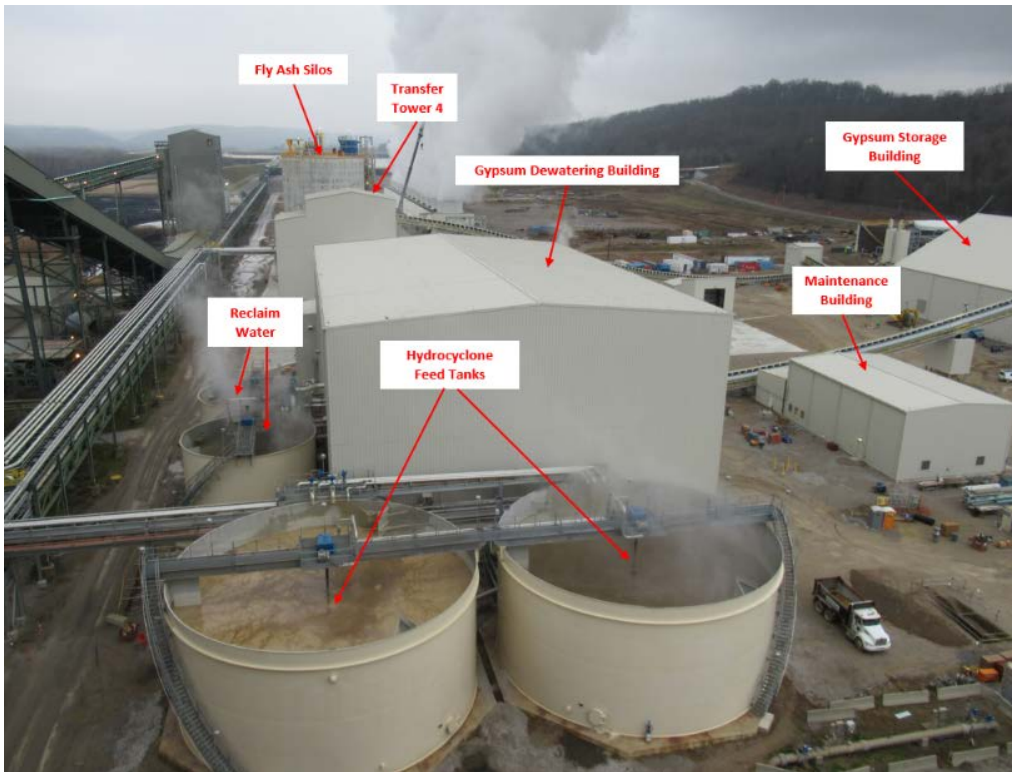
CCRT Project Area Looking North – December 2018
