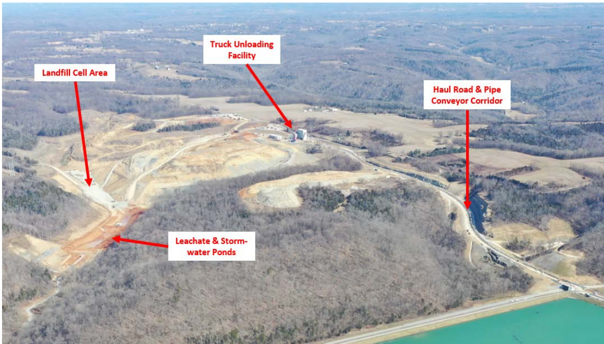
CCR Landfill Overview – View from Station (Looking East) – March 2019
