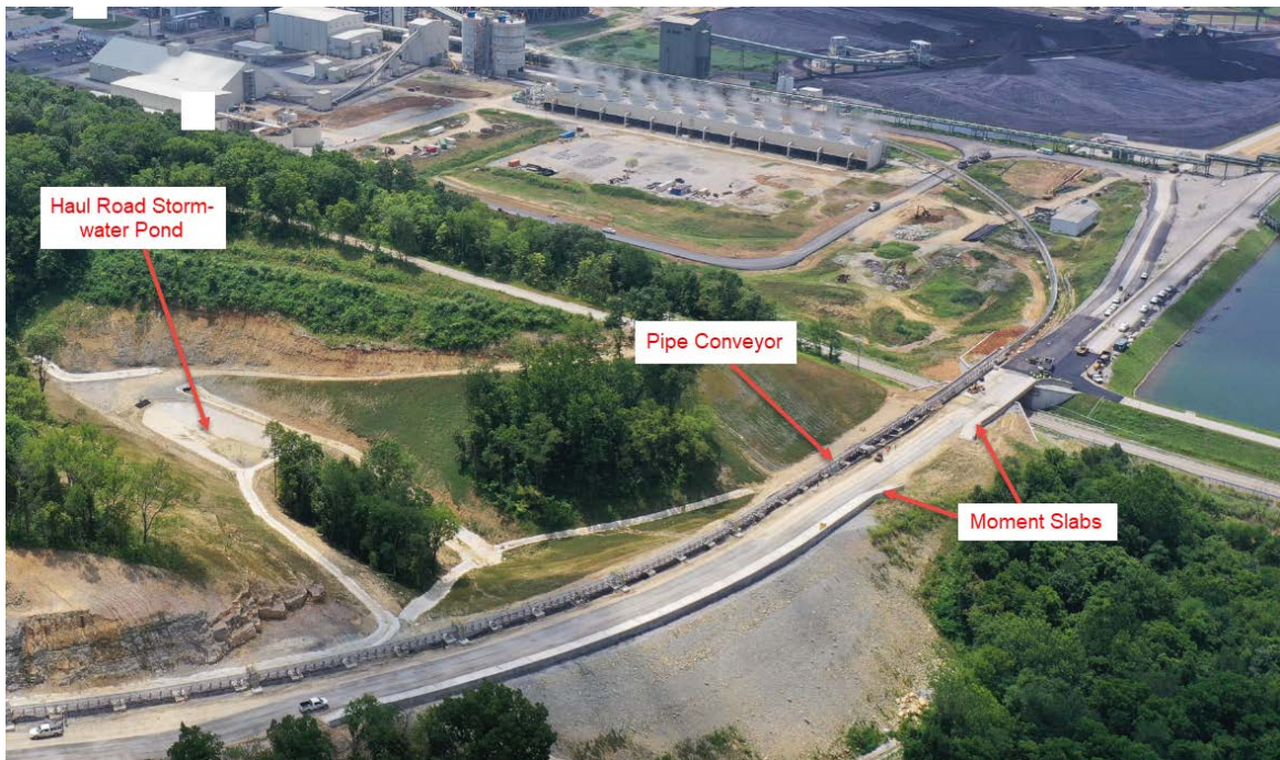
CCRT Transport Corridor – View of Bridge Over KY 1838 to Landfill (Looking West) – June 2019
