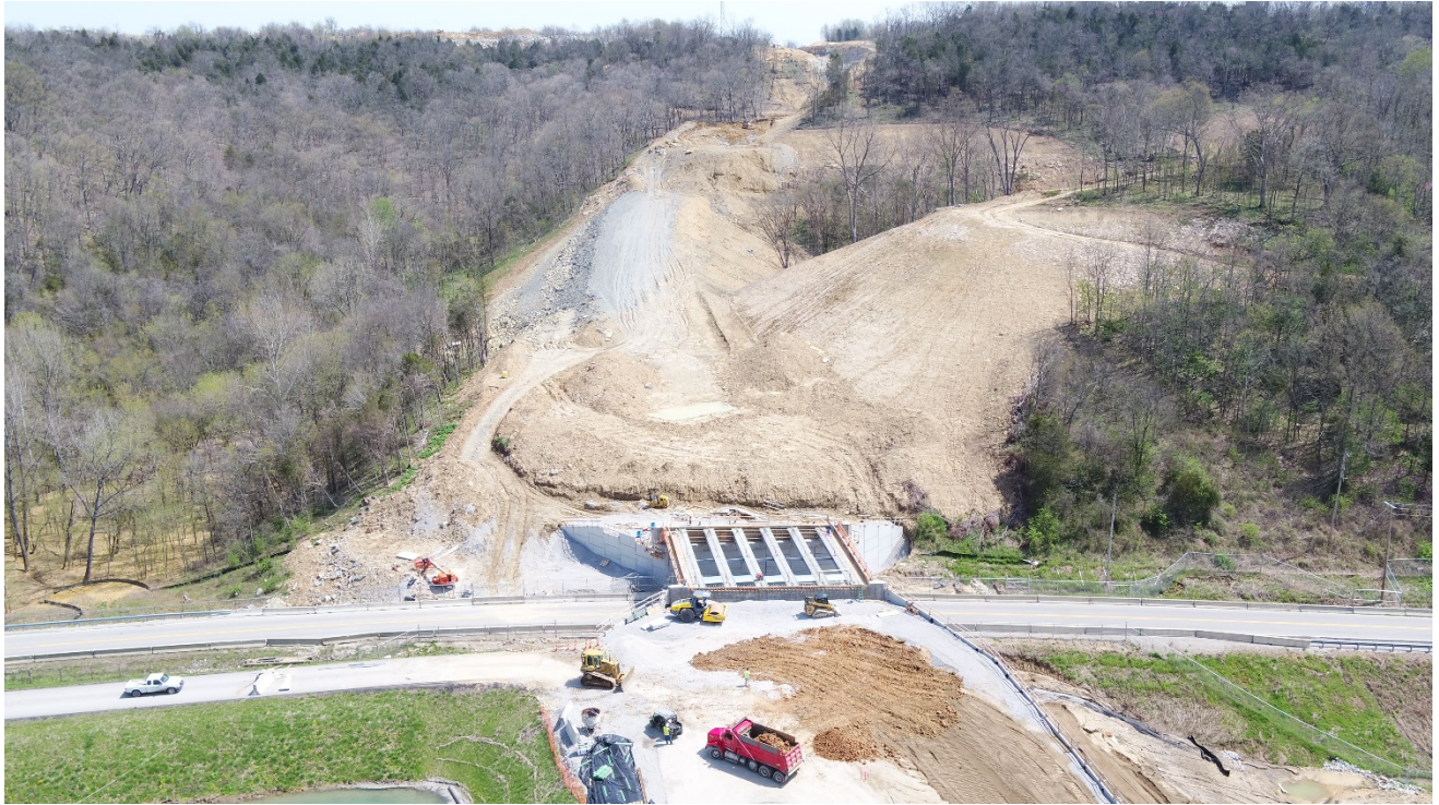
CCR Transport Corridor – View from Bridge over KY 1838 to Landfill (Looking East) – Photo from the April 2018 Report
