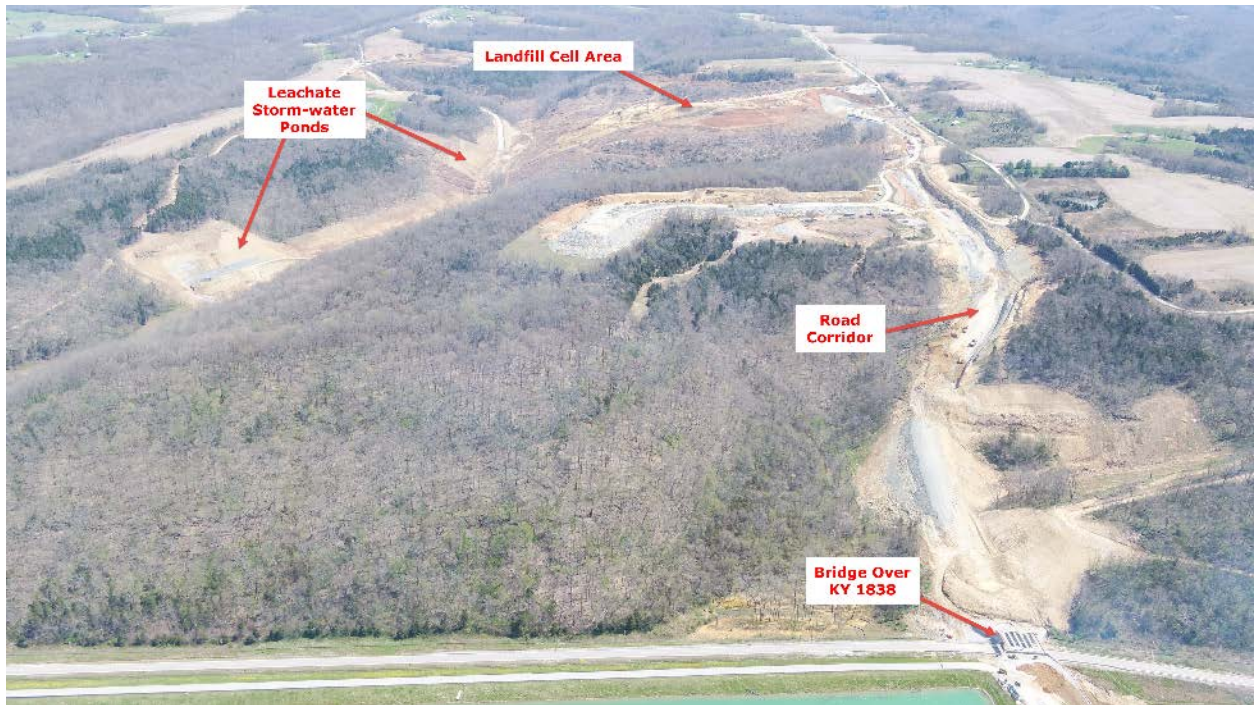
CCR Landfill Overview – View from Station (Looking East) – Photo from the April 2018 Report
