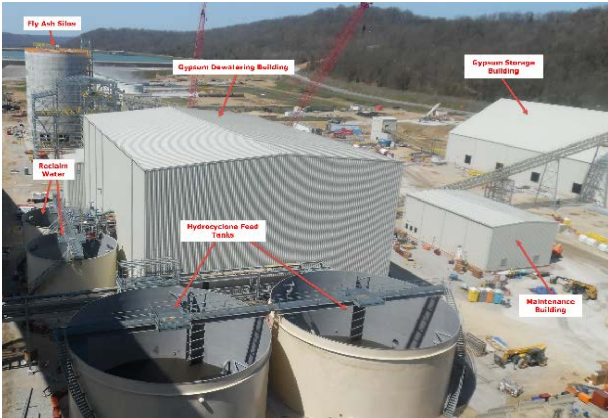
CCRT Project Area Looking North – Photo from the April 2018 Report
