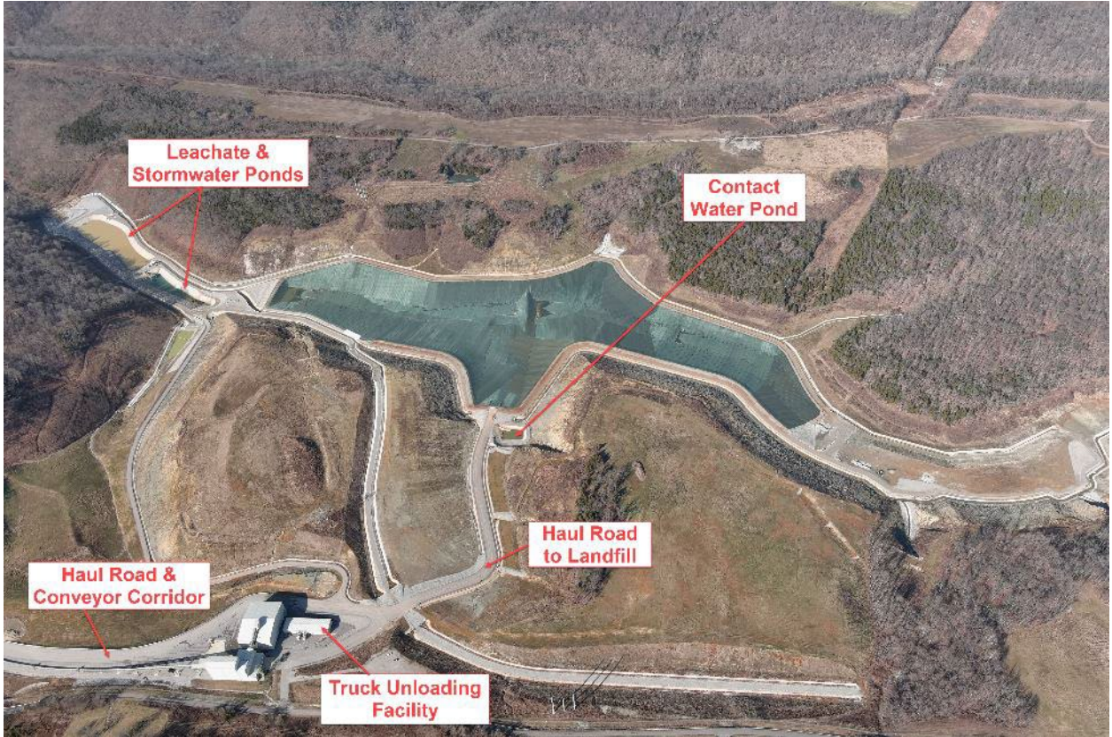
CCR Landfill Overview – View Looking North – December 2022
