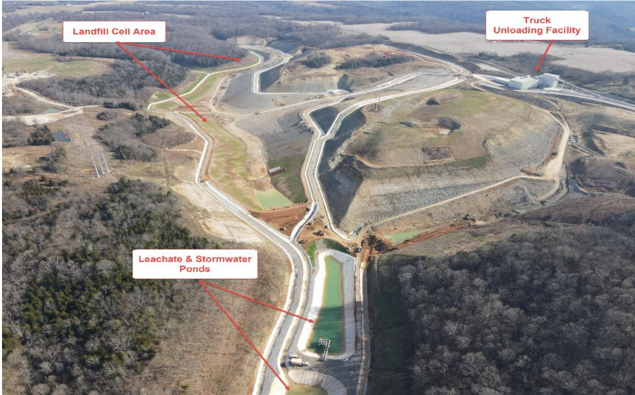
CCR Landfill Overview – View Looking East – December 2020
