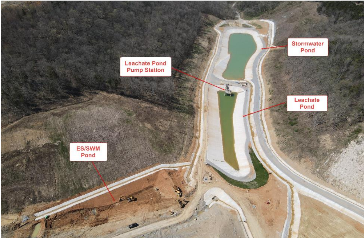
CCR Landfill Overview – View of leachate and stormwater ponds (Looking West) – March 2021
