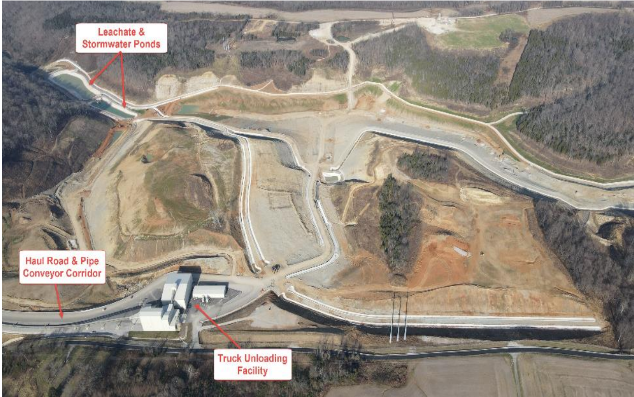
CCR Landfill Overview – View Looking North – December 2020
