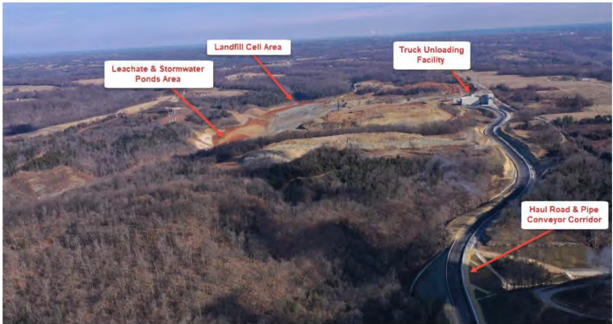
CCR Landfill Overview – View from Station (Looking East) – December 2019
