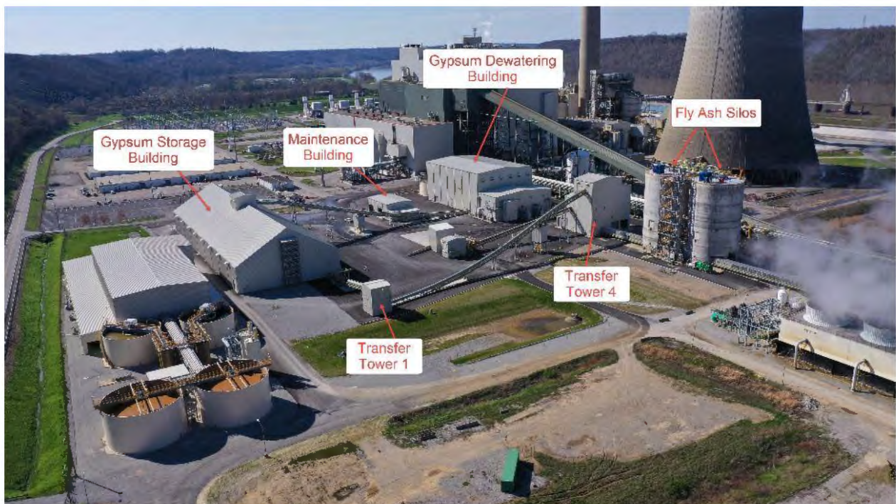
CCRT Project Area Looking South – March 2020
