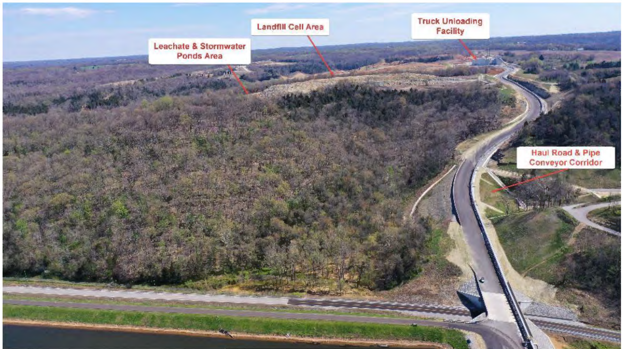
CCR Landfill Overview – View from Station (Looking East) – March 2020
