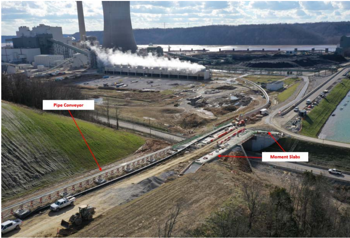
CCRT Transport Corridor – View of Bridge Over KY 1838 to Landfill (Looking West) –December 2018
