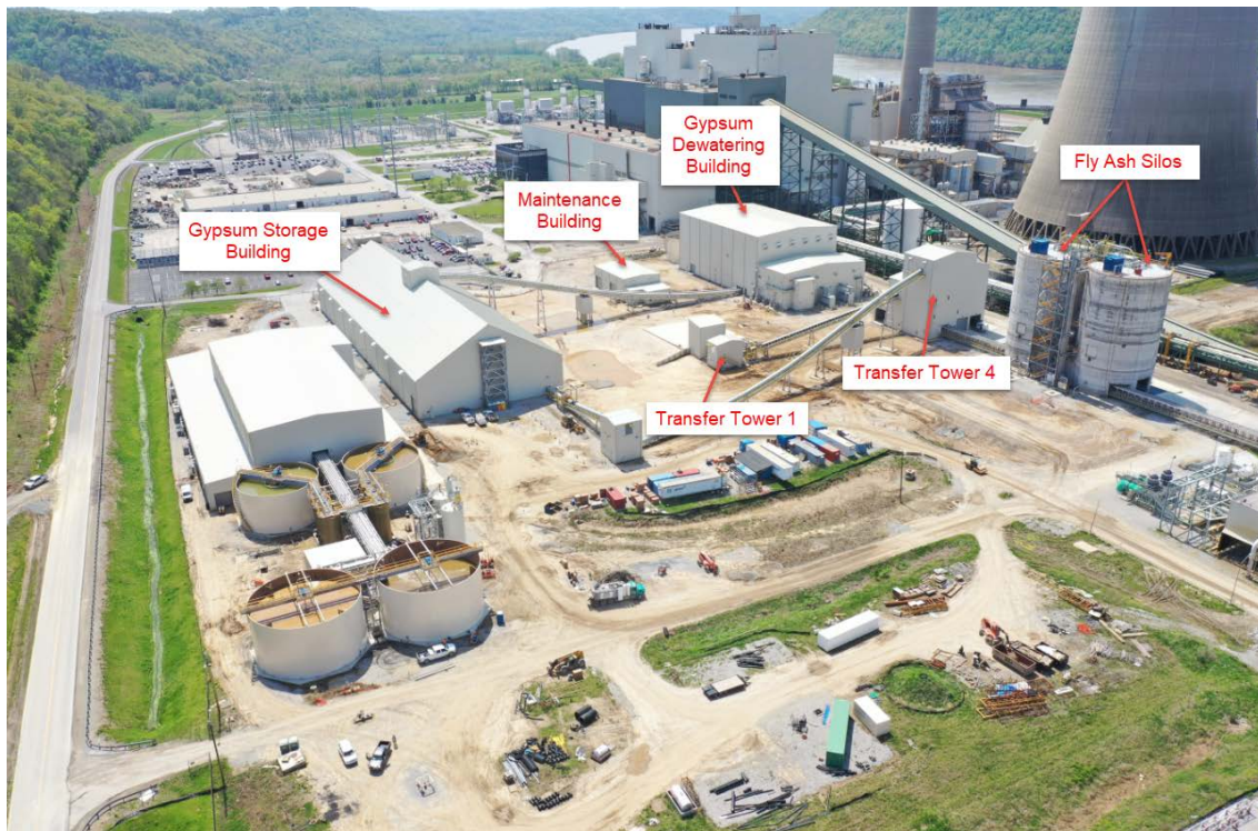
CCRT Project Area Looking South – April 2019
