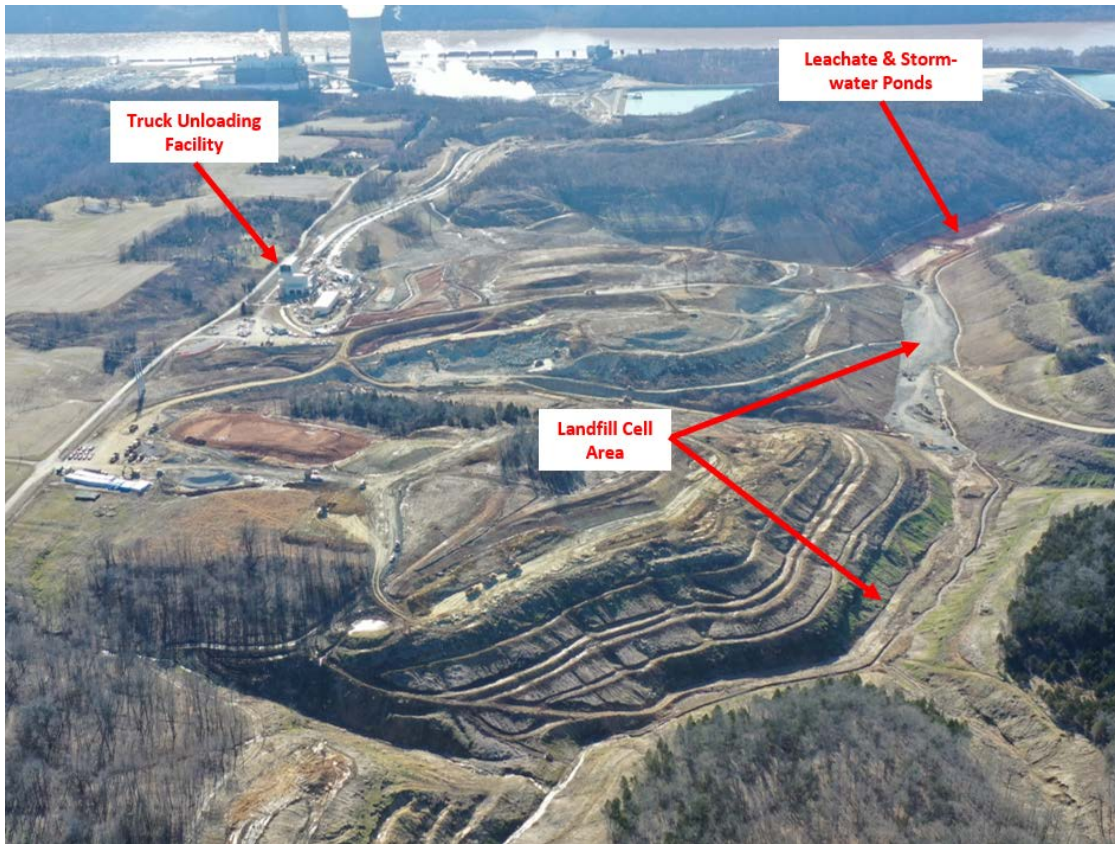
CCR Landfill Overview – View toward Station (Looking West) – March 2019
