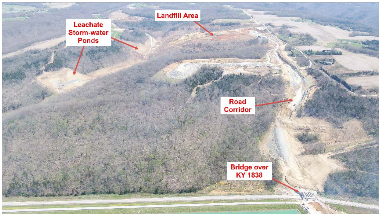
CCR Landfill Overview – View from Station (Looking East) – Current
