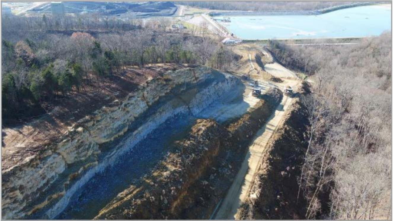
CCR Transport Corridor – View to Bridge over KY 1838 and Station (Looking West) – Photo from the January 2018 Report
