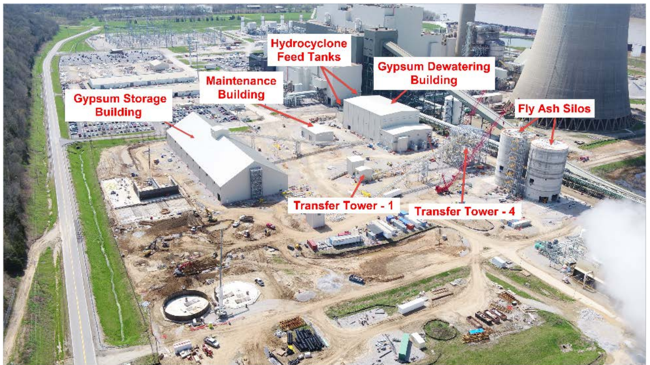
CCRT Project Area Looking South – Current
