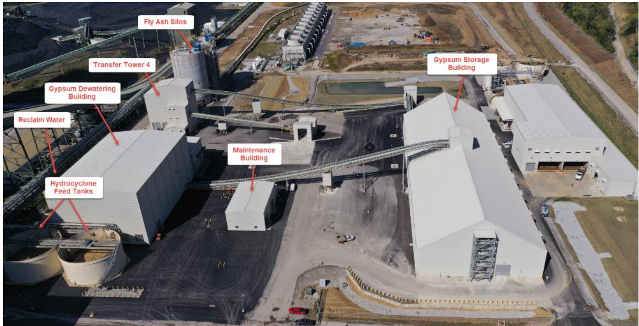
CCRT Project Area Looking North – October 2019
