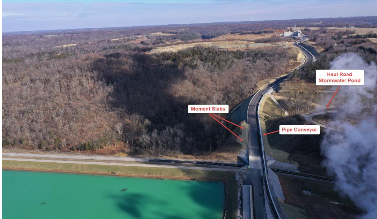
CCRT Transport Corridor – View of Bridge Over KY 1838 to Landfill (Looking East) – December 2019
