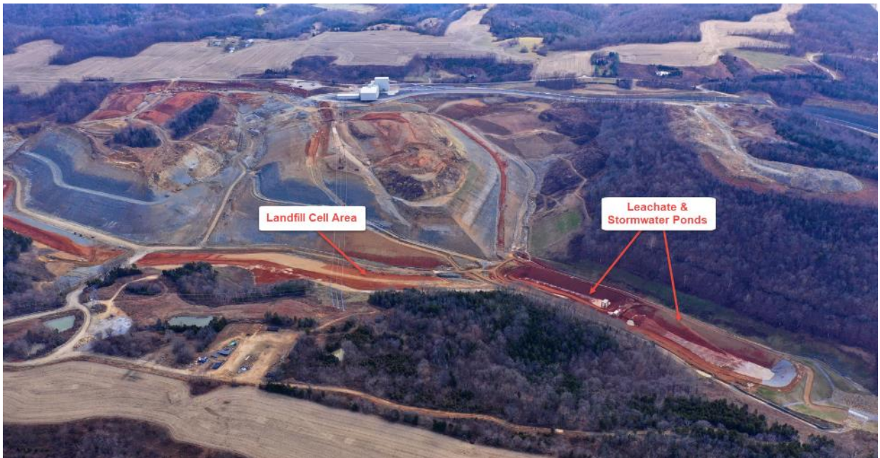
CCR Landfill Overview – View toward Station (Looking South West) – December 2019
