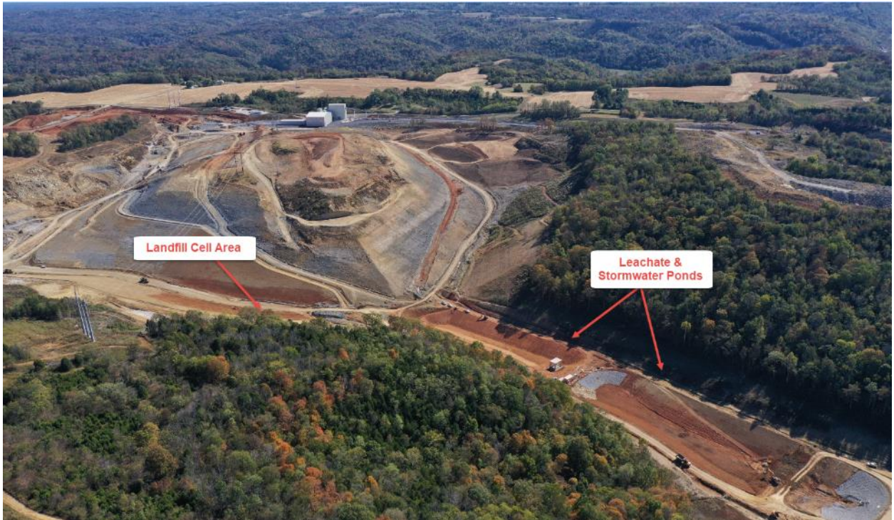
CCR Landfill Overview – View toward Station (Looking South West) – October 2019
