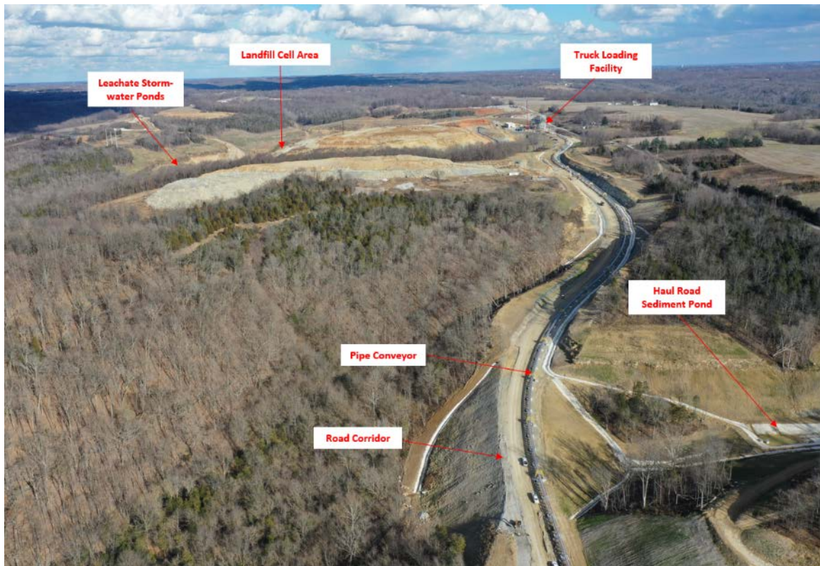
CCR Landfill Overview – View from Station (Looking East) –December 2018
