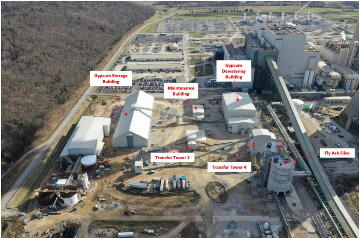
CCRT Project Area Looking South – December 2018
