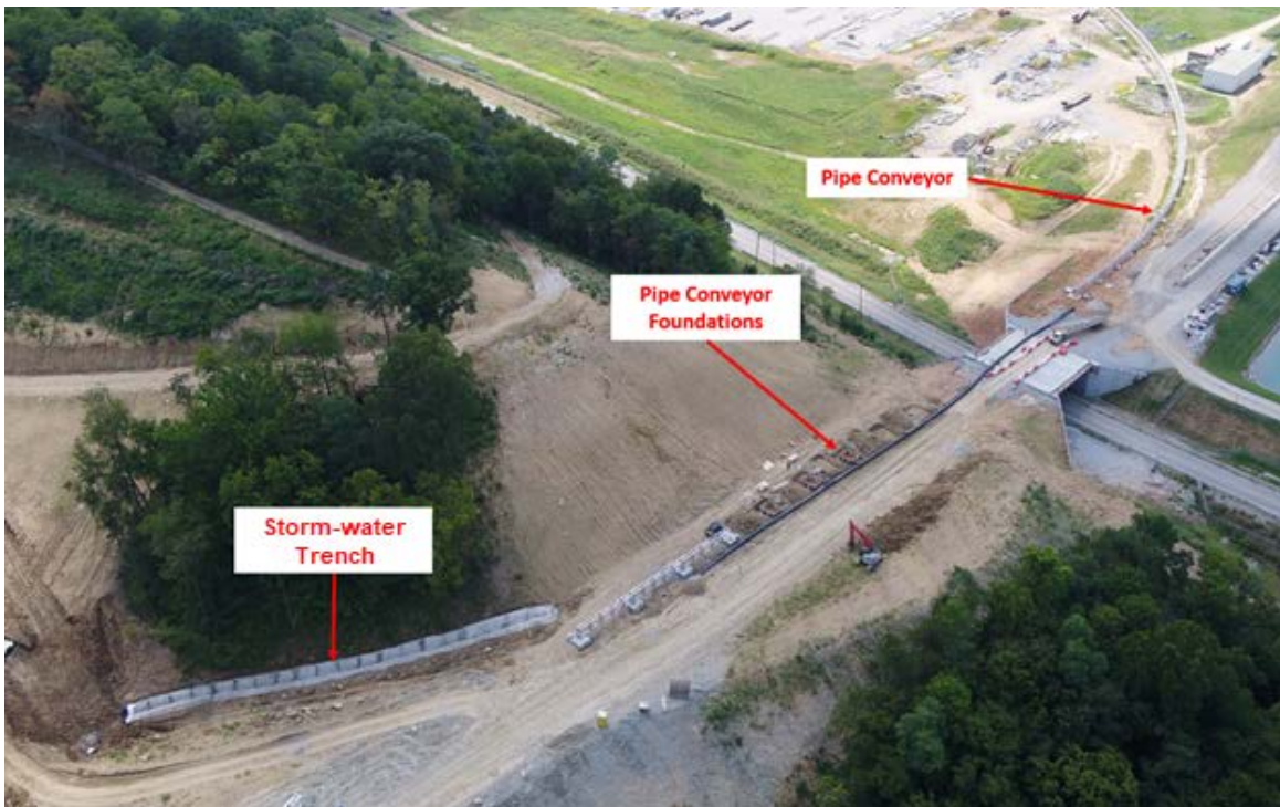
CCRT Transport Corridor – View of Bridge Over KY 1838 to Landfill (Looking West) – August 2018
