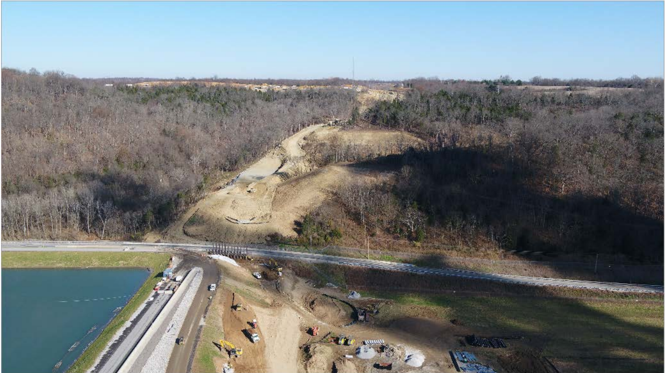
CCR Transport Corridor – View to Landfill from Station (Looking East) – Current
