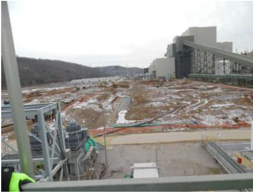
CCRT Project Area Looking South
