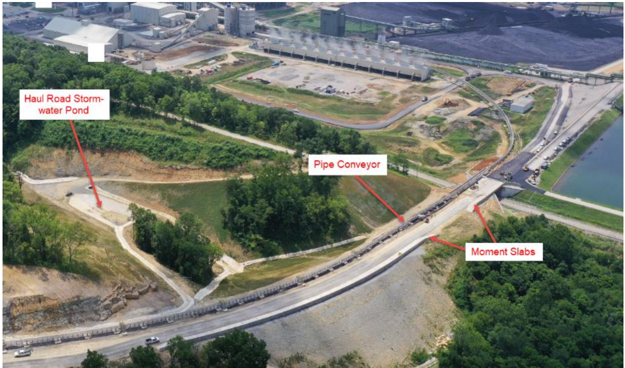
CCRT Transport Corridor – View of Bridge Over KY 1838 to Landfill (Looking West) – June 2019
