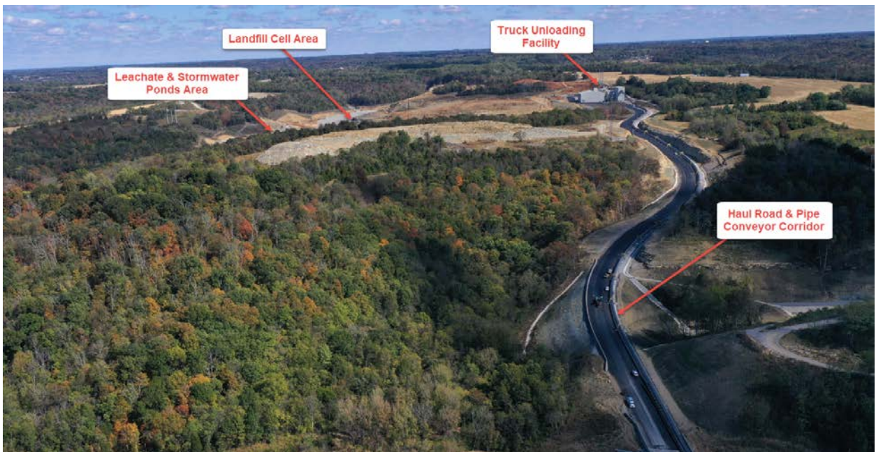
CCR Landfill Overview – View from Station (Looking East) – October 2019
