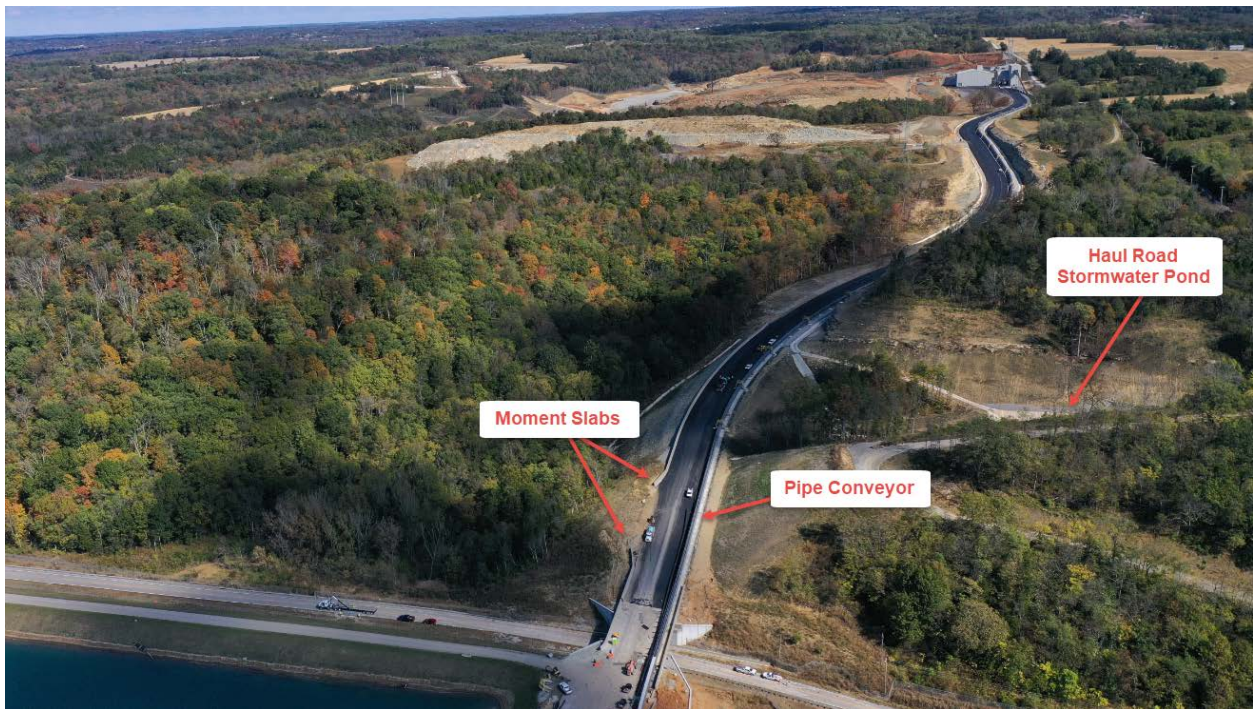
CCRT Transport Corridor – View of Bridge Over KY 1838 to Landfill (Looking East) – October 2019
