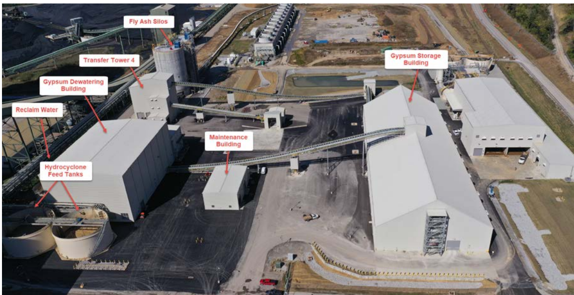
CCRT Project Area Looking North – October 2019
