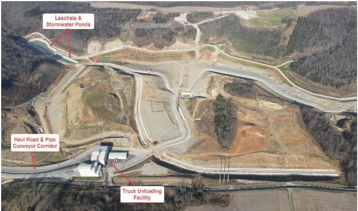
CCR Landfill Overview – View Looking Toward Station (Looking North) – December 2020
