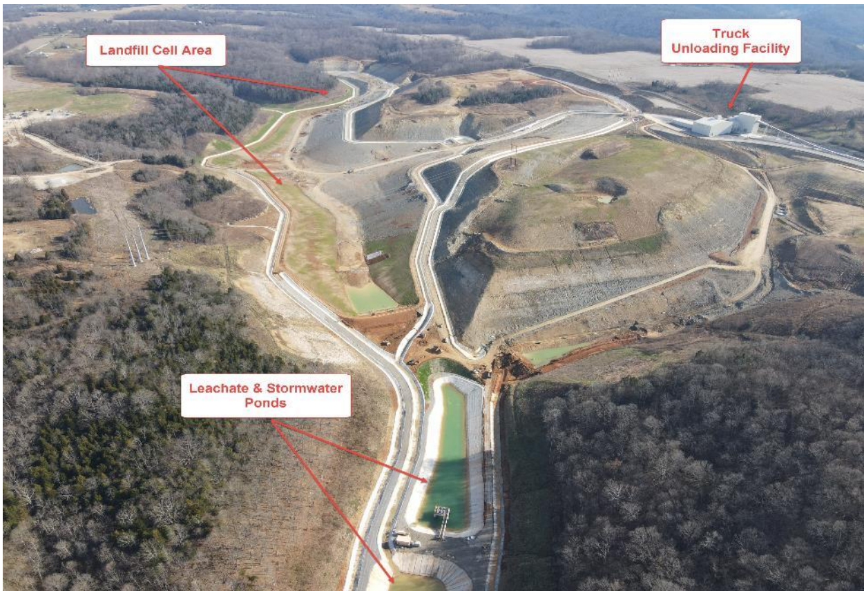
CCR Landfill Overview – View Looking East – December 2020
