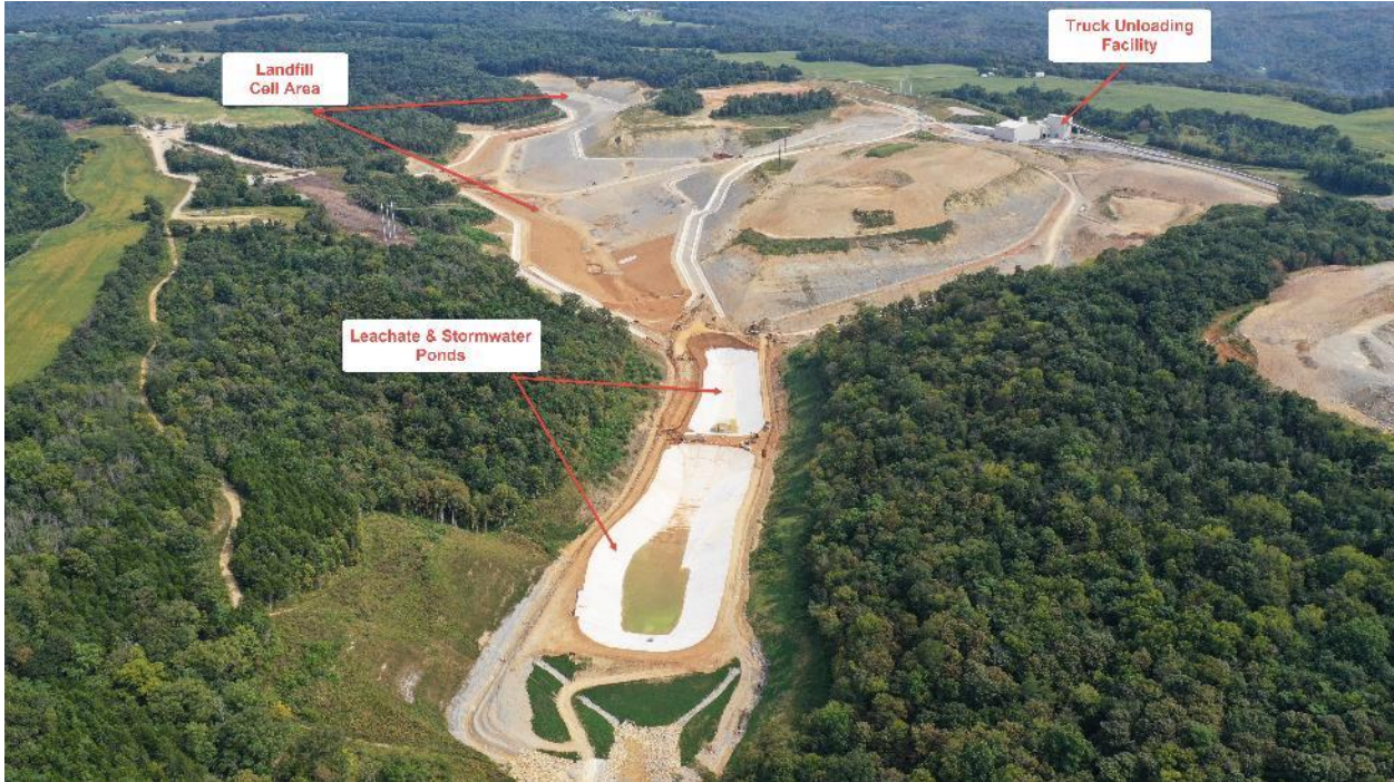
CCR Landfill Overview – View Looking East – September 2020
